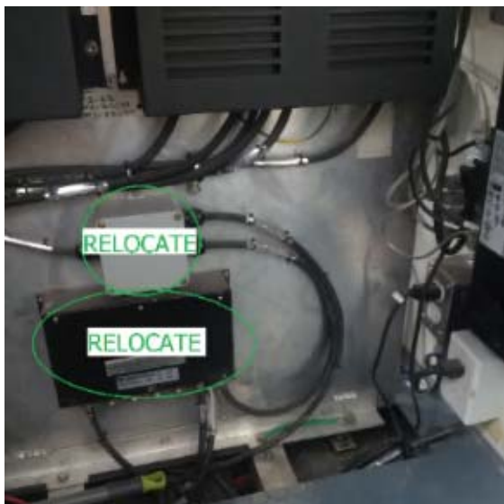
Photo #26 – JB AIS-01 & RZ255 Unit (To be Relocated)
