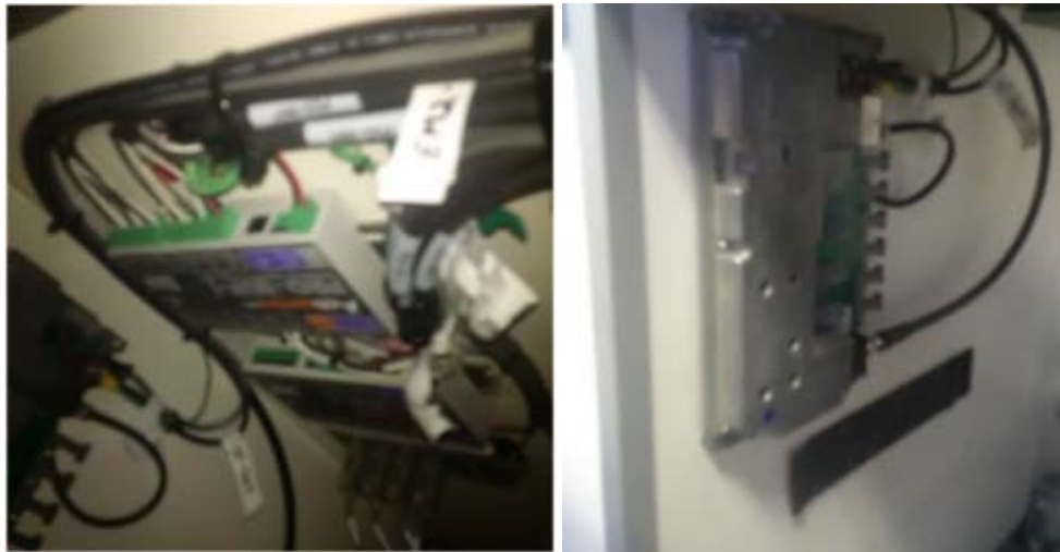
Photo #31 & #32 – Example Install of New PRO-BUF-1 & Navtex Units
