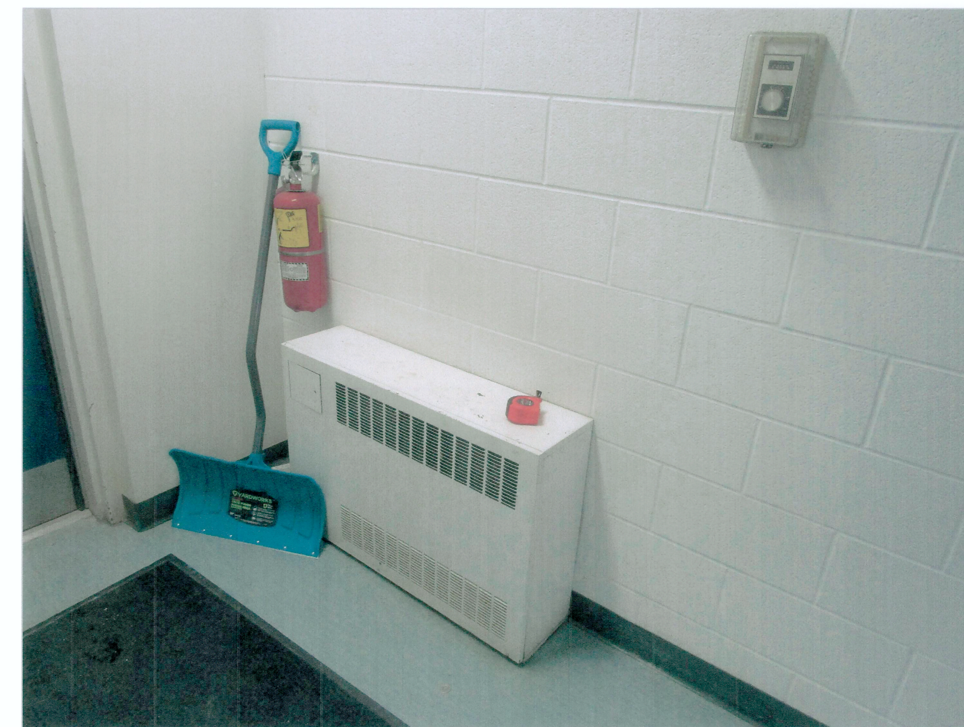
7 TYPICAL EXISTING FORCE FLOW AND THERMOSTAT
