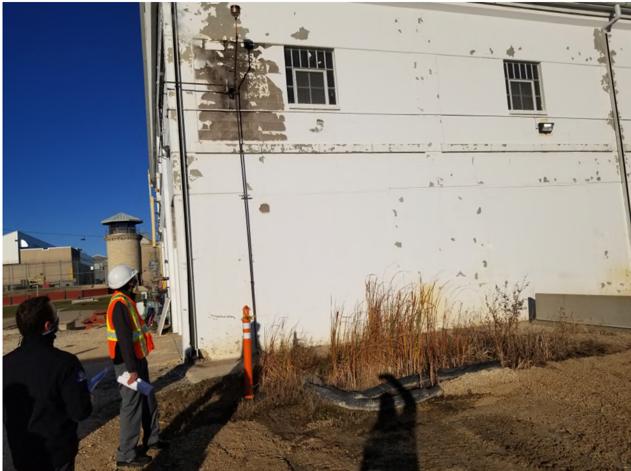
Picture 1 Showing Building Exterior, East
