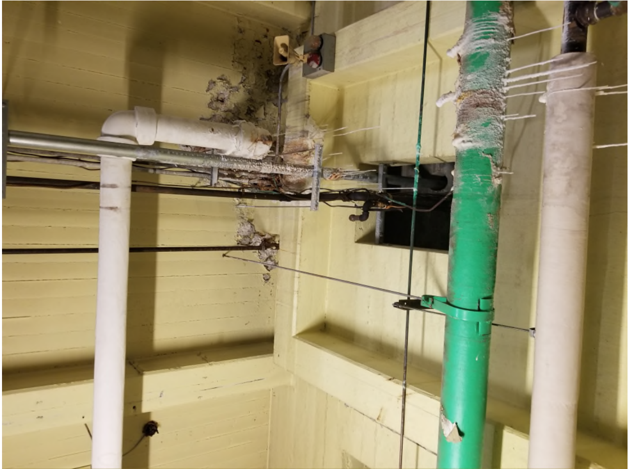
Picture 23 Showing sub basement walls
