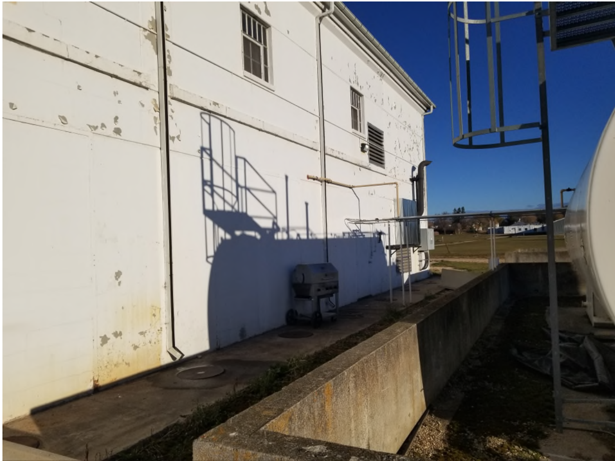
Picture 2 Showing Along Building Exterior, East
