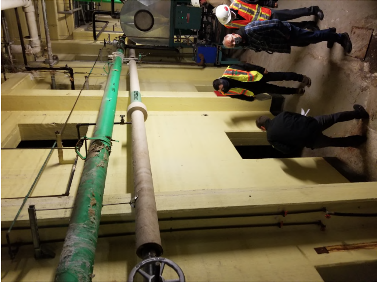
Picture 15 Showing sub basement wall
