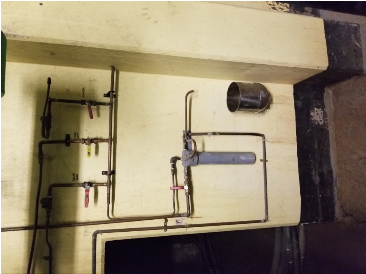
Picture 21 Showing sub basement walls
