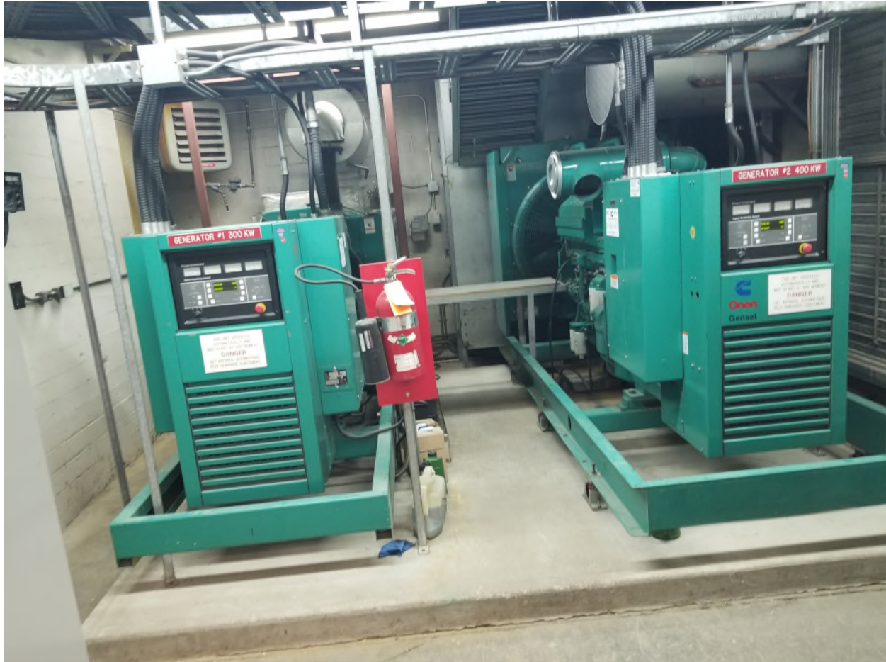
Picture 10 Showing Generator Room, above Coal Vaults
