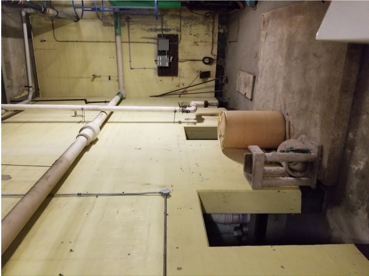
Picture 17 Showing sub basement walls
