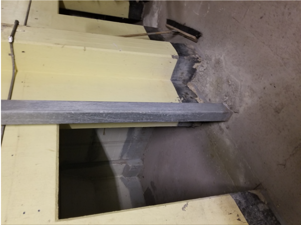
Picture 20 Showing sub basement walls
