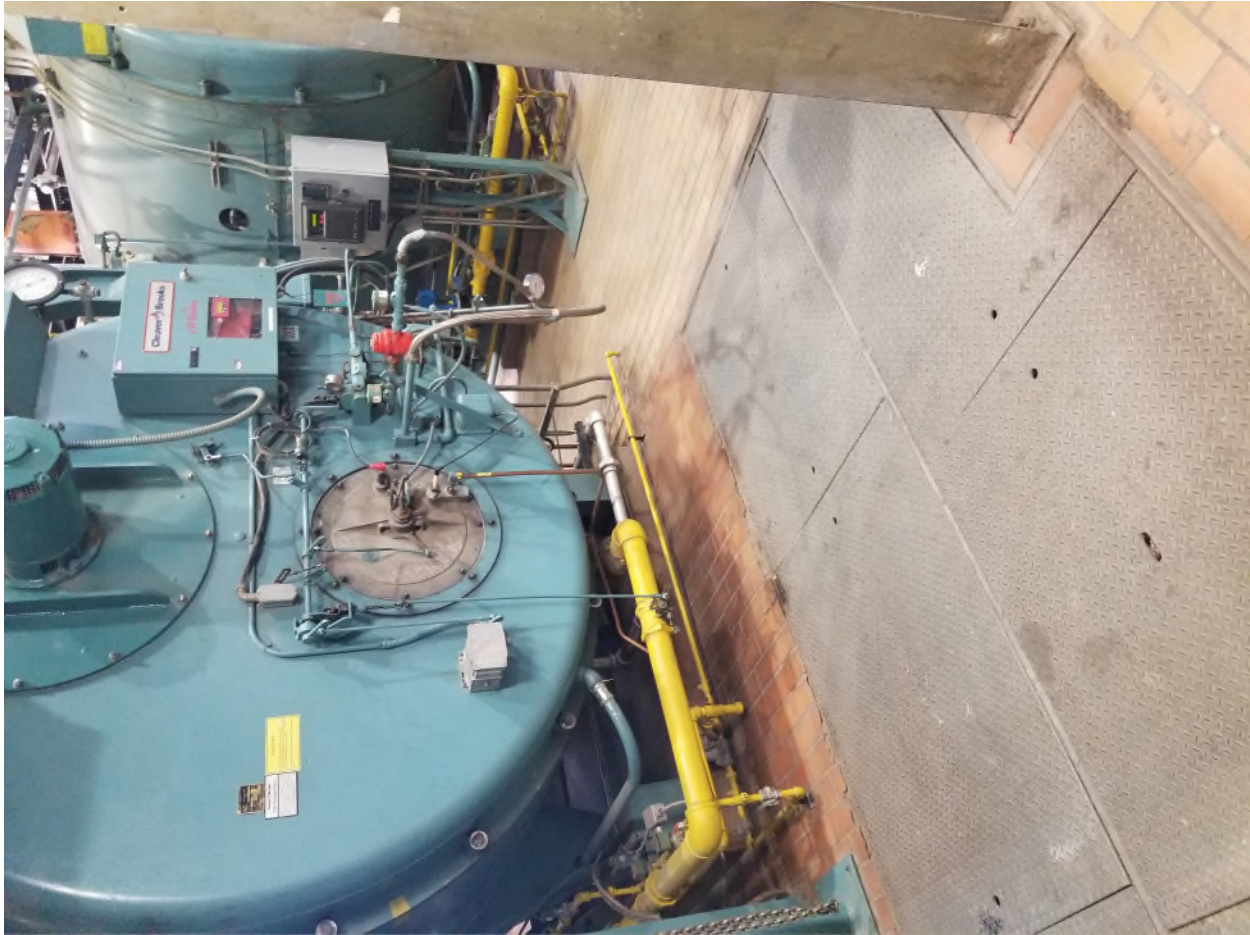
Picture 26 Showing main floor access panels above sub basement
