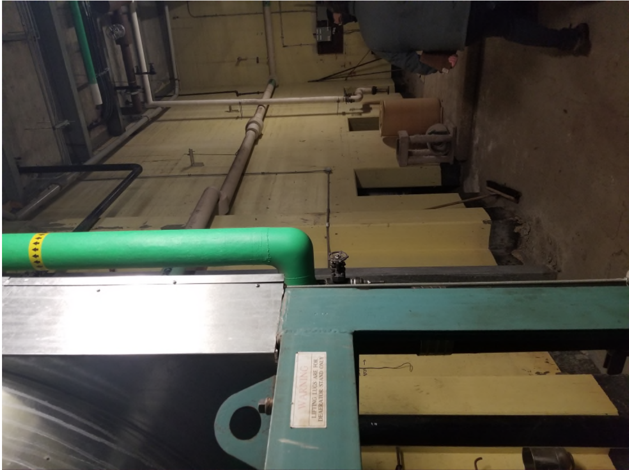
Picture 16 Showing sub basement walls
