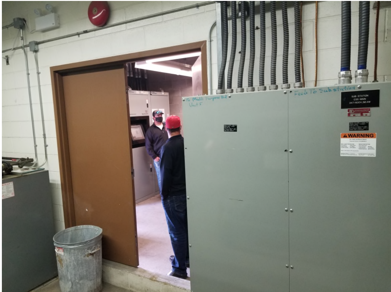
Picture 8 Showing Generator Room, above Coal Vaults
