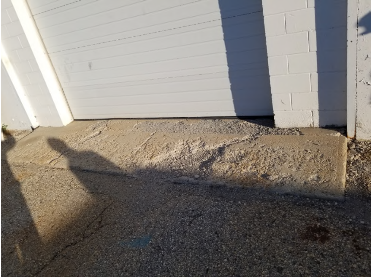
Picture 3 Showing Exterior Concrete Apron
