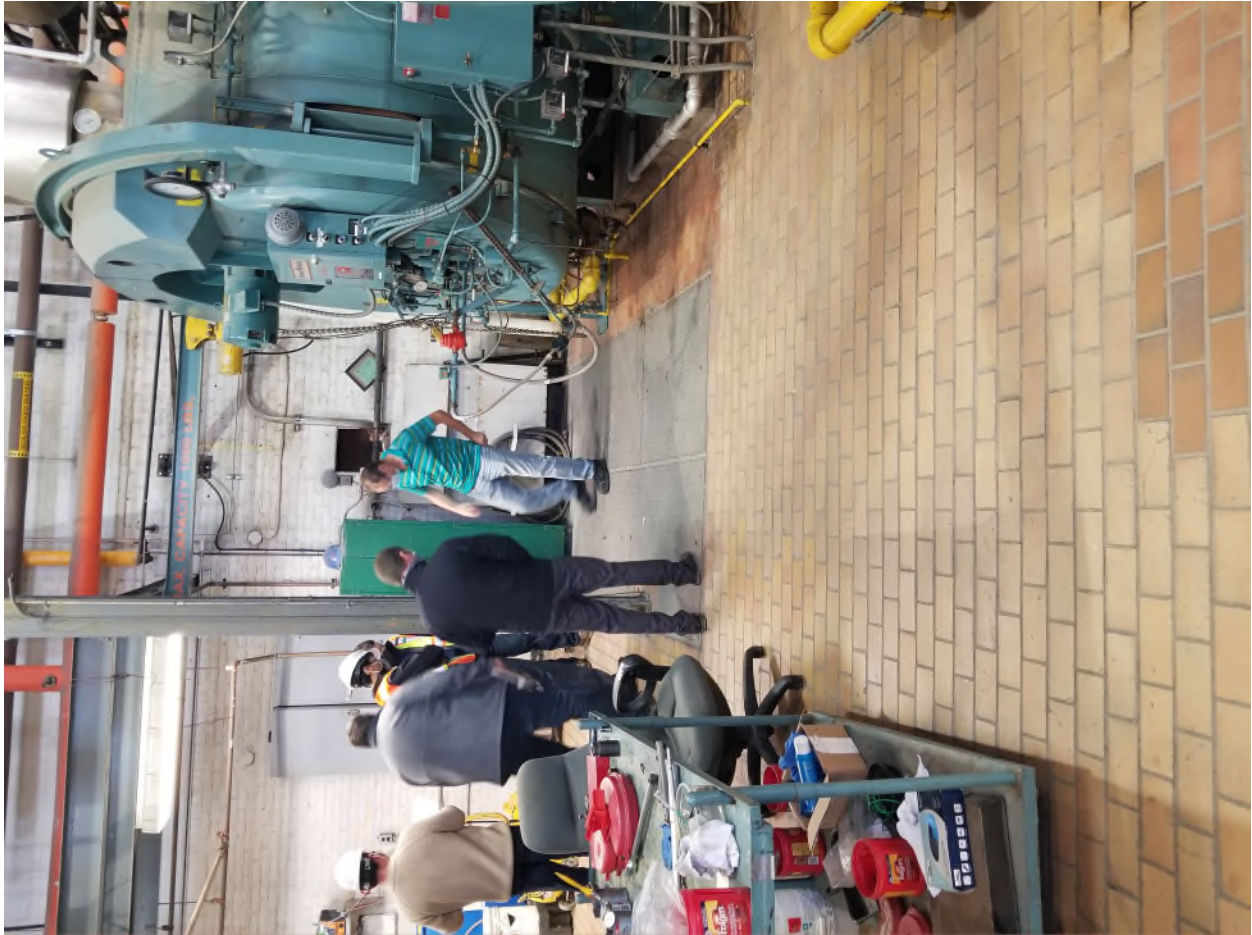
Picture 24 Showing main floor access panels above sub basement
