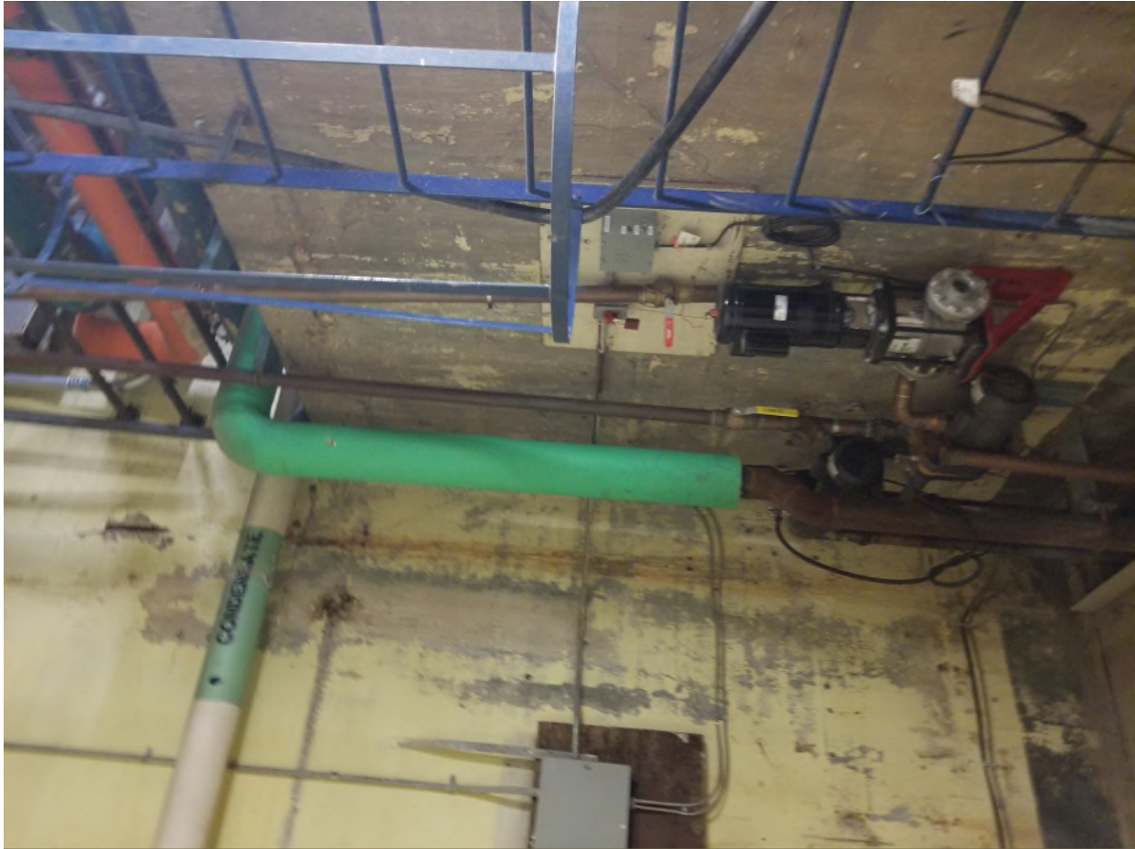
Picture 19 Showing sub basement walls
