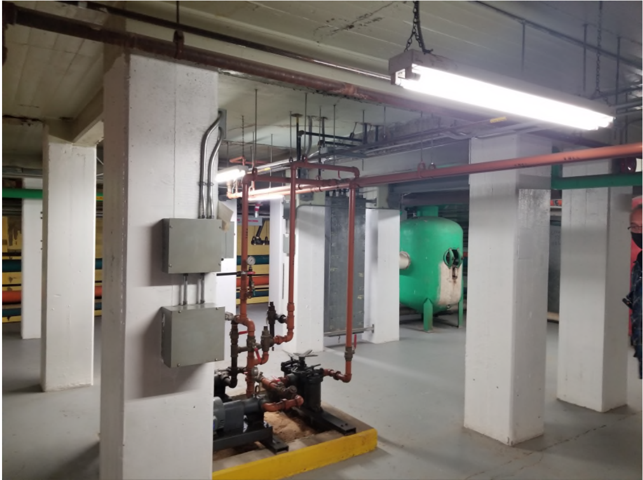
Picture 11 Showing Beam to be Repaired
