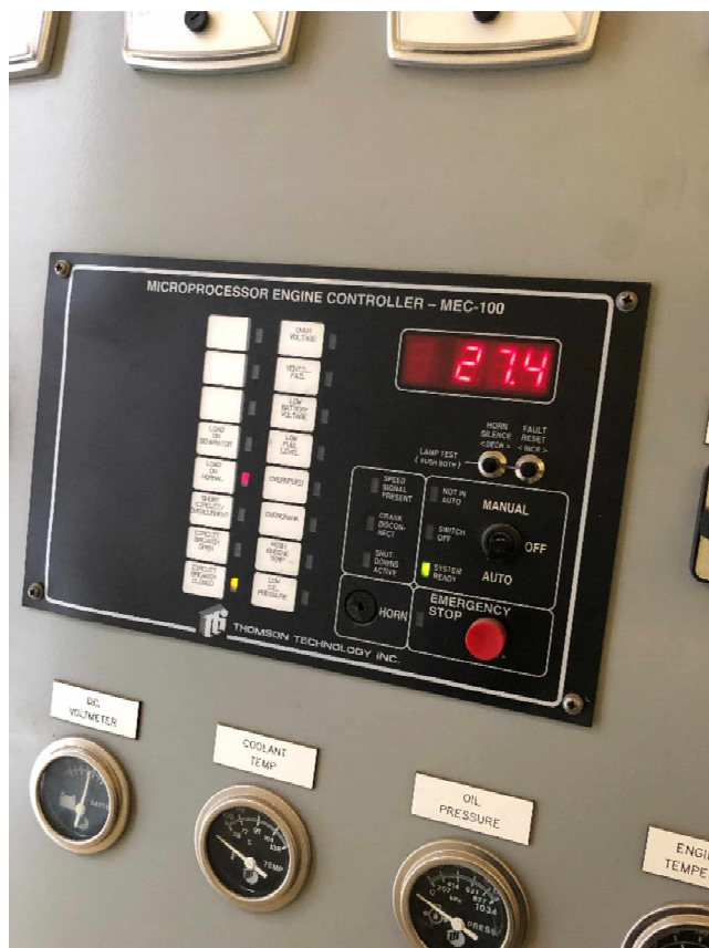
Photo #24- Existing controller // disconnect old fuel alarms and reconnect new alarms
