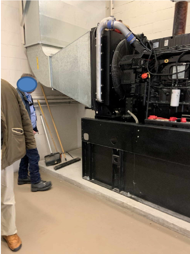
Photo #6 – location where condensate tank will be installed
