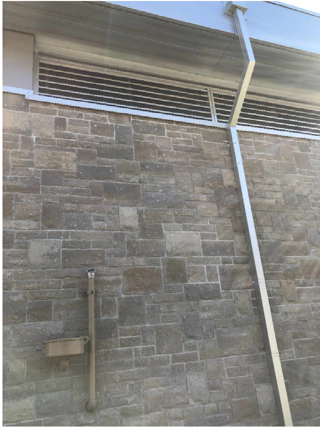
Photo #11– Location of new Lighting fixture
