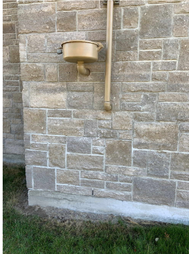
Photo #4 – showing area where service platform will be installed
