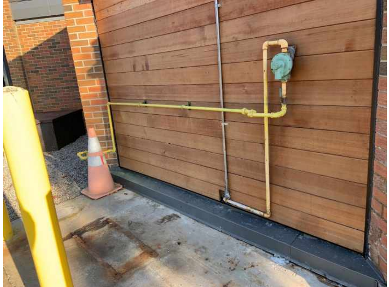
Photo #2 – Close up Photo of area of work
