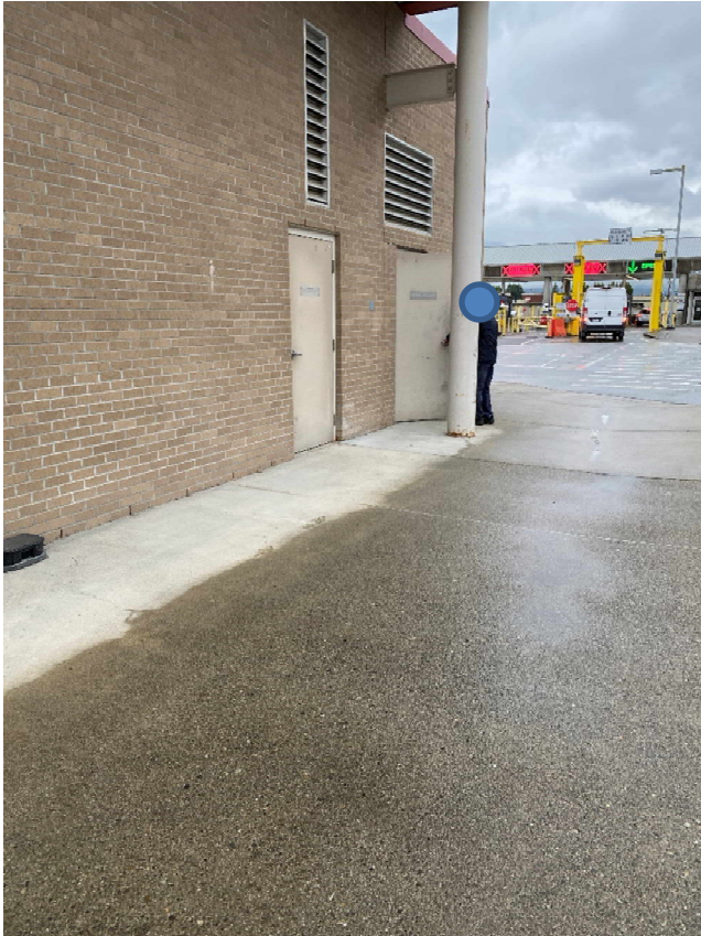
Photo #12 – Showing location of Generator and Electrical room
