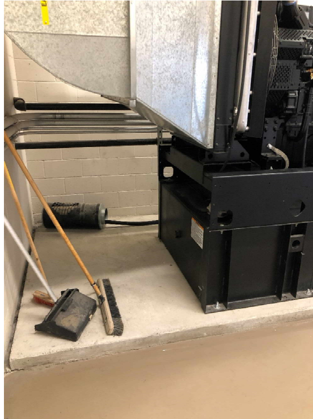
Photo #7 – location where condensate tank will be installed
