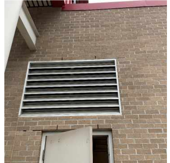
Photo #23 – Location of roof in relation to generator room
