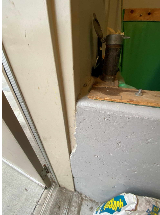
Photo #17 – Showing spill containment interface
