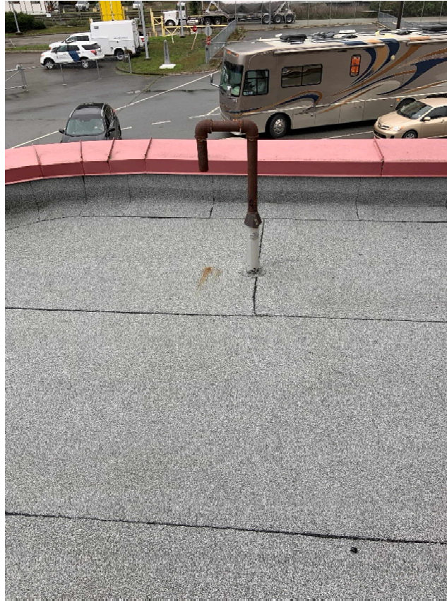
Photo #22– Showing top of roof vent line
