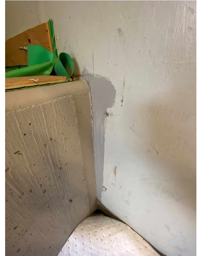
Photo #18 – Showing spill containment interface
