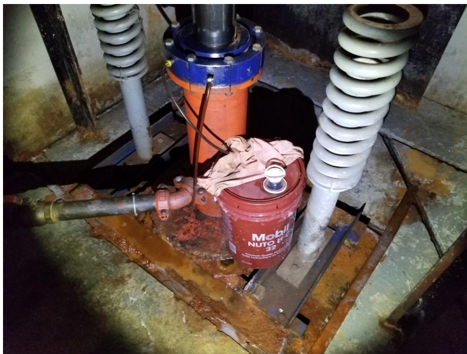
Photo 2: A oil container was observed inside the elevator pit. Grey floor paint in the pit contains less than 20 ppm lead.
