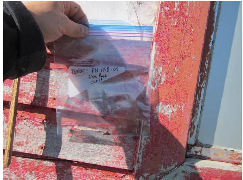
Photo 18: View of location of caulking sample FH-ASB-05 (exterior window frame).
