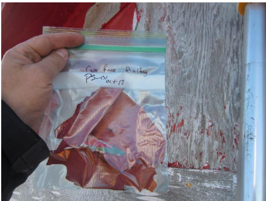
Photo 33: View of location of paint sample PS-01 on exterior wall.
