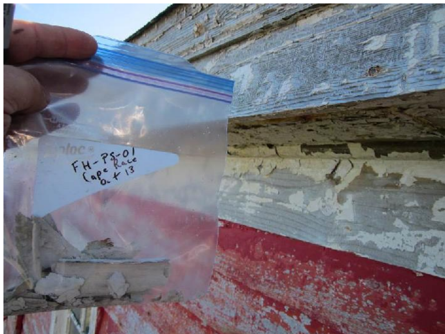
Photo 23: View of location of paint sample FH-PS-01 (exterior wall).
