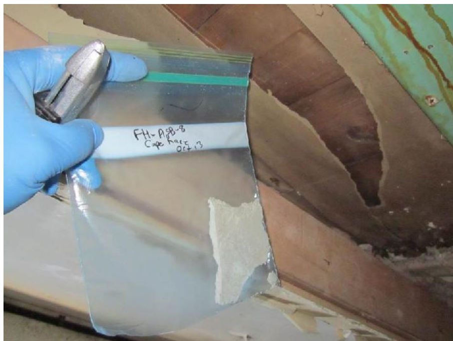
Photo 21: View of location of gyprock sample FH-ASB-08 (wall).
