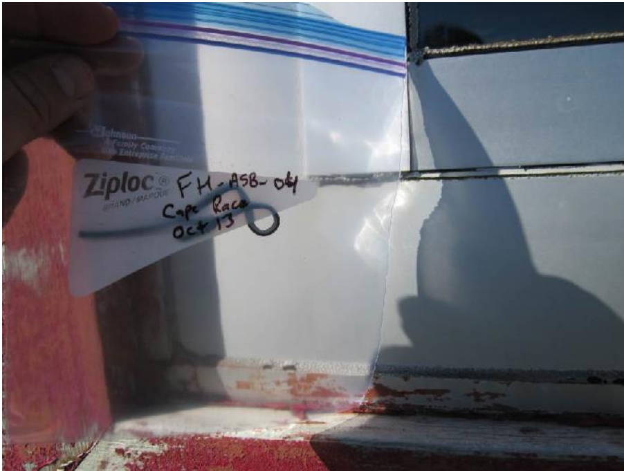
Photo 17: View of location of caulking sample FH-ASB-04 (exterior window frame).
