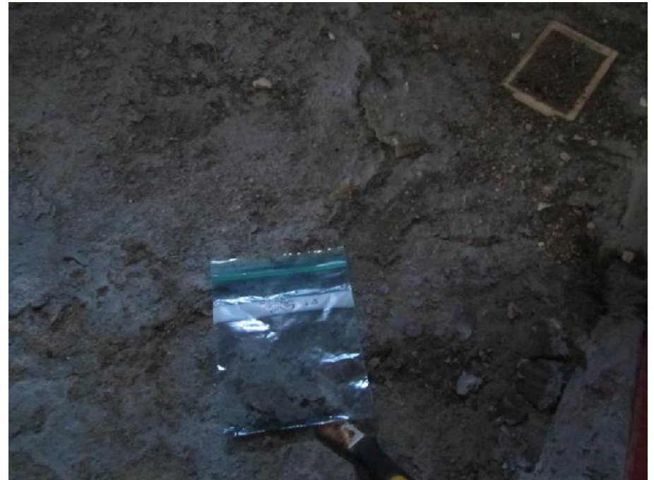
Photo 40: View of location of paint sample PS-08 in Room 11 (floor).
