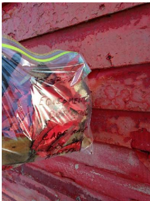
Photo 23: View of location of paint samples PS-2-A (exterior wall).
