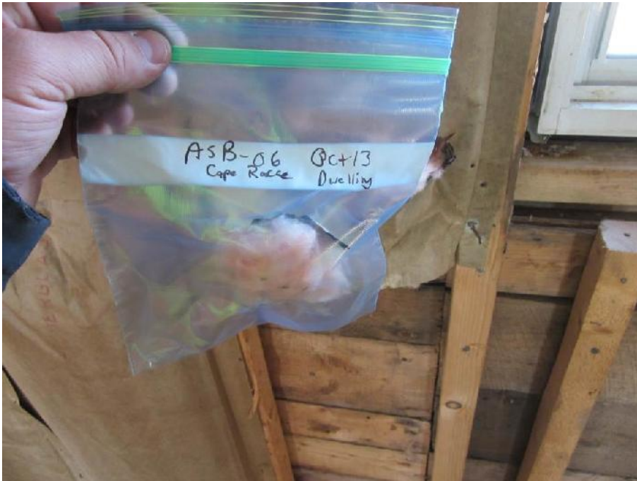
Photo 25: View of location of fiberglass insulation/paper backing sample ASB-06 (Room 3).
