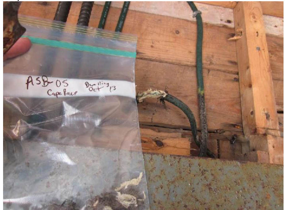
Photo 24: View of location of wire casing sample ASB-05 (Room 1).
