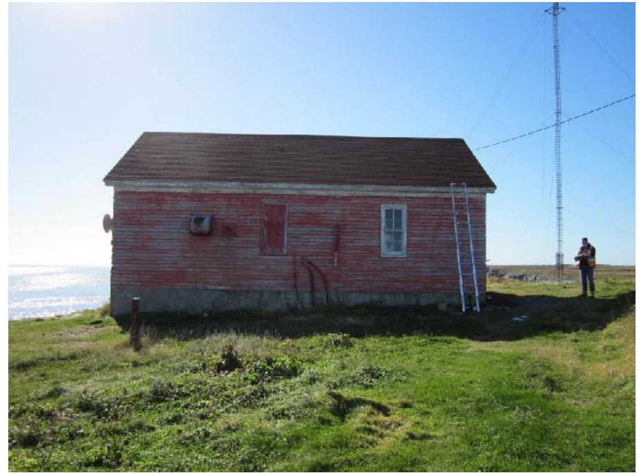
Photo 2: View of the northeast side of the Former Fog Horn Building.
