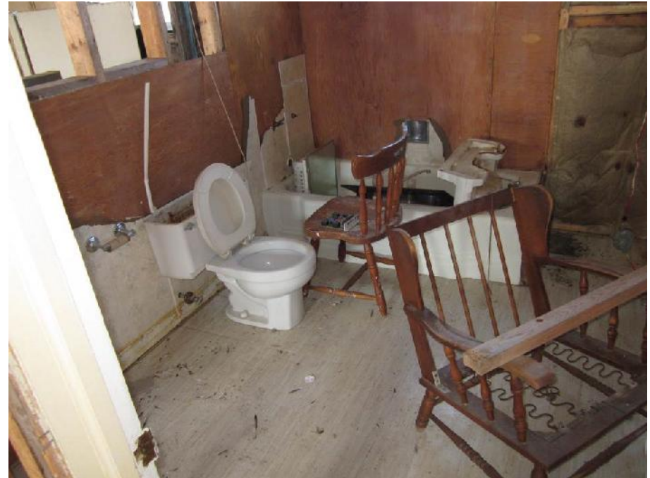
Photo 12: View of the bathroom (Room 4) in the Former Dwelling.
