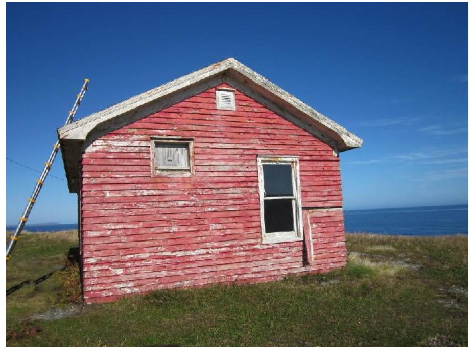
Photo 2: View of the southwest side of the Former Generator Building.
