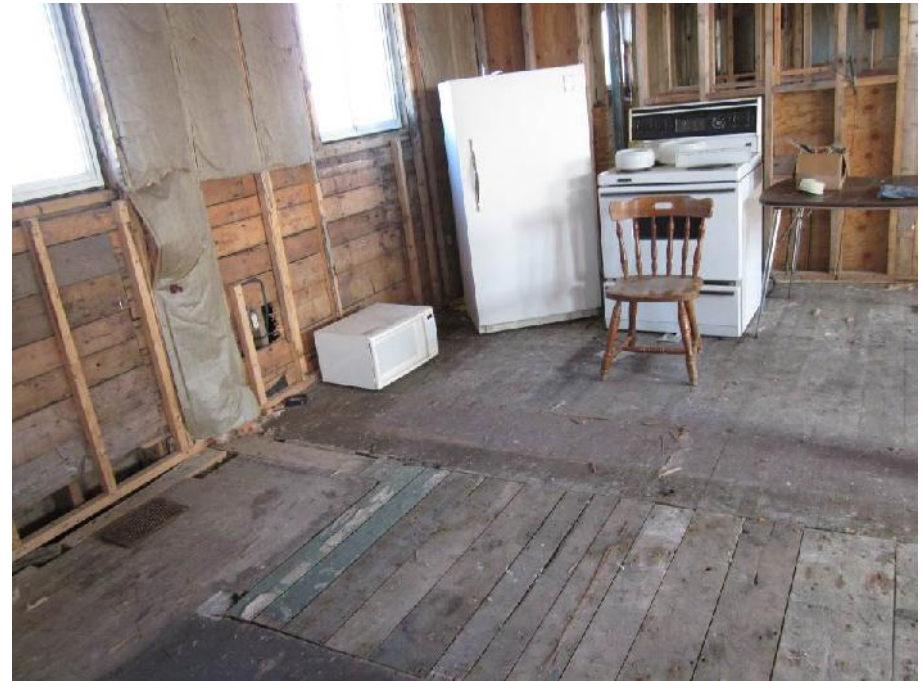
Photo 10: View of the dining room (Room 3) in the Former Dwelling. Note insulation in the wall on the left.
