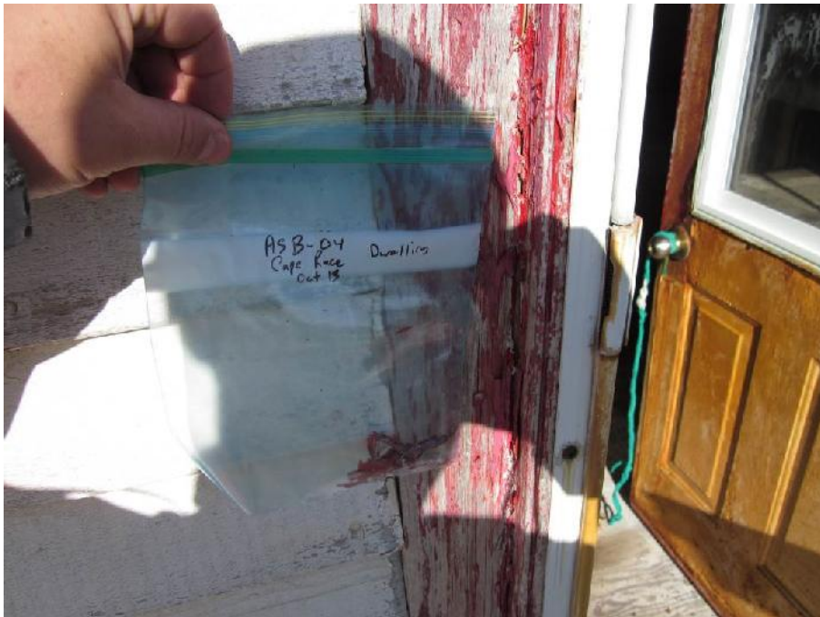
Photo 23: View of location of caulking sample ASB-04 (exterior door frame).
