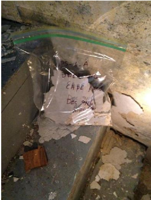
Photo 47: View of location of paint sample PS-6-A in Room 11 (foundation wall).
