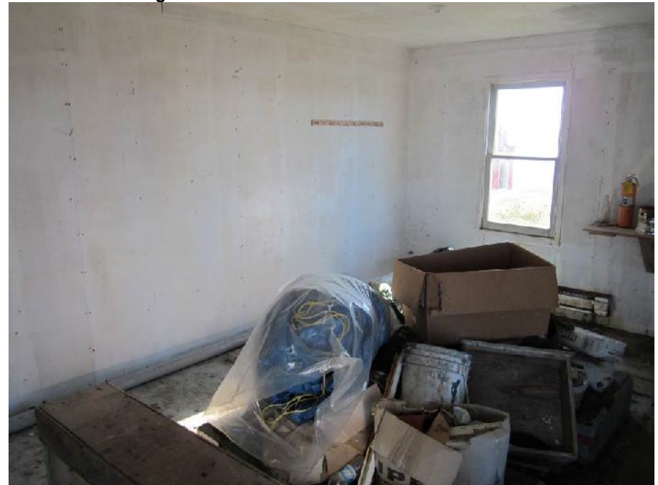
Photo 8: View of Room 1 in the Former Generator Building.
