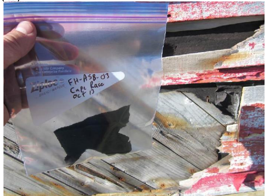
Photo 16: View of location of tar paper sample FH-ASB-03 (exterior wall).
