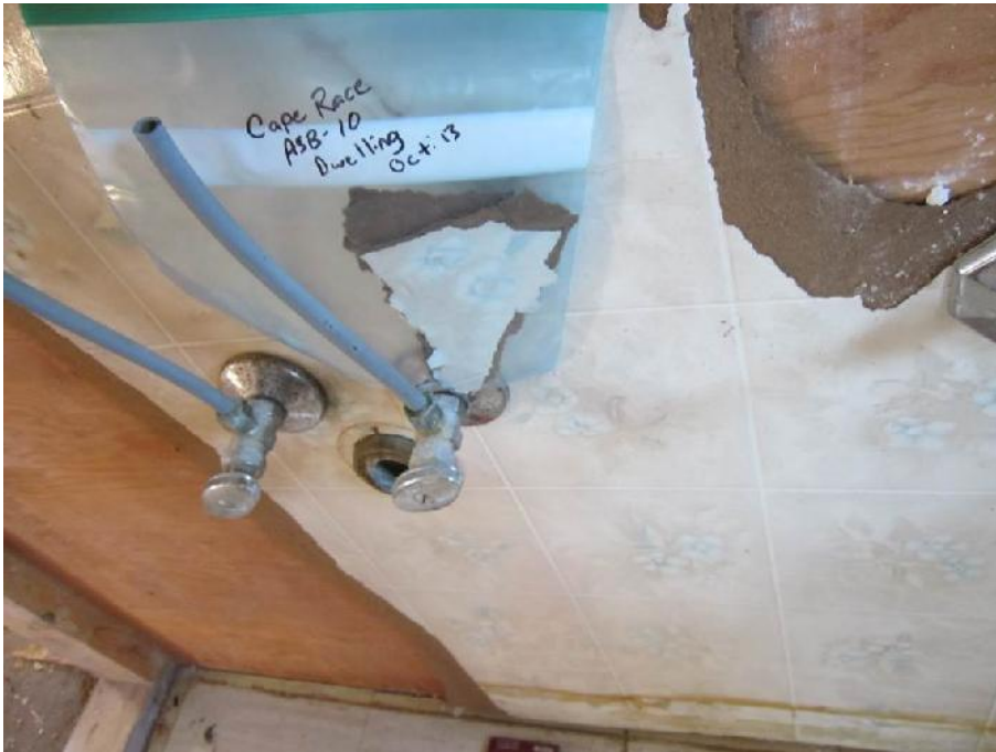
Photo 29: View of location of panel board sample ASB-10 (Room 4).
