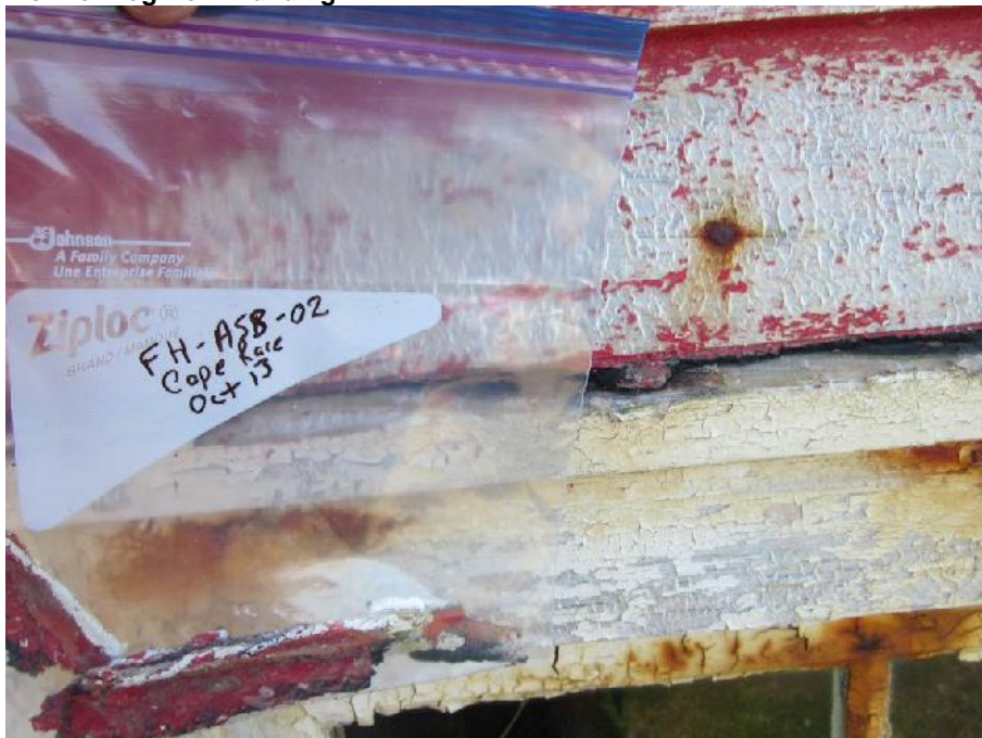
Photo 15: View of location of caulking and felt sample FH-ASB-02 (exterior wall).
