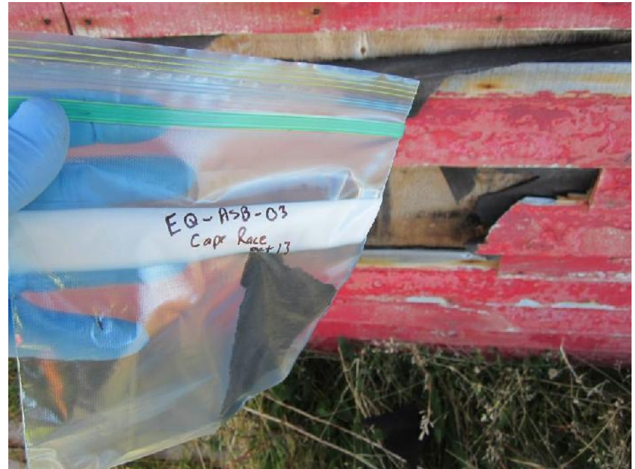
Photo 18: View of location of tar paper sample EQ-ASB-03 (exterior wall).
