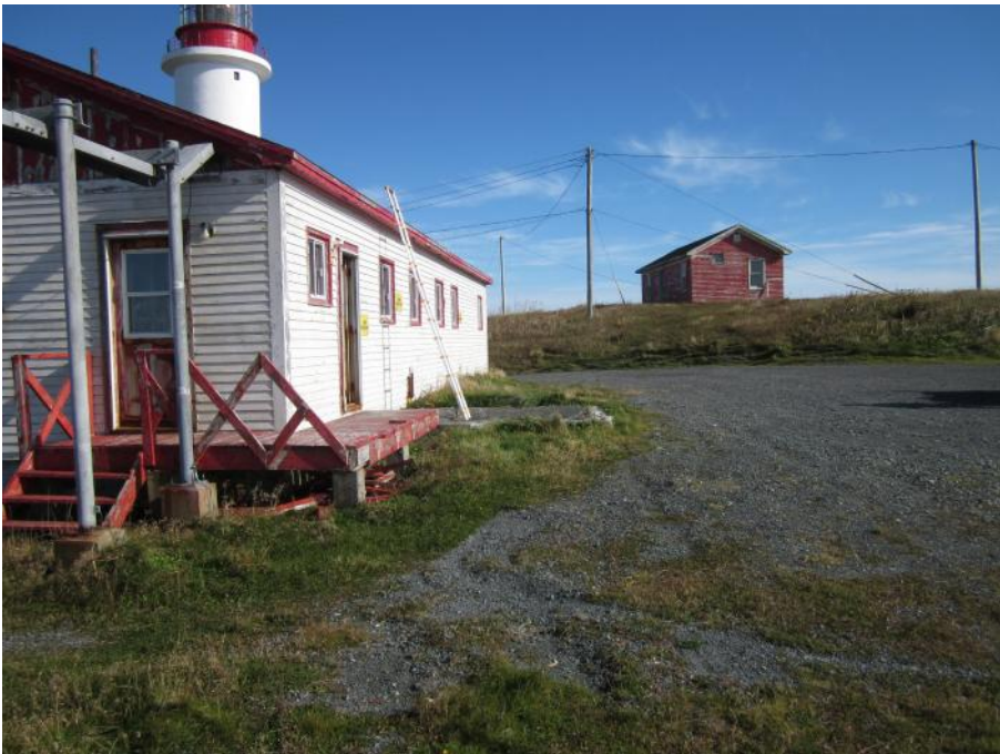
Photo 3: View of the Former Dwelling with the Light Tower and Former Generator Building in the background.
