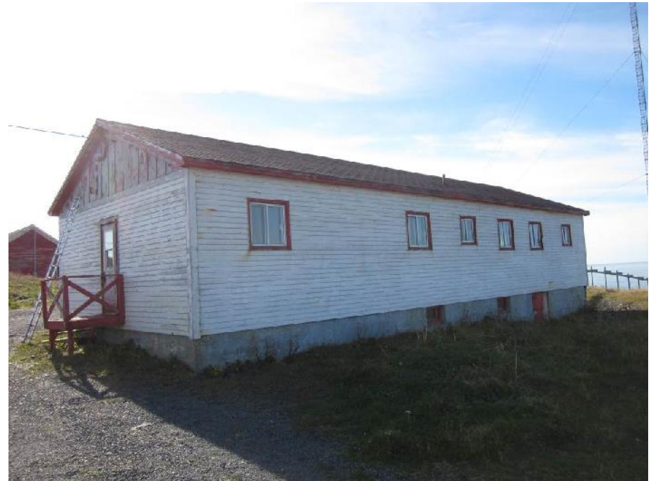
Photo 2: View of the north side of the Former Dwelling.
