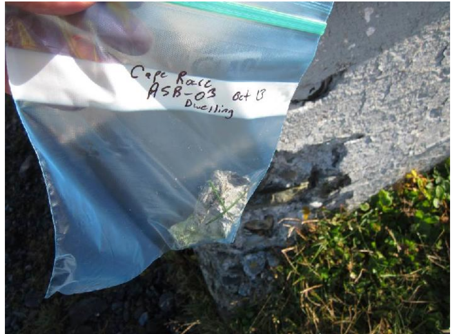
Photo 22: View of location of concrete sample ASB-03 (exterior foundation wall).
