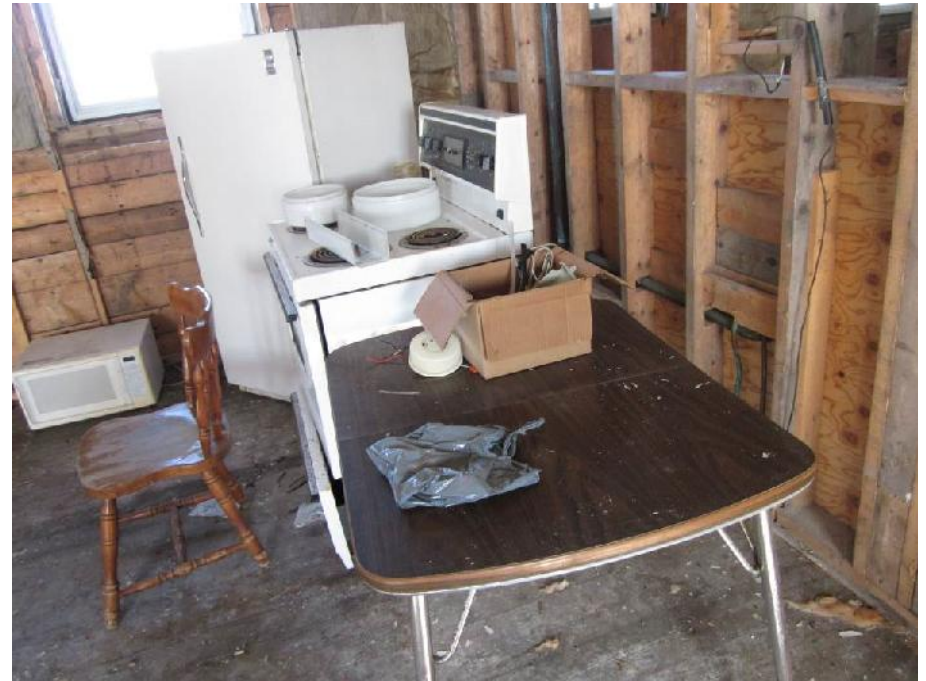
Photo 58: View of copper piping in Room 3. Note smoke detector on table.
