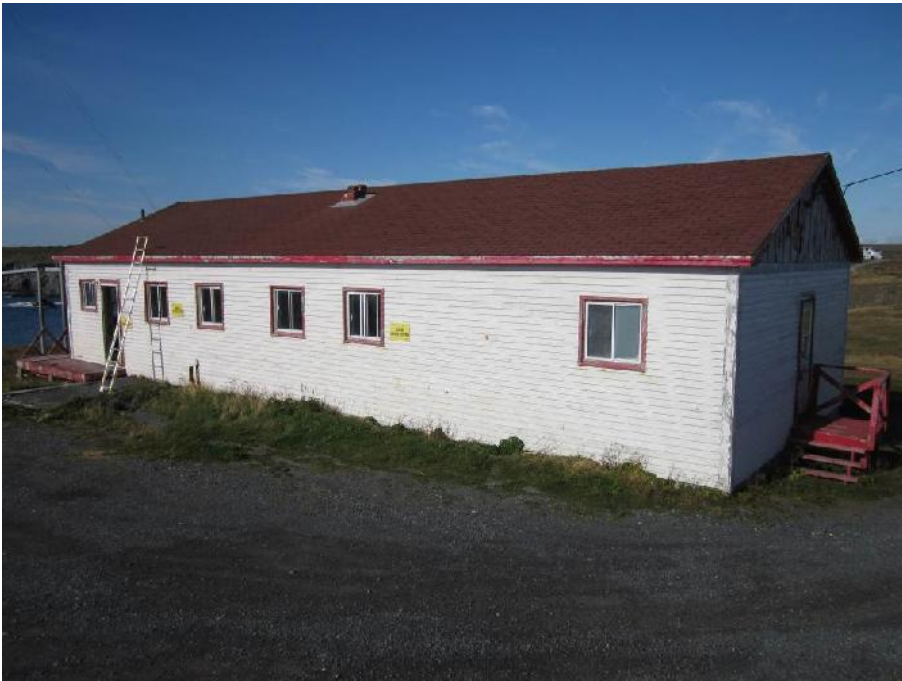
Photo 1: View of the south side of the Former Dwelling. Note side deck on the right.
