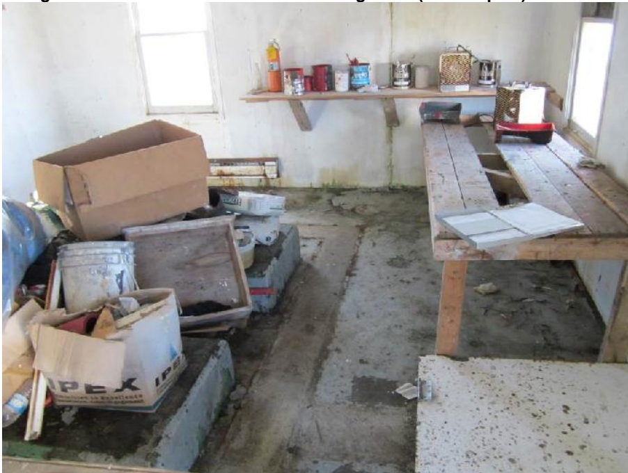
Photo 7: View of Room 1 in the Former Generator Building.
