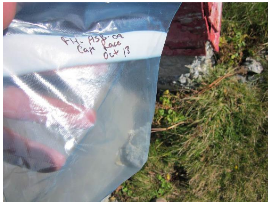
Photo 22: View of location of concrete sample FH-ASB-09 (exterior wall).
