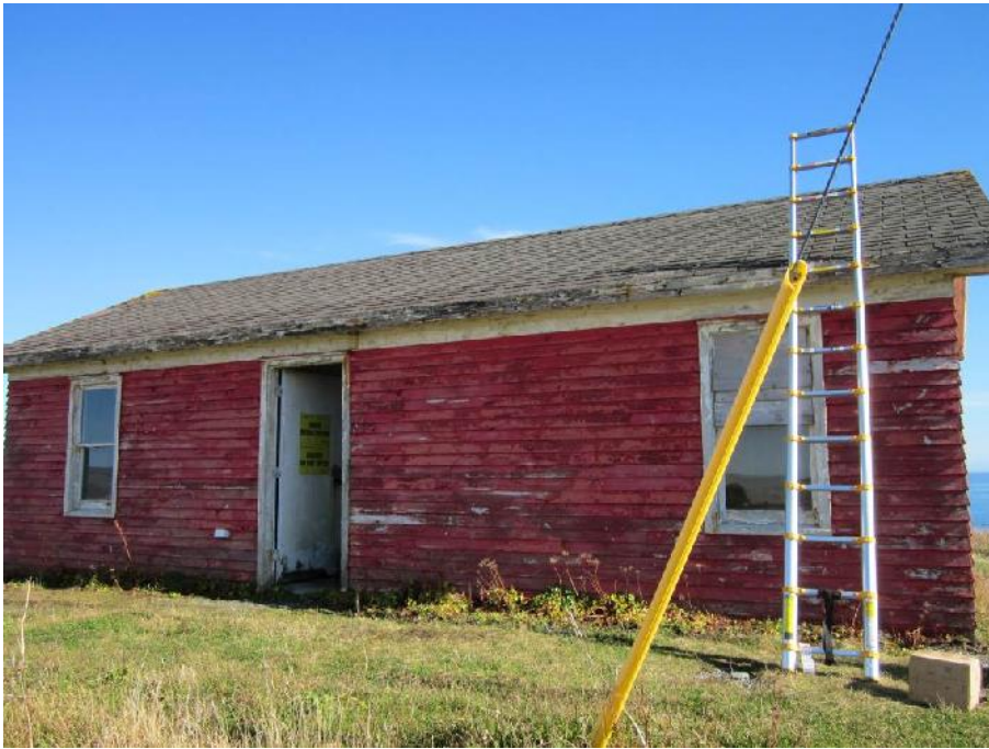
Photo 1: View of the northwest side of the Former Generator Building.
