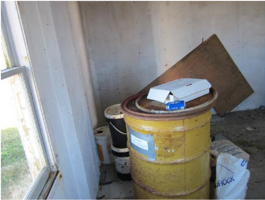
Photo 13: View of a 45 gallon drum (spill kit) and 5 gallon pails (hydraulic oil) in Room 2 of the Former Generator Building.
