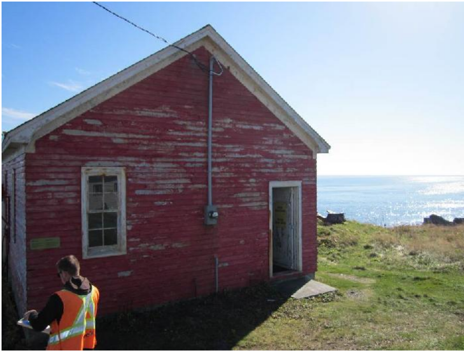
Photo 1: View of the northwest side of the Former Fog Horn Building.
