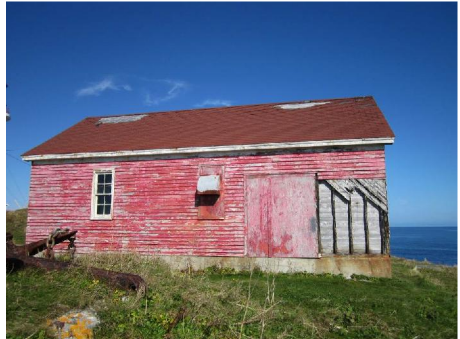
Photo 4: View of the southwest side of the Former Fog Horn Building.
