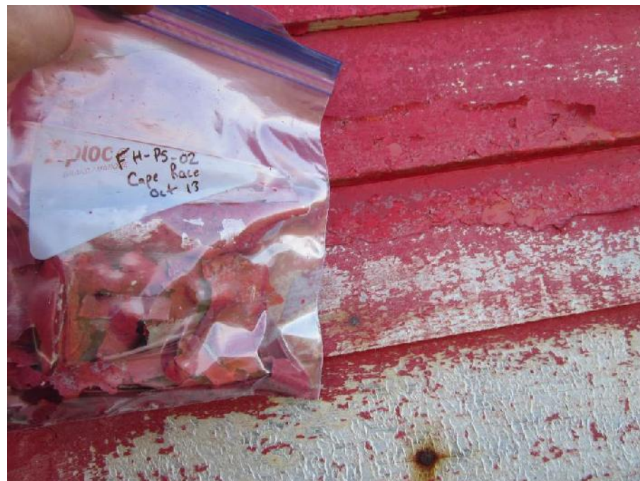
Photo 24: View of location of paint sample FH-PS-02 (exterior wall).
