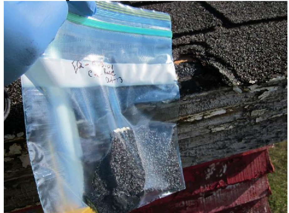
Photo 16: View of location of shingle and tar sample EQ-ASB-01 (roof).
