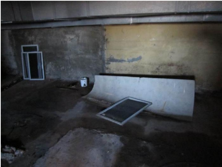
Photo 17: View of the basement (Room 12) of the Former Dwelling.
