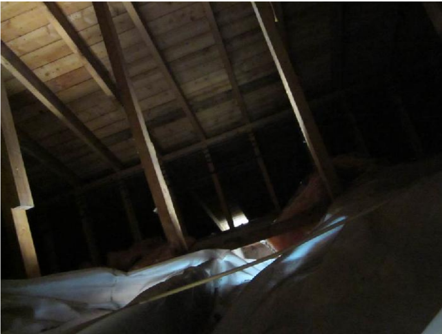
Photo 5: View of the attic in the Former Dwelling.
