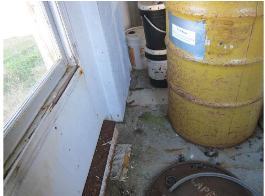
Photo 14: View of electrical baseboard heater in Room 2 of the Former Generator Building.
