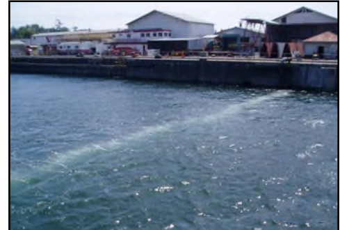
Bubble curtain employed during vessel transfer.
