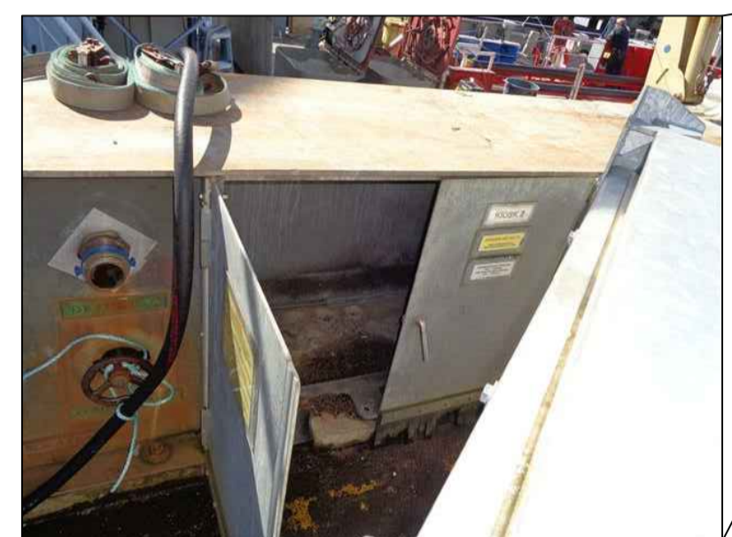
EXISTING KIOSK #2 SHELL. TO BE MAINTAINED.
