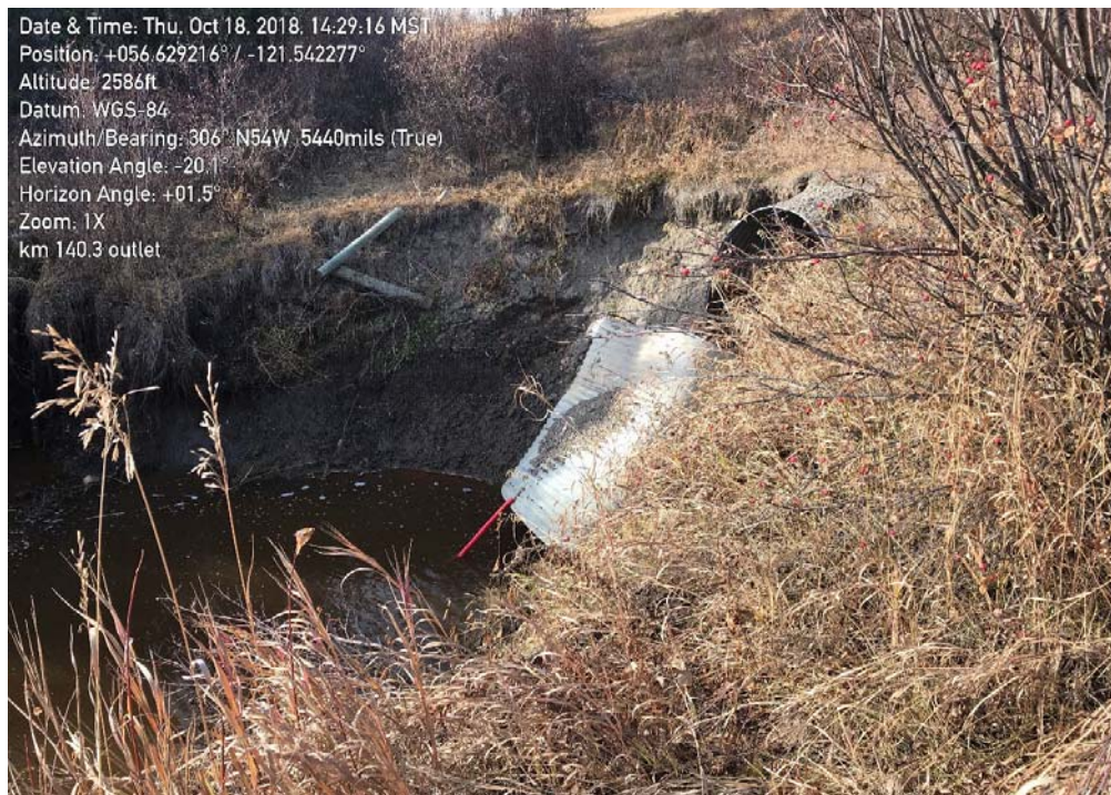
Photo 1: Scour Pocket and Culvert Failure at Outlet
