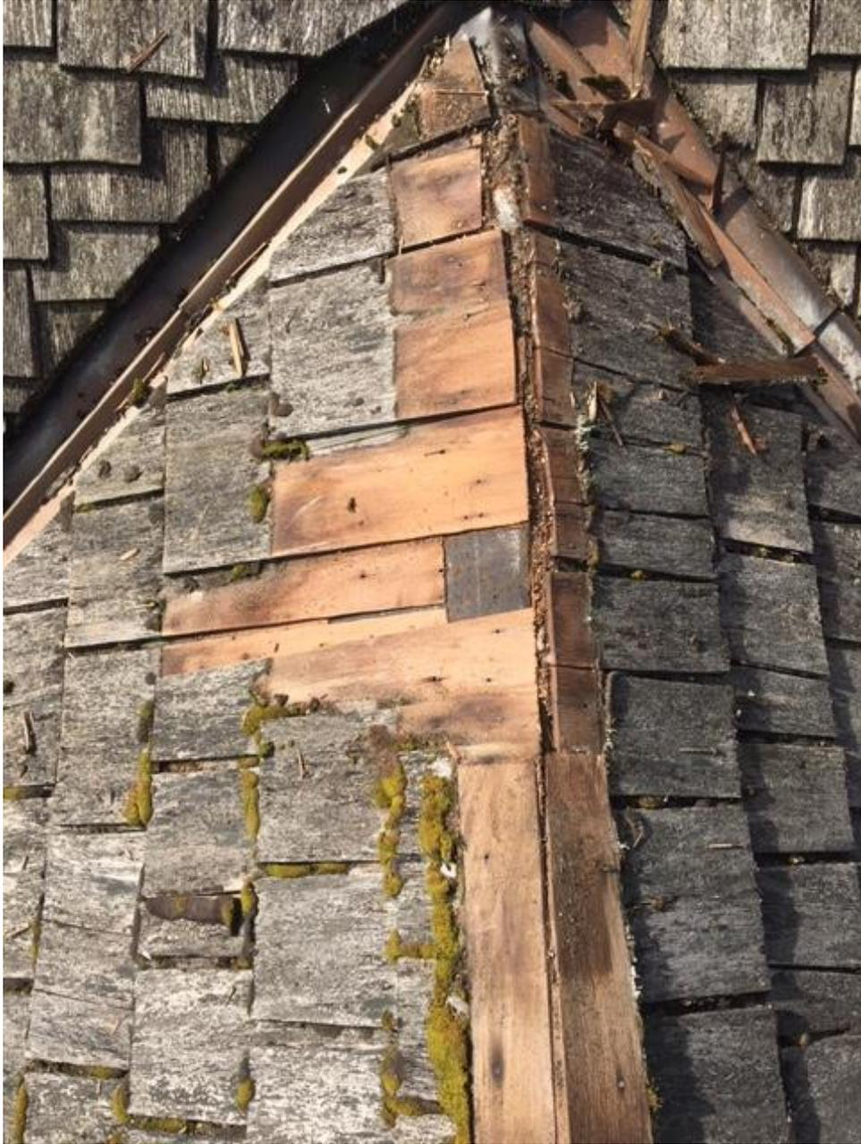
Lodge Building - Non-asbestos felt beneath cedar shingles.
