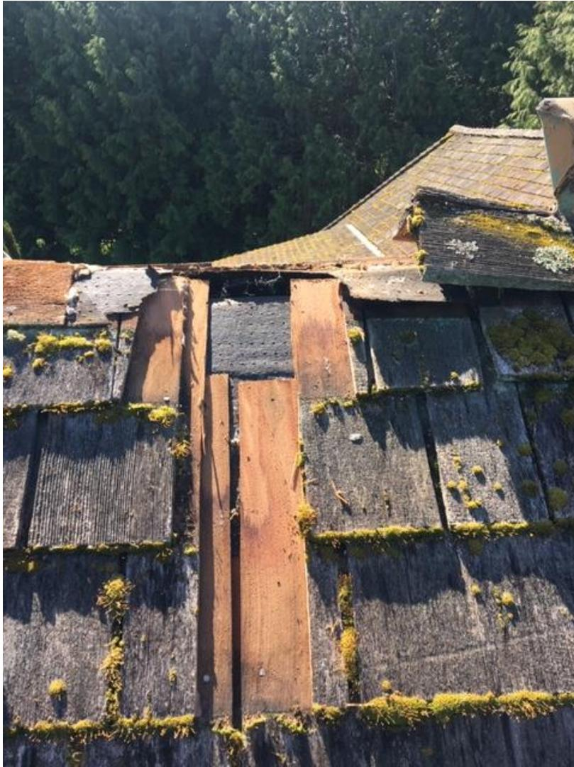
Science Building - Non-asbestos felt beneath cedar shingles.
