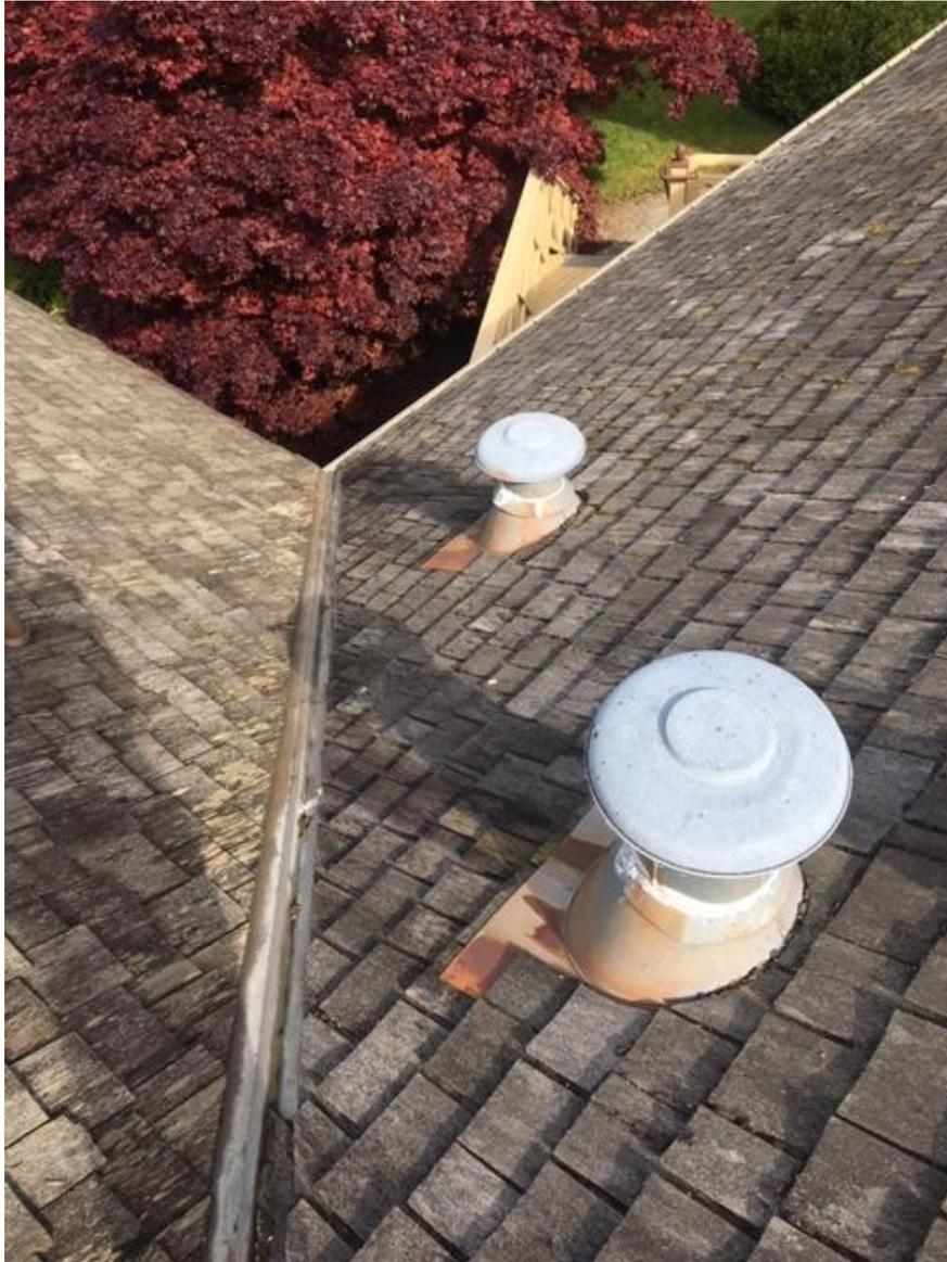
Lodge Building - Non-asbestos caulking on roof vents.
