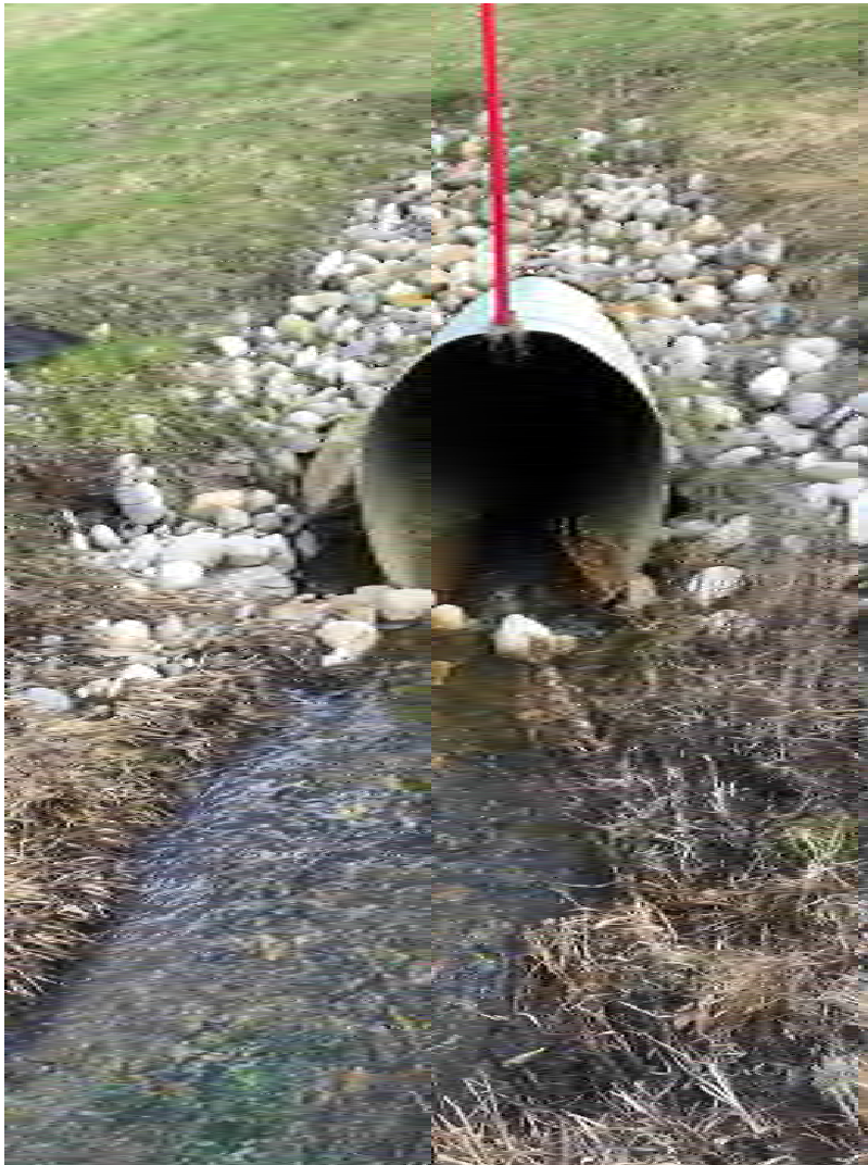
Photograph D-3: Culvert crossing Inlet looking Northeast (approximately Km 155+120)
