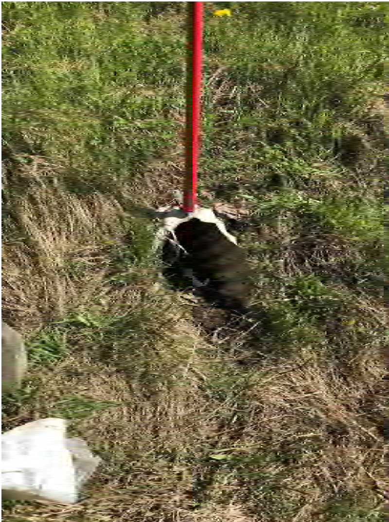
Photograph D-2: CSP culvert on West Highway fill
