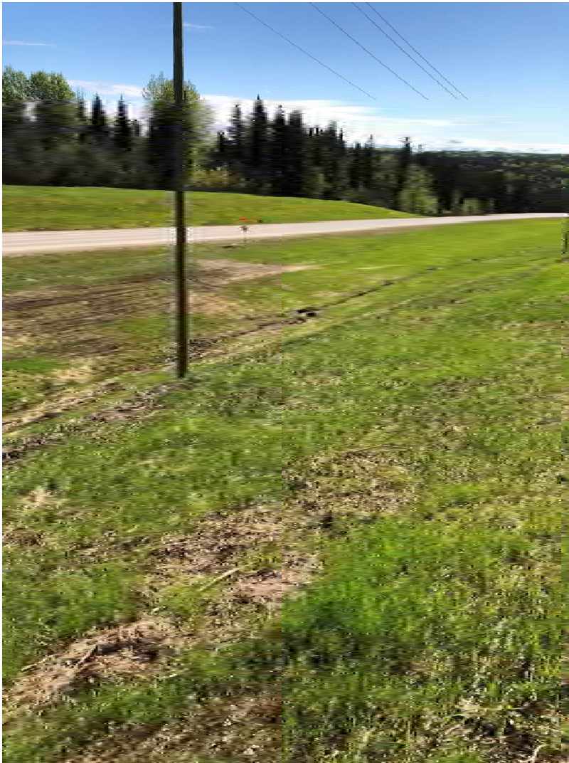
Photograph D-6: Ditch on the southwestern side of Alaska Highway (looking East)
