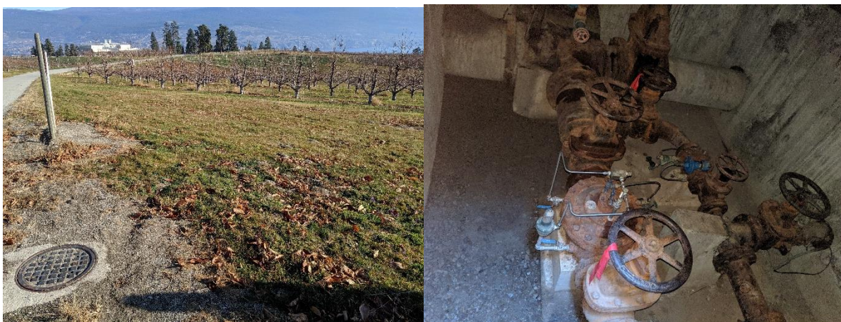
Photo 2.1 Existing PRV Station / Manhole
