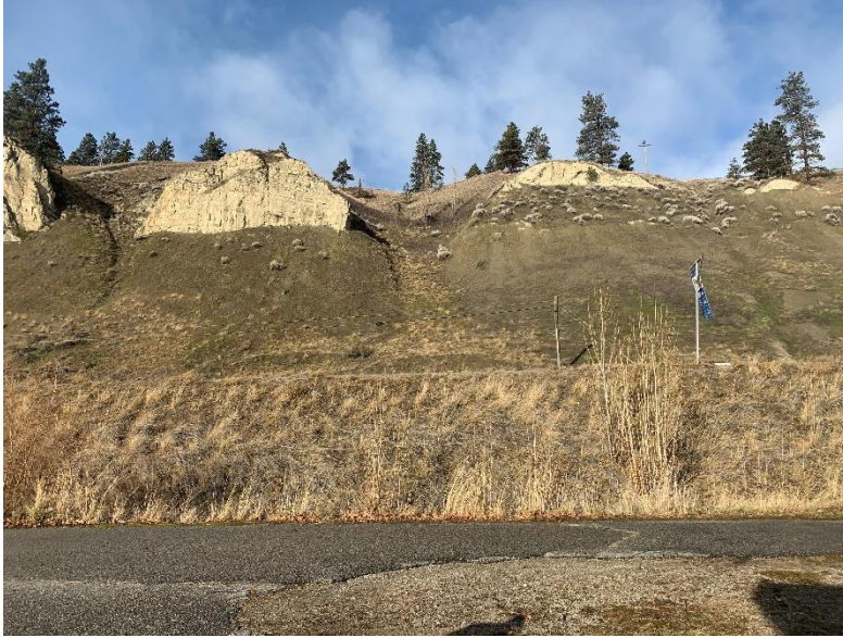
Photo 2.3 Approximate location of mainline highway crossing/embankment looking upstream from the pumphouse
