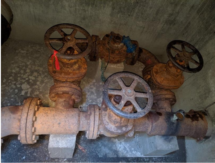
Photo 2.2 Existing PRV Station / Manhole
