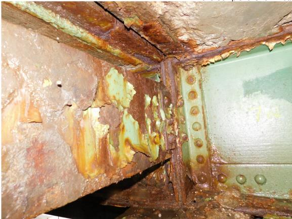
97 N Approach Span, Heavy Wet and Severe Corrosion on Diaphragm @ Stringers 6&7 under Exp Joint with N Tower
