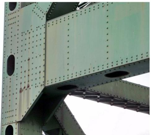
222 North Tower, Local Light Rust on Gusset Plate at top NE Corner of Panel 1, looking East Page A2 [111] of A2 [169]
