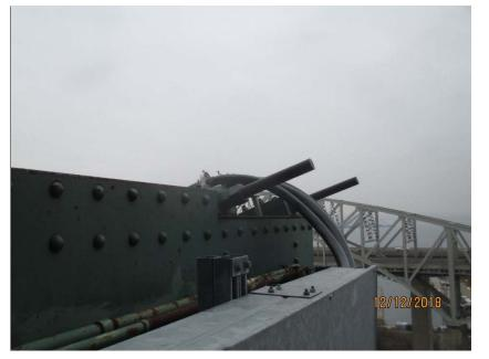
Photo E65 Typical Aerial Suspension Cables Routing. Sufficient bending radius has been created for the aerial cable before routing into the cable tray.
