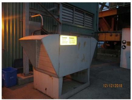
Photo E8 Main Standby Generator Load Bank. This load bank is located outside the control house and is appropriately sized to exercise the main (600kW) standby generator under load. Note the minor corrosion exhibited on the load bank enclosure.
