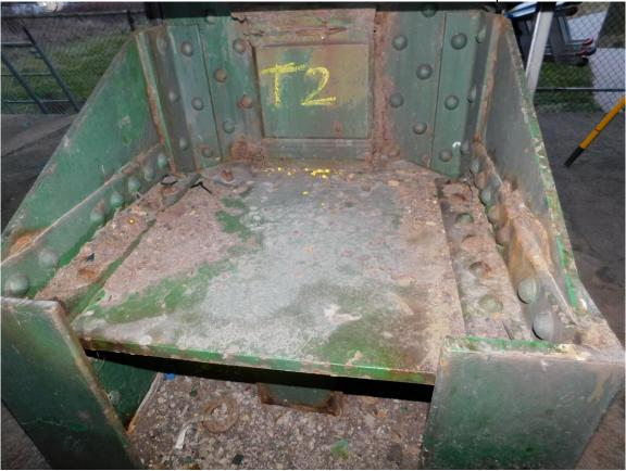
197 North Tower, Typical Local Corrosion on Top Exterior Surface Anchor Assembly, NW Rear Column T3 Shown
