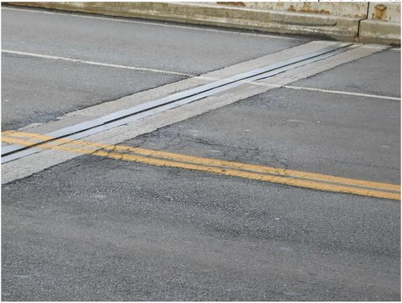
111 North Approach Span, Large Unsealed Pattern Cracks on Central North End of Deck
