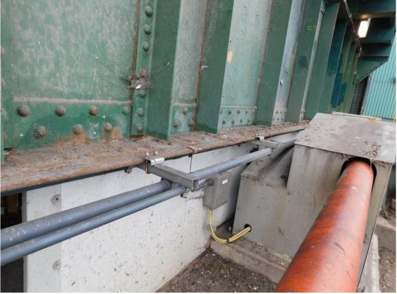
151 South Tower, Light Surface Rust on bottom Flange Section of Front Floor Beam (TYP)
