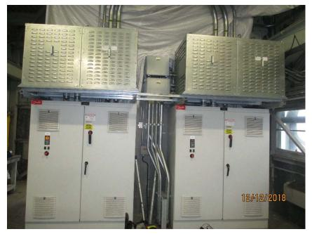
Photo E21 Typical VFD Drives Enclosure with Braking Resistors. Two new drives with resistors were installed in each tower as part of the recent recent motor and drive replacement project. Both drives are in as new condition. Note two drives are providing redundancy for the main drive operation. Operator can select drives automatically or manually.
