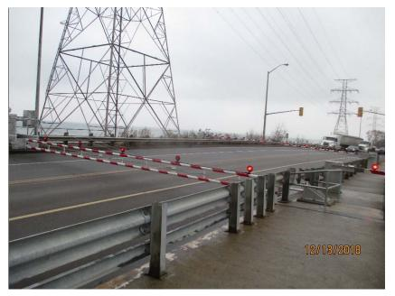
Photo E59 Typical Barrier Gate. Note the newly installed barrier gate, including arm light flasher and gong. The gate is in as-new operational condition.
