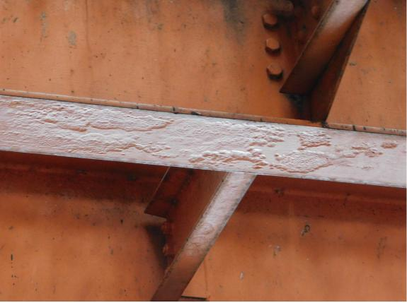
271 Typical Painted-over Pitted Stringer Surface at Lift Span, Stringer 6 in Bay 12 Shown
