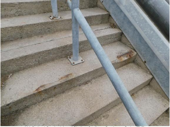
333 Stained Cracks & Local Shallow Spalls on Southwest Stairs (TYP)
