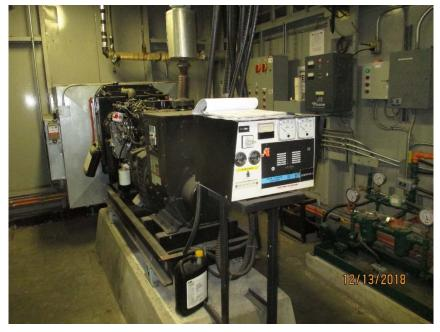
Photo E5 Auxiliary Standby Generator. Note auxiliary standby generator only provides power to bridge facility and auxiliaries in the event of a utility electric failure. It is not capable of providing power to operate the bridge. This generator is in acceptable and serviceable condition.
