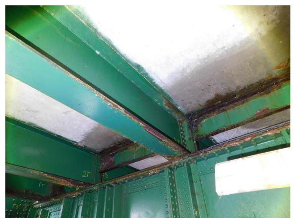
118 South Tower Span, Typical Heavy Wet Areas at South End of Soffit at Expansion Joint wth South Approach Deck Page A2 [59] of A2 [169]
