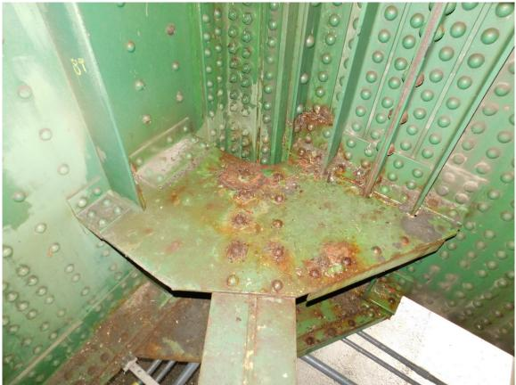
184 Typical Light Rust on Gusset Plate at Bracing Connection to Tower Column, NW Column at North Tower Shown Page A2 [92] of A2 [169]
