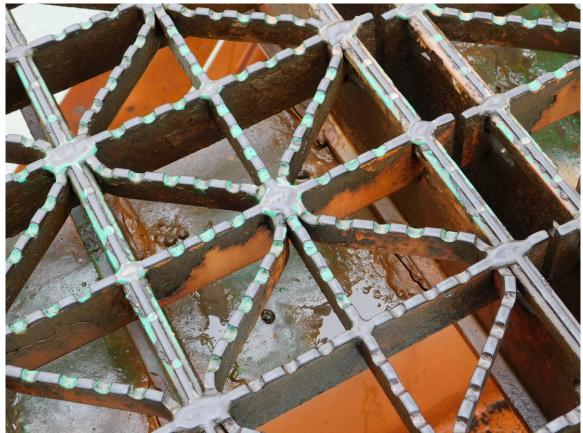
236 Cracked Hold-down Weld @ Grating to Stringer 9 in Central Section of 4th Bay from South Page A2 [118] of A2 [169]
