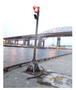
Photo E49 Typical Marine Traffic Navigation Light. The marine traffic lights are located at the tip end of the pier for signaling approaching vessels. The lights were operational at the time of the inspection and exhibit moderate corrosion on lighting fixture visors and poles.
