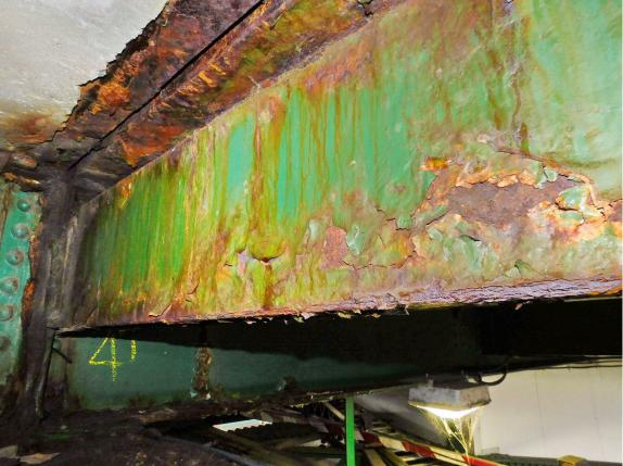
85 S Approach Span, Typical Heavy Wet with Local Severe Corrosion on Diaphragm under Exp Joint with S Tower Span
