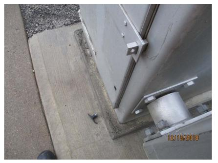
Photo E61 Broken Lock on North Barrier Gate Enclosure. North barrier gate enclosure lock was broken at the handle and left on the floor as indicated.
