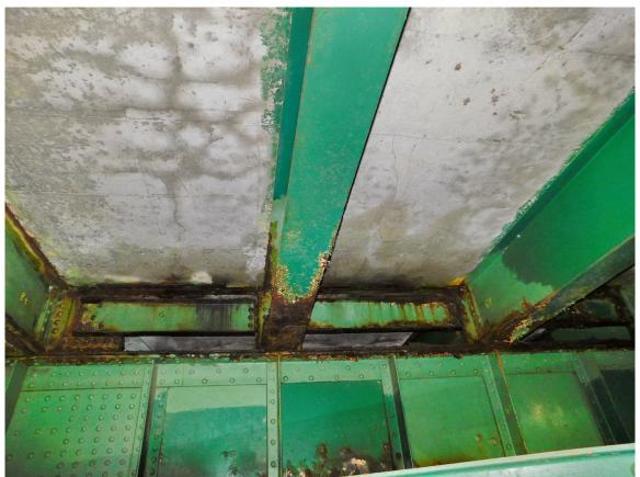
128 North Tower Span, Large Wet Areas on Soffit at NW Section of Deck, Stringers 6 to 8 Page A2 [64] of A2 [169]
