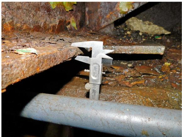
94 N Approach Span, Severe Corrosion on Bottom Flange of Stringer 8 at North Abutment End (TYP) Page A2 [47] of A2 [169]
