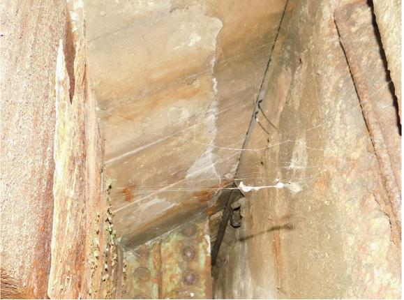
69 Stained Cracks & Large Delamination on North Abutment End Soffit between Stringers 4&5
