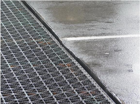
307 Severe Abrasions on Top East Section of End Plate for Open Gap Expansion Joint @ South Tower & Lift Span
