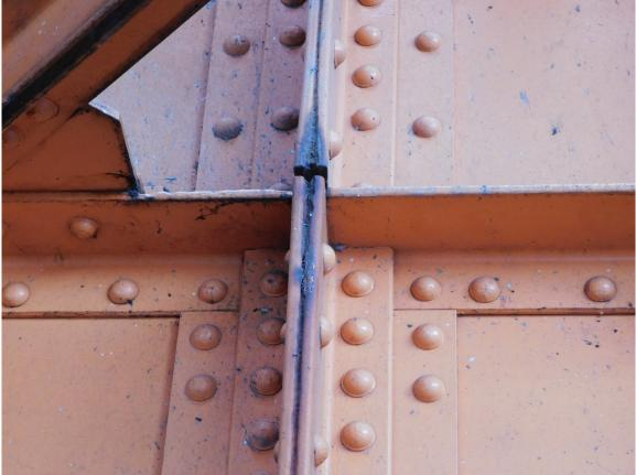
267 Localized Rust Jacking on Stiffener Angles on North Floor Beam A13-B13 (TYP)
