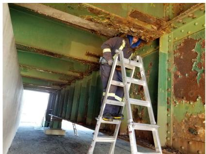
North tower main support beam. Several severe patches of corrosion identified.
