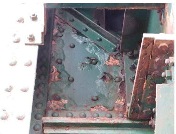
152 South Tower, Local Light-Medium Corrosion on Stiffener Plate at Top East Corner of Front Floor Beam Page A2 [76] of A2 [169]
