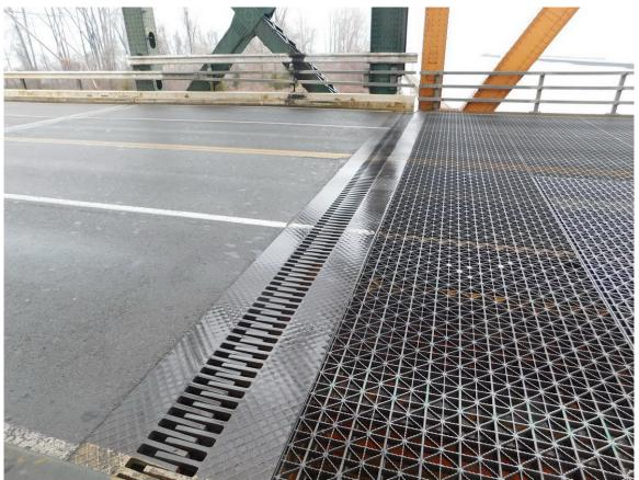
306 Open Gap Finger Plate Expansion Joint @ North Tower & Lift Span Decks, looking East Page A2 [153] of A2 [169]
