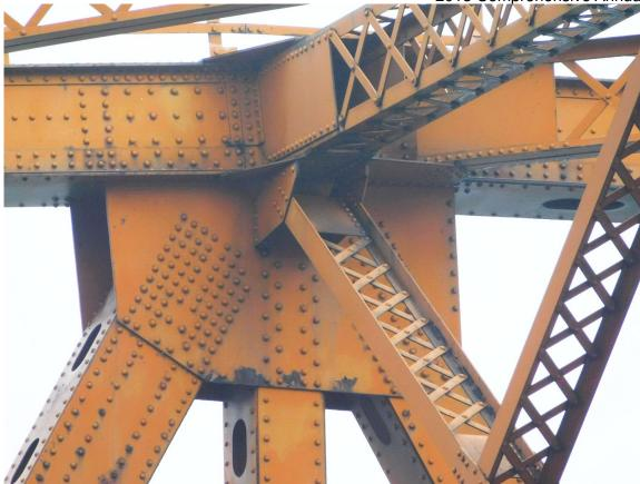
285 Typical Peeled Paint Coating at Upper Truss Connection, North BT10 Shown
