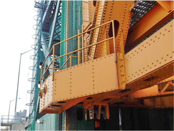
277 Southeast Lower Guide Roller Assembly at Lift Span
