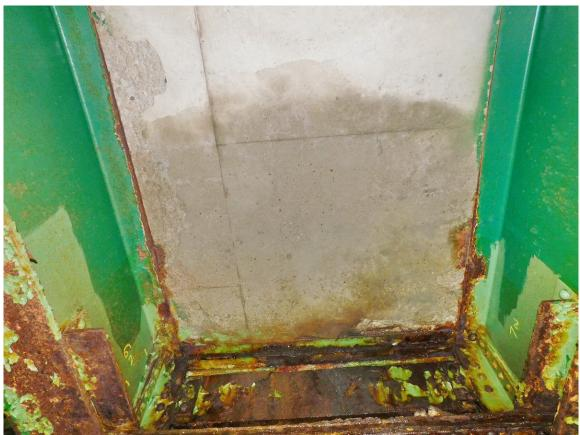
72 Heavy Wet Area on SW Section of North Span Soffit between Stringers 6&7 Page A2 [36] of A2 [169]
