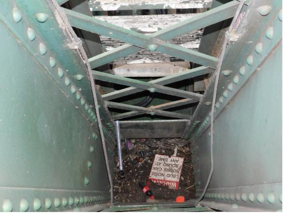
221 Typical Debris on Interior Plate below West Sidewalk at North Tower
