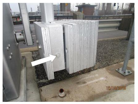
Photo M36 North Barrier Gate. The gate arm counterweight has a bolt that is not fully seated at the east side of the counterweight.
