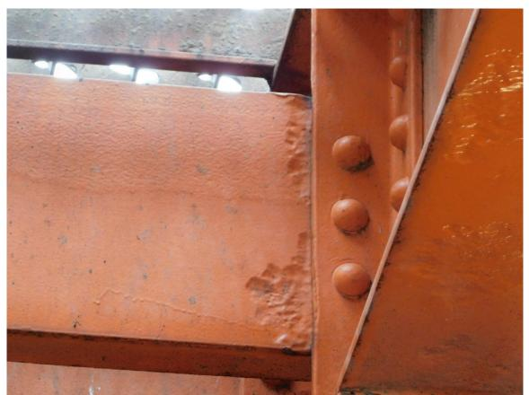
272 Typical Painted-over Pitted Diaphragm Surface at Stringer Connection, Stringer 9 at Bay 1 Shown Page A2 [136] of A2 [169]
