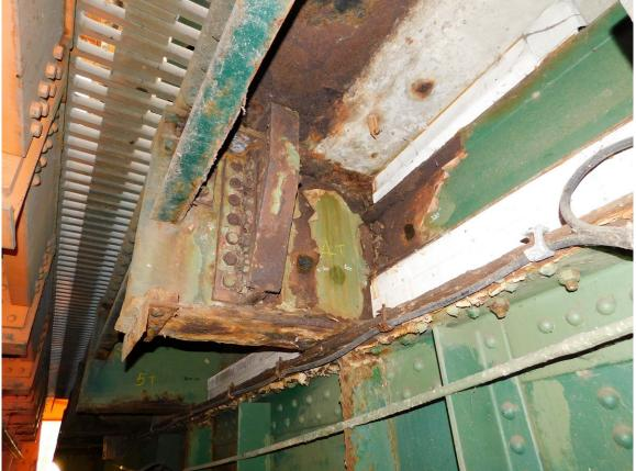
137 North Tower Span, Local Medium-Severe Corrosion on Stringer 4 and Diaphragm near Exp Joint with Lift Span
