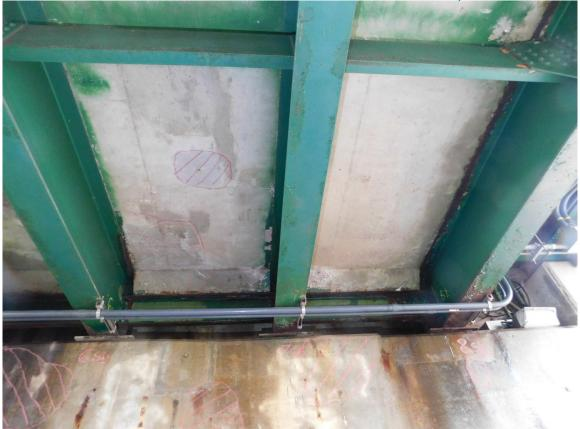
49 Wet Areas with Local Severe Delamination on SW Section of South Approach Soffit, looking South
