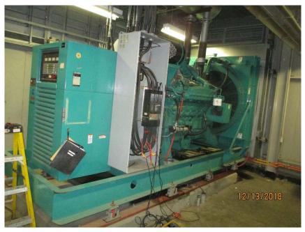
Photo E4 Main 600kW Standby Generator. Generator is used as an alternative source of power to operate the bridge. The standby generator has been well maintained and is tested monthly.
