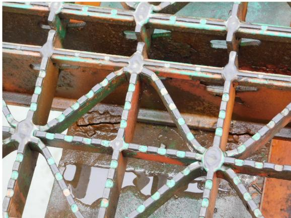
238 Cracked Hold-down Weld @ Grating to Stringer 9 South of Floor Beam A6-B6 Page A2 [119] of A2 [169]
