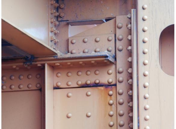
269 Typical Localized Area of Surface Rust on Steel Floor Beam, Beam A2-B2 looking North Shown
