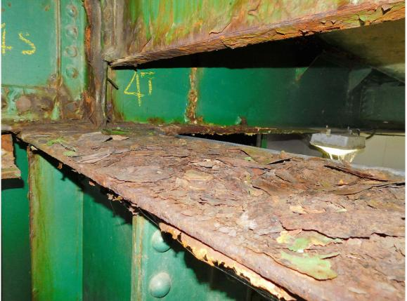
149 South Tower, Heavy Corrosion on Top Flange of Rear Floor Beam below South Exp Joint with South Approach Span
