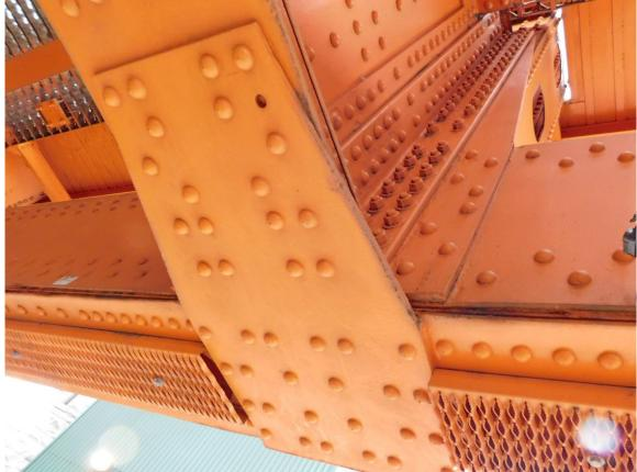
259 Typical Truss Bottom Chord Connection at Intermediate Floor Beam, Node Point B2 Shown
