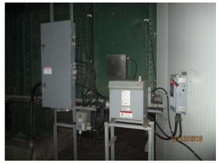
Photo E47 Lighting Panel on North Pier (LP-4). The disconnect switch, transformer, lighting panel and the lighting contactor are is in good physical condition. The lighting contactor has been modified to work with the current bridge control system.
