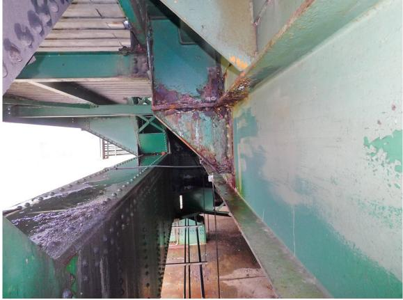
139 North Tower Span, Local Light-Medium Corrosion on Exterior Face of Stringer 8, looking North
