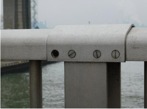
315 Missing Nut on Splice Bolt for Top Handrail @ Post near Mid Section of Lift Span
