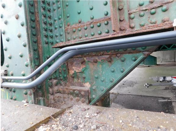
153 South Tower, Local Light-Medium- Corrosion on Stiffener Plate at Bottom East Corner of Front Floor Beam
