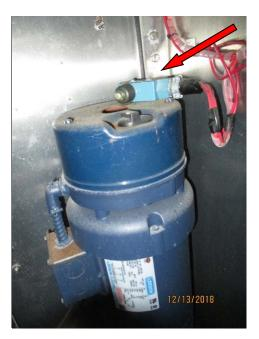
Photo E56 Typical Traffic Gate Motor and Hand Crank Limit Switch. The components were found to be in as-new condition. Note that the gate is provided with a hand crank limit switch (arrow) for interlocking proses.
