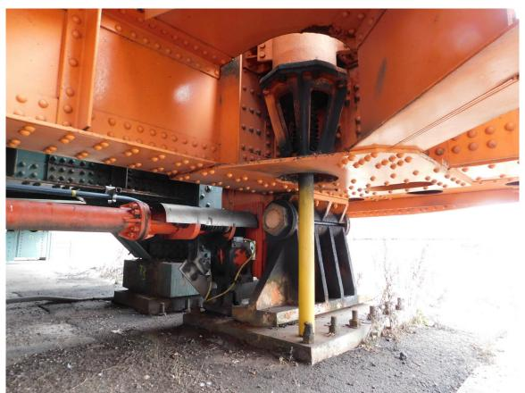
292 Rocker Bearing & Air Cushion at Northeast Corner of Lift Span
