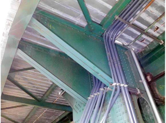
323 Typical Stand-off Brackets Supporting Sidewalk at South Tower Column
