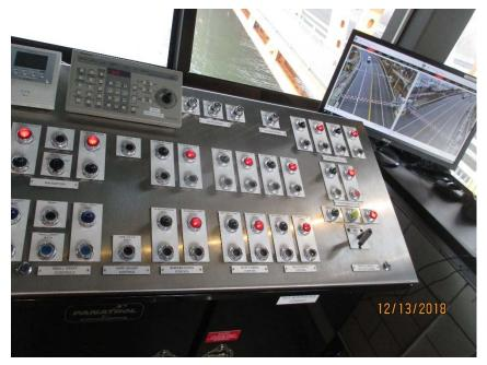
Photo E15 Traffic Control Panel. The new traffic control console top was recently installed and is in like new condition.
