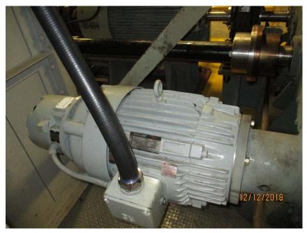
Photo E26 Typical Auxiliary Drive Motor. The new auxiliary motor with integral brake was installed during the recent motor and drive replacement project. Note that the original chain drive aux. has been changed to the direct coupling to the reducer.
