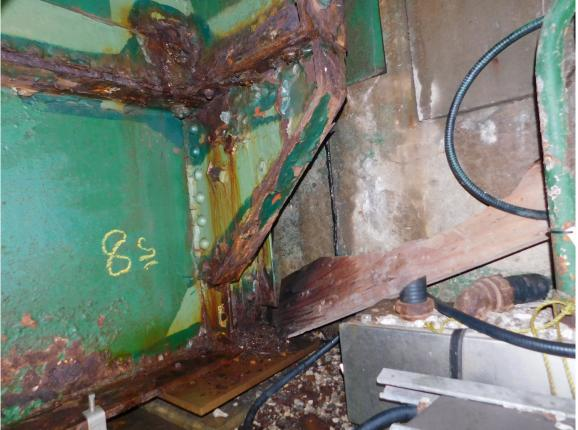
87 S Approach Span, Wet with Local Severe Corrosion on Stringer 8 at South Abutment End
