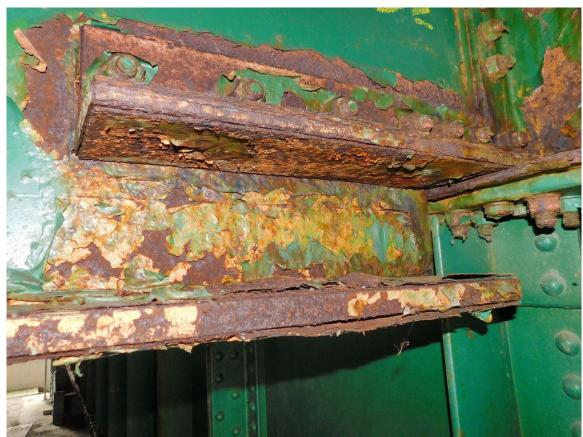
84 S Approach Span, Medium Corrosion on bottom North End of Stringer 3 (TYP) Page A2 [42] of A2 [169]
