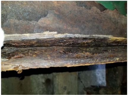
Severe delamination on diaphragm flange
