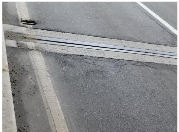
110 North Approach Span, Light Asphalt Depression with Local Unsealed Pattern Cracks on NW Corner of Deck Page A2 [55] of A2 [169]
