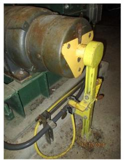
Photo E43 Typical Span Lock Motor. Note the lock motor is in fair physical condition but exhibits moderate corrosion. The hand crank limit switch was been replaced during the recent motor and drive replacement project, to prevent electrical operation of the lock motor when the hand crank cover is removed.
