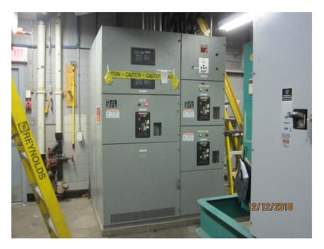
Photo E3 Switchboard #1. The switchboard was installed in approximately 1994 and is in good condition. Note the yellow tape on the metering compartment door. There are some unterminated live wires inside the metering compartment.
