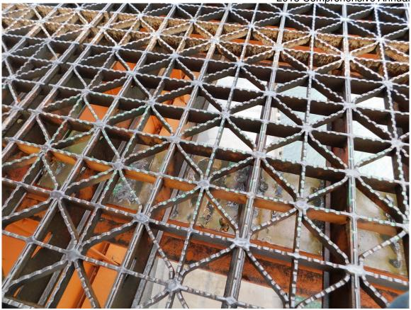
229 Typical Deck Grating & Visible Top Surface of Steel Stringer on Lift Span Bridge Deck
