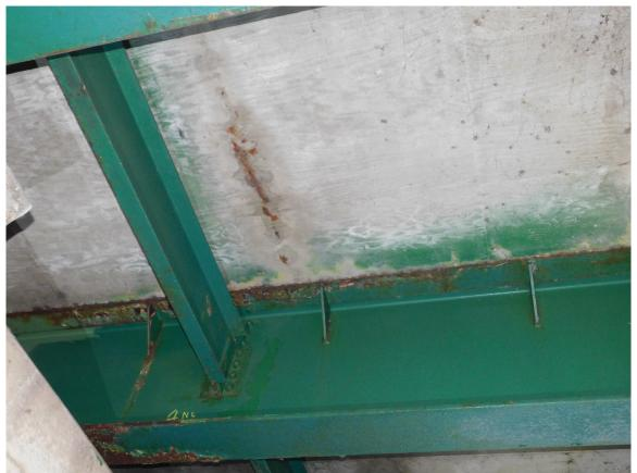
68 Crack with Wet & Rust Stains on South Central Section of North Approach Span Soffit Page A2 [34] of A2 [169]
