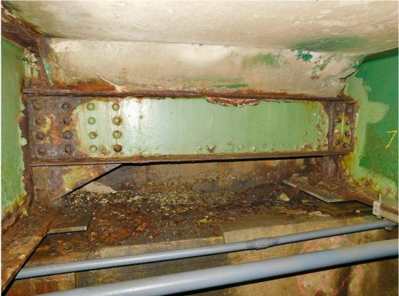
91 N Approach Span, Typical Heavy Corrosion on Stringers & Diaphragm at North Abutment, Stringers 7&8 Shown
