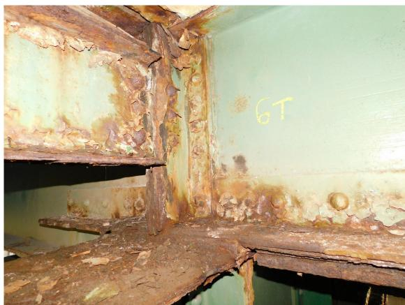
136 North Tower Span, Local Severe Corrosion on Diaphragm & Stringer 6 under Expansion Joint at North End of Span Page A2 [68] of A2 [169]
