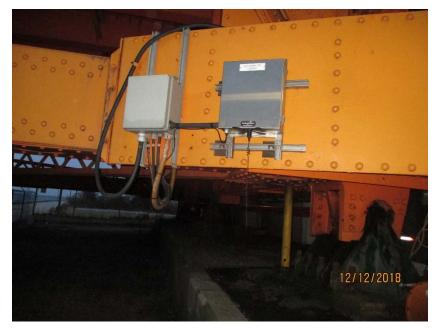
Photo E39 Span Inclinometer Enclosure. Per the recent motor and drive replacement project design, the span inclinometer was to be installed in the enclosure and to communicate wirelessly with a transmitter located inside the CP-2 enclosure. The inclinometer was to be used for the span skew control but does not presently function as intended and has been disconnected.
