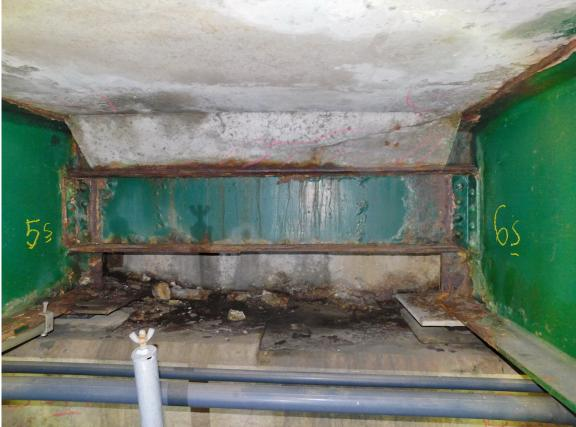
79 S Approach Span, Typical Heavy Corrosion on Interior Stringers & Diaphragm at South Abutment, Stringers 5&6 Shown
