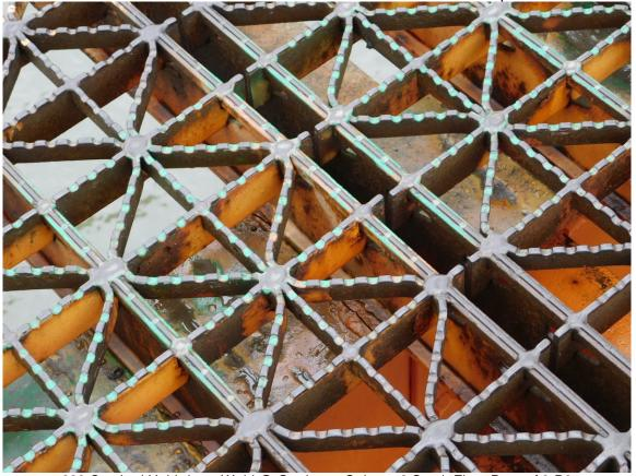
239 Cracked Hold-down Weld @ Grating to Stringer 8 South Floor Beam A8-B8
