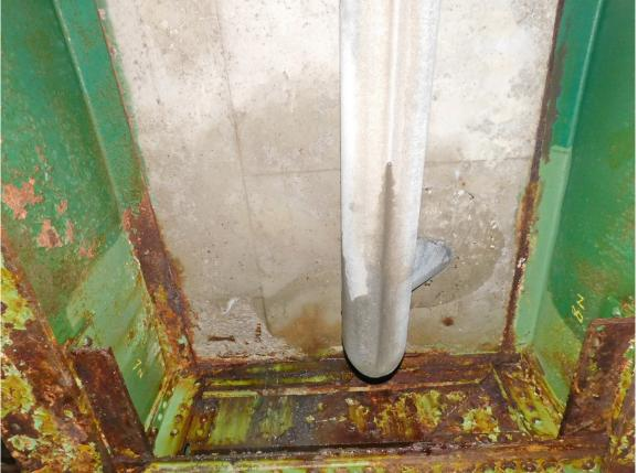
73 Large Wet with Local Severe Spall on North Span between Stringers 7&8
