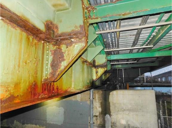
99 N Approach Span, Heavy Corrosion on Outside Face of Stringer 8 @ Central Section of Span, looking South
