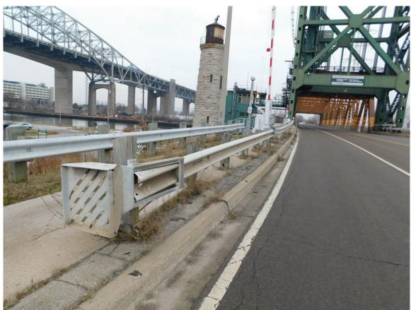
328 Extruder End-Treatment at End of SW Approach Guiderail, looking North Page A2 [164] of A2 [169]
