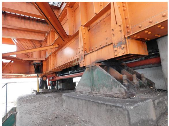
294 North Centering Bearing at North End of Lift Span, looking West
