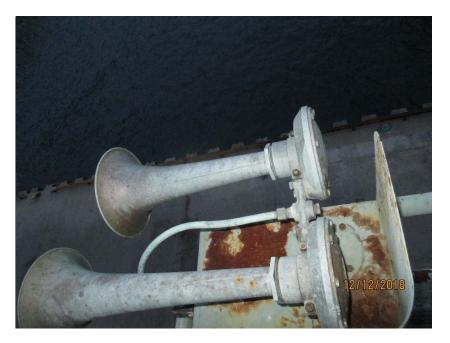
Photo E69 Typical Air Horn. The air horn is operational and is in serviceable condition. Note the moderate corrosion on the air horn housing.
