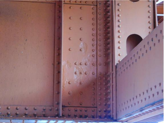
273 Painted-over Pitted West Section of Floor Beam A12-B12 Surface (TYP)
