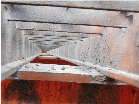
240 Typical Hold-down Weld between Deck Grating to Steel Stringers Page A2 [120] of A2 [169]
