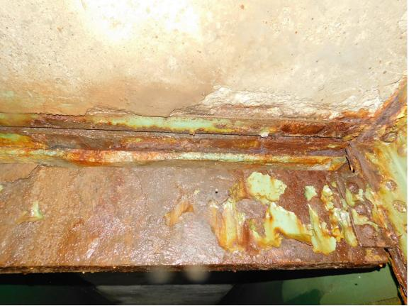
75 Local Severe Delamination on South End of North Span Soffit between Stringers 6&7
