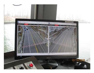
Photo E17 CCTV and Intercom. A CCTV monitor for new CCTV cameras is located next to the traffic control console. Note that both CCTV and intercom system are original and are functional. Also note that an original CCTV CRT monitor and original cameras that were installed prior to the recent motor and drive replacement project and remain in service. The intercom unit is located at the top right corner of the control console.
