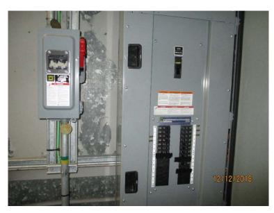
Photo E36 Typical New Lighting Panel and Disconnect. A 45kVA transformer primary disconnect switch and associated lighting panel were installed as part of the recent motor and drive replacement project.. These components are in an asnew condition. Note the black electrical tape over the empty space. Breaker space fillers should be used in place of the tape.
