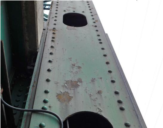
175 Typical Local Peeled Paint showing Light Rust on Tower Column, SE Column T3 at South Tower Shown
