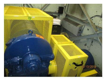
Photo E41 Typical Elevator Motor. The elevator motor is in good physical and operational condition.
