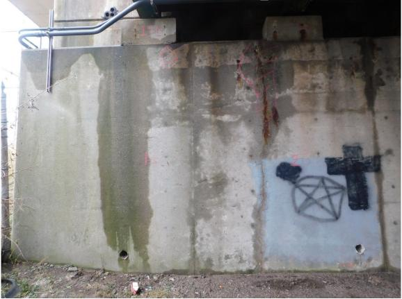
09 South Abutment, Wide Vertical Crack with Rust & Delamination on Wall between Stringers 1&2
