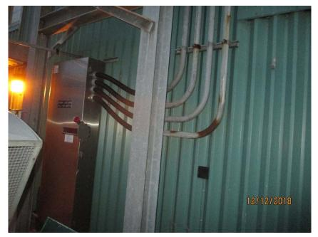
Photo E9 Load Bank Disconnect Switch. The disconnect switch is wall mounted outside the generator room facing the load bank. Note the as-new condition of the disconnect switch.
