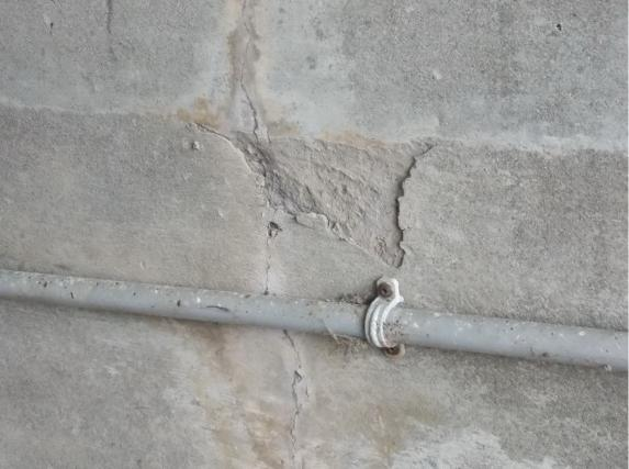
31 Local Minor Spall on East Section of South Curtain Wall
