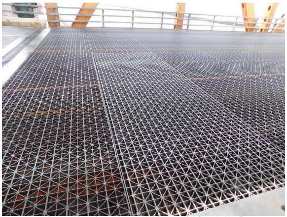
228 Replaced Deck Grating Panel at NW Section of Lift Span, looking East Page A2 [114] of A2 [169]
