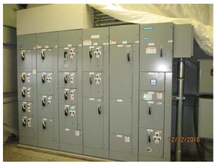
Photo E20 Typical New Motor Control Centre. Note that similar to the findings of last years inspection, the white plastic sheets that cover the MCC which are an indication of a roof leak above the MCC.
