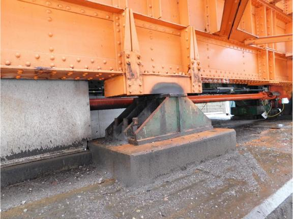
293 Steel Centering Bearing under Central South End of Lift Span
