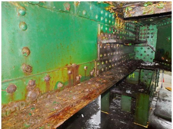
148 South Tower, Heavy Corrosion on Lower NW Section of Rear Floor Beam near SW Tower Leg T4 Page A2 [74] of A2 [169]
