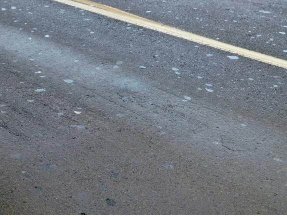
105 South Tower Span, Local Small Area of Light asphalt Depression with Few Light Pattern Unsealed Cracks on SBL
