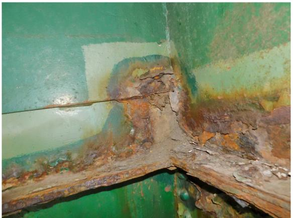
88 S Approach Span, Perforated Curb Plate atop South End of Stringer 8 Page A2 [44] of A2 [169]
