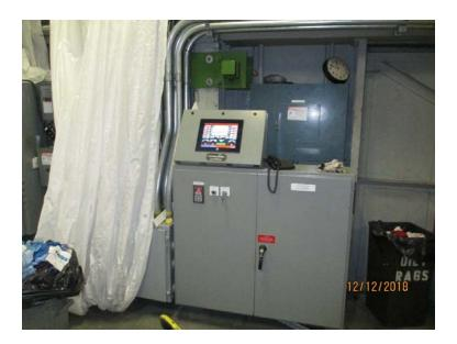
Photo E29 Typical Pull Box and Control Cabinet (CP-3) in South Tower. The control cabinet with PLC display was installed as part of the recent motor and drive replacement project.. They were in as-new condition at the time of the inspection. Note the white plastic sheet cover used to protect enclosure from a roof leak.
