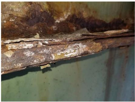
Delamination on girder flanges
