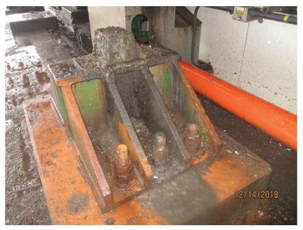
Photo M29 South Centering Device. There is minor debris accumulation on the support. The anchor bolts have paint failure and section loss.
