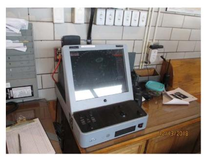
Photo E18 Bridge Radar System. A marine traffic radar system was installed to aid the bridge operation and schedule bridge openings for the boat traffic. It is also capable of displaying wind speed and direction and was found to be operational at the tie of the inspection
