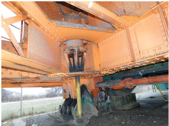
290 Saddle Bearing & Air Cushion @ Southeast Corner of Lift Span, looking East Page A2 [145] of A2 [169]
