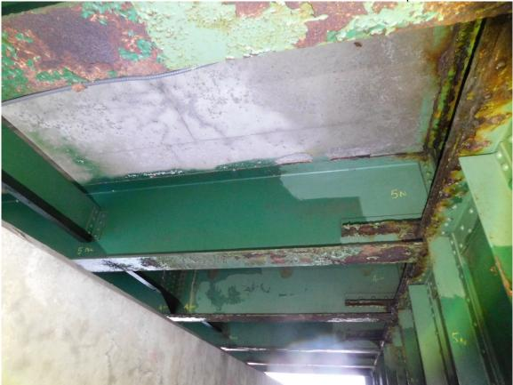
71 Large Wet Areas on South Section of North Span Soffit between Stringers 5&6, looking East
