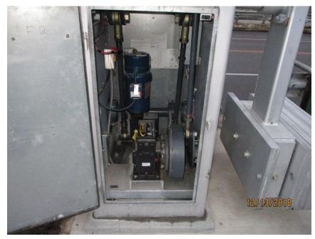
Photo M34 South Barrier Gate. The south barrier gate emitted a groaning sound during each operation.
