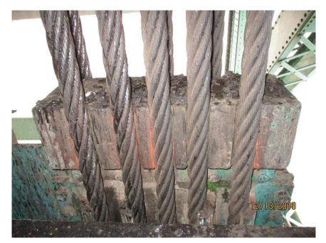
Photo M18 NE-OB Counterweight Rope Connections. Fretting corrosion is present where the counterweight ropes rub against the counterweight splay casting.
