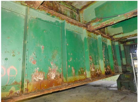
164 North Tower, Local Severe Corrosion on Bottom North Face at West Section of Rear Floor Beam, looking West Page A2 [82] of A2 [169]
