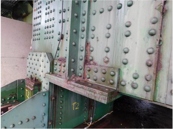
173 North Tower, Local Medium Corrosion on Bottom North Section of West Jacking Girder (TYP)
