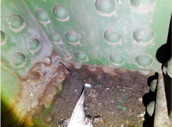
177 Typical Sediment & Local Medium Corrosion on Bottom Interior Surface of Front Columns, NE Column at S Tower
