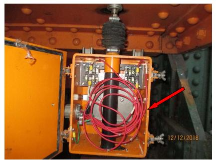
Photo E38 Typical New Span Seated Limit Switch. The switches are of the plunger type and provide indication that the span is fully seated. Note spare wires installed in the switch enclosure are missing cable ties.
