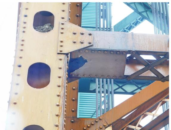
286 Large Built-up of Bird Guano in Vertical Member & Peel Coating of West Truss below Node BT12 Page A2 [143] of A2 [169]
