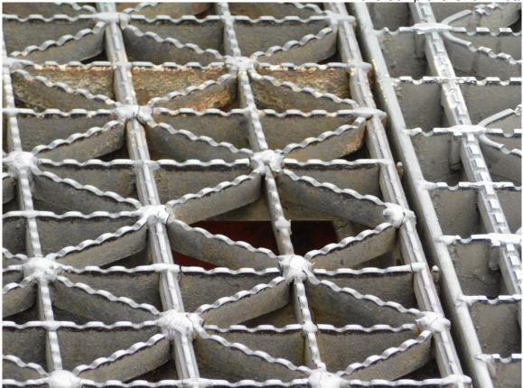
233 Several Cracked Grating & Broken Bearing Bar at North Panel near Stringer 9 and Replaced Panel, looking East
