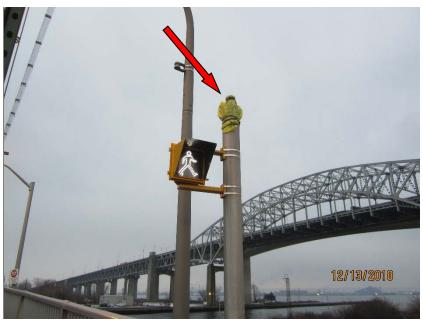
Photo E52 North Pedestrian Light. The pedestrian light is LED type Walk and Halt light. The pedestrian lights functioned properly and were found to be in good condition at the time of the inspection. The North pedestrian bell (arrow) has been completely removed from the pole.
