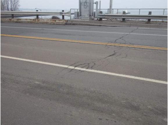
327 Typical Unsealed Pattern Cracks on Approach Road Surface, South Approach Road looking East Shown
