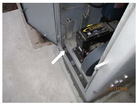
Photo M35 South Barrier Gate. The southeast anchor bolt is loose.
