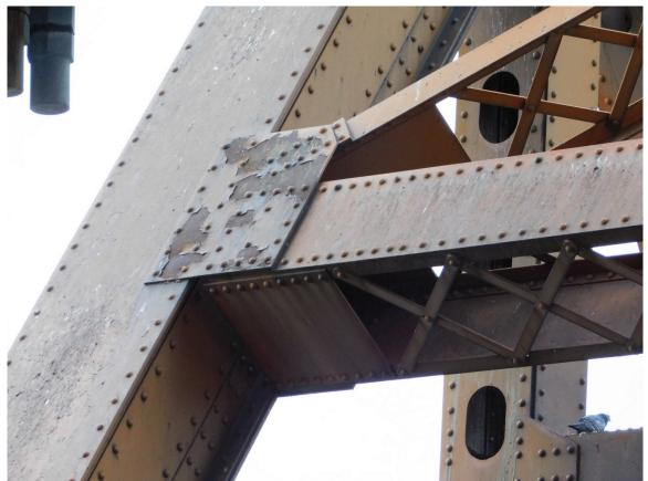
284 Peeled Coating & Light Corrosion on Lower East Gusset at North Portal Truss Page A2 [142] of A2 [169]
