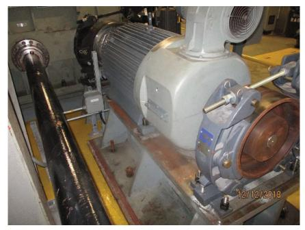
Photo M5 Motor-SW. The motor mounting bolts and support anchor bolts are unpainted with light corrosion forming. The top of the support is also unpainted with light corrosion forming.
