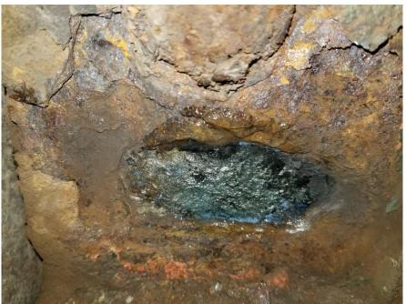
Girder 4S - Severe corrosion
