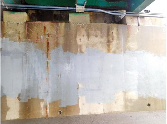
15 Local Severe Delamination Areas on Upper East Section of Wall
