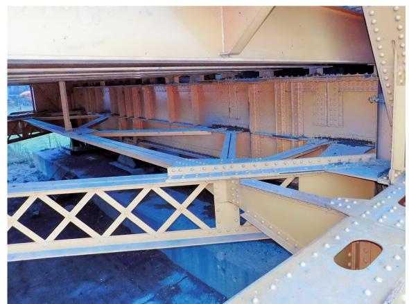
262 Typical Sway Bracing at Main Floor Beam, North Bracing at Floor Beam A13-B13 looking West Shown Page A2 [131] of A2 [169]
