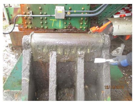
Photo M27 SE Live Load Support. The saddle screw identified by the scraper was found to be hand loose.
