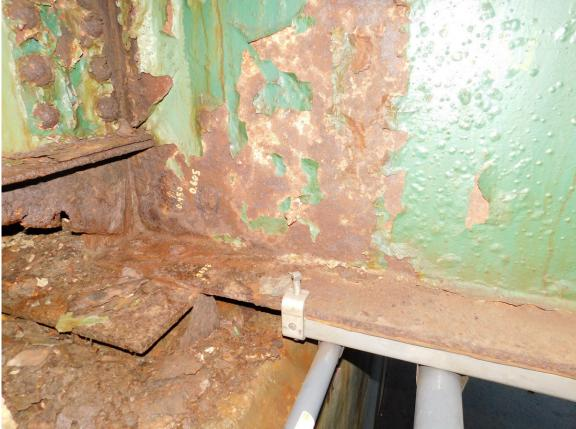
93 N Approach Span, Severe Corrosion on Lower Web and Flange at Stringer 4 & Perforated Gusset Plate at North Abut
