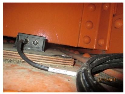
Photo E40 Inclinometer Unit. The span inclinometer was moved several times under the direction of the Engineer during its commissioning without success. The function of the inclinometer has now been disabled. The multi-turn span height resolvers, one in each tower, are presently being used in place of the inclinometers. The bridge presently has no secondary or backup means of skew detection.
