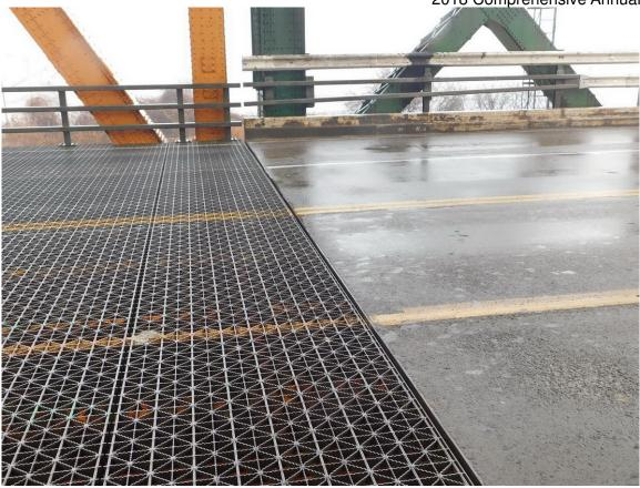
305 Open Gap Expansion Joint @ South Tower & Lift Span Decks, looking East
