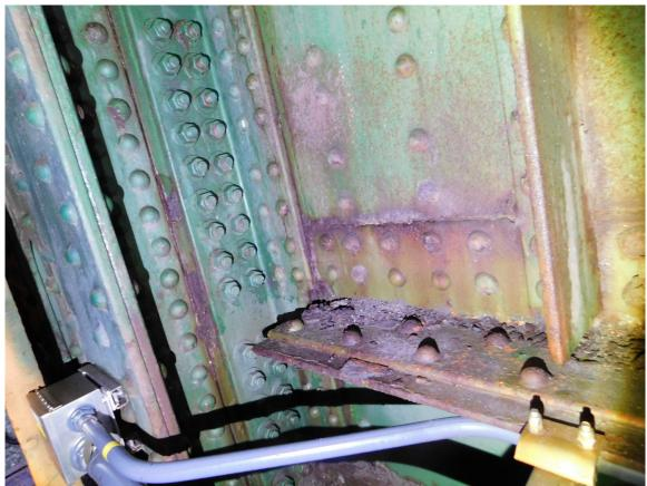
170 North Tower, Rust Stains with Local Light-Medium Rust Jacking at Bottom West Section of Front Floor Beam Page A2 [85] of A2 [169]
