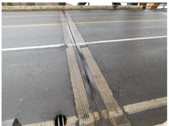
300 Compression Seal Expansion Joint at North Approach & North Tower Spans, looking East Page A2 [150] of A2 [169]
