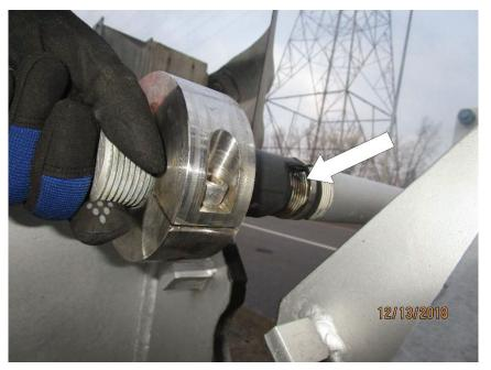
Photo M37 North Barrier Gate. The neoprene insulator (arrow) at the end of the arm is deteriorated.
