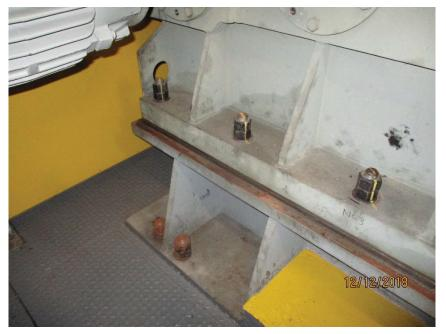
Photo M13 North Span Drive Reducer. The reducer mounting bolts and support anchor bolts are unpainted.
