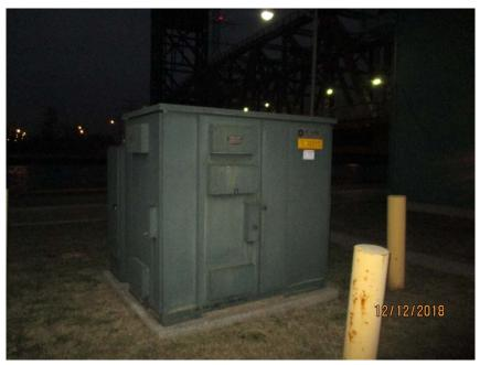
Photo E2 1,000KVA Outdoor Pad Mounted Incoming Service Transformer/Unit Substation. Note the primary service to the transformer is 13.8kV from the local utility overhead supply and the secondary of the transformer serves the bridge at 575volt, 3-phase, 60 Hz.
