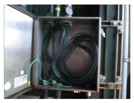
Photo E70 Typical Bonding. The raceway system bonding has been well installed and conforms to the CSA standard.
