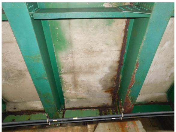
66 Wet Area on Central North End of North Approach Span Soffit
