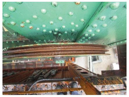
Photo M23 SW Auxiliary Counterweight Ropes. The counterweight ropes and sheave are devoid of lubricant.
