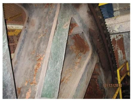
Photo M24 SW-OB Counterweight Sheave. There is paint deterioration and light corrosion on the sheave.
