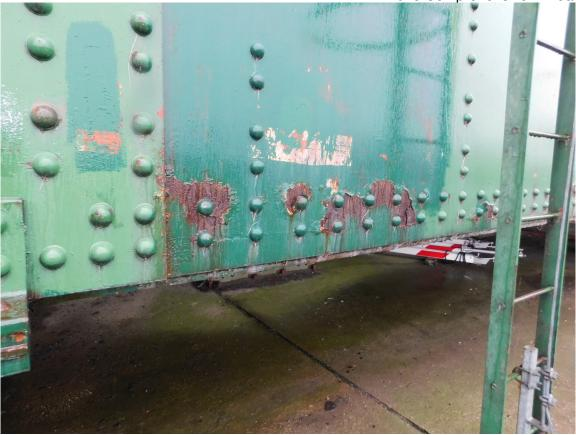
155 South Tower, Local Peeled Paint with Light Surface Rust on Bottom South Section of East Jacking Girder
