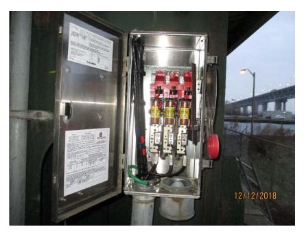
Photo E72 Existing Mobile Generator Disconnect Switch. The disconnect switch and generator receptacle are located at the foot of each tower. They have never been used but are capable of hooking up a mobile generator to operate the auxiliary drive motor in the respective tower.
