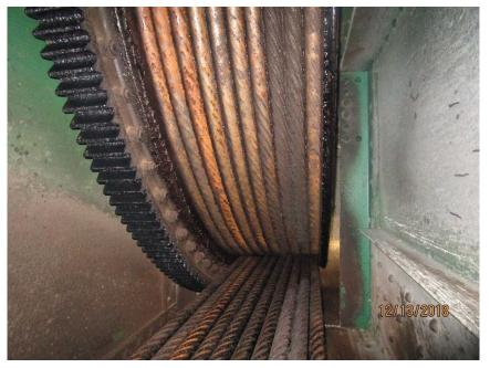
Photo M25 NE-OB Counterweight Sheave. The counterweight grooves have many sections that are devoid of lubricant and exhibit surface corrosion.
