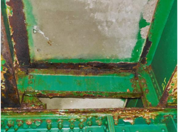
119 South Tower Span, Heavy Wet with Isolated Light Stained Crack at SE Corner of Deck Soffit
