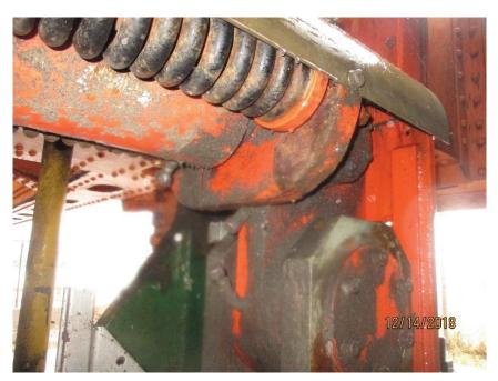
Photo M32 SE Span Lock, Spring Assembly. The springs and bolts have moderate corrosion.
