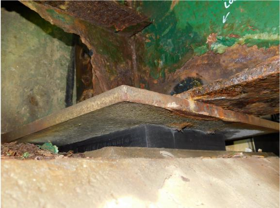
21 Typical Laminated Bearing & Oversized Shoe Plate at Abutments, Stringer 8 at South Abutment Shown
