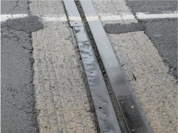
303 Deformed & Abrasion Marks on Joint Steel Angle @ Expansion Joint @ North Approach & North Tower Span
