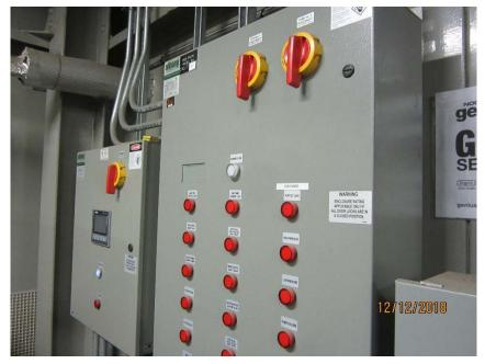
Photo E7 Generator Fuel Pump System. This pump system allows automatic refuelling of the day tank from the main tank located within the control house compounded area.
