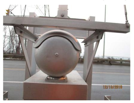
Photo E54 Typical Gong. Gongs were generally found to be in like new condition at the time of the inspection.
