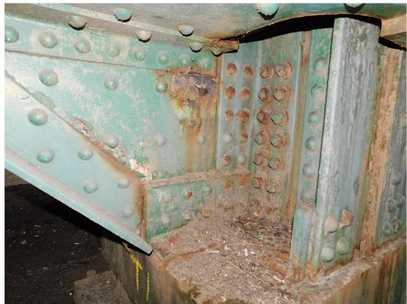
176 Typical Light Rust with Local Light-Medium Corrosion at Bottom of Tower Column, NE Column at S Tower Shown Page A2 [88] of A2 [169]
