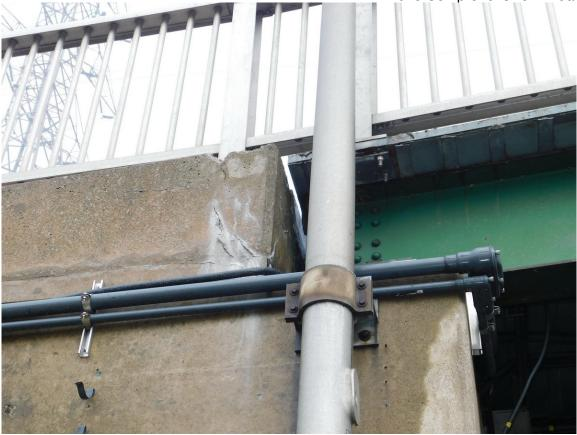
37 Local Minor Spalled and Stained Cracks at Top South Corner of Northwest Wingwall
