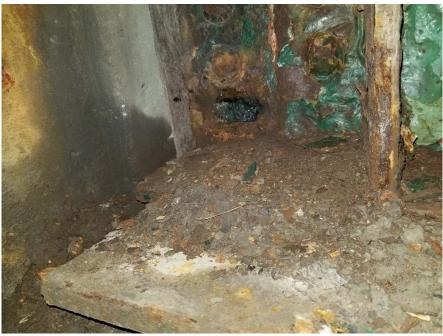
Girder 4S at the abutment wall - Severe corrosion
