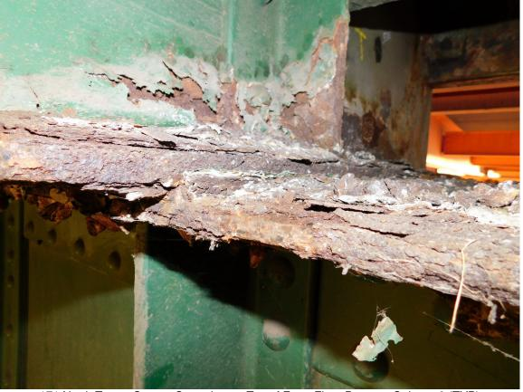
171 North Tower, Severe Corrosion on Top of Front Floor Beam at Stringer 8 (TYP)
