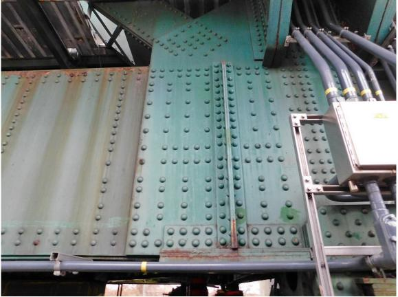
159 South Tower, Local Light Surface Rust on South End of West Jacking Girder
