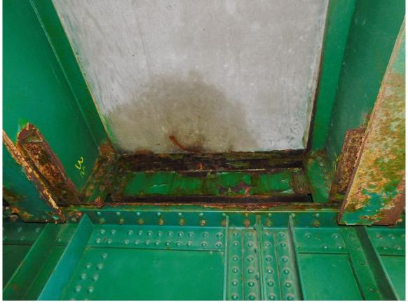
55 Typical Wet Area on North End of South Approach Span Soffit, Section between Stringers 2&3 Shown
