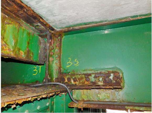
83 S Approach Span, Wet with Heavy Corrosion on Stringers & Diaphragm at North End of Span, Stringer 3 Shown
