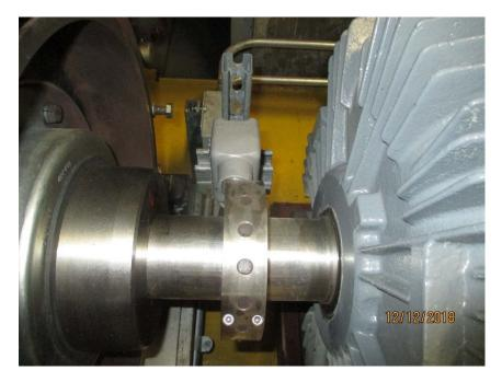
Photo E34 Typical Speed Switch Sensor. The speed switch sensor and pulse wrap have been installed between the motor and machinery brake for overspeed protection. The units are in good condition and the speed switch is operating as intended.
