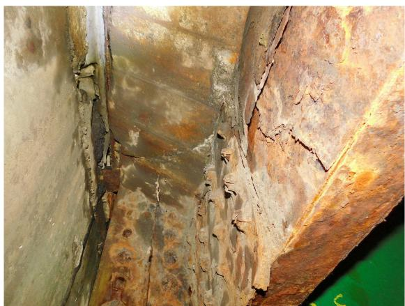
82 S Approach Span, Typical Severe Corrosion on Back Face of Diaphragm at South Abutment, Stringers 7&8 Shown Page A2 [41] of A2 [169]
