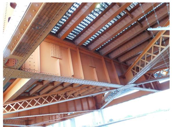
254 Intermediate Floor Beam A12-B12 and Stringers in Bay 13 of Lift Span, looking Southwest (TYP) Page A2 [127] of A2 [169]
