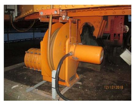
Photo E62 South Cable Reel. Note the south cable reel is in as-new condition, it provides power and control for electrical equipment on the movable span.
