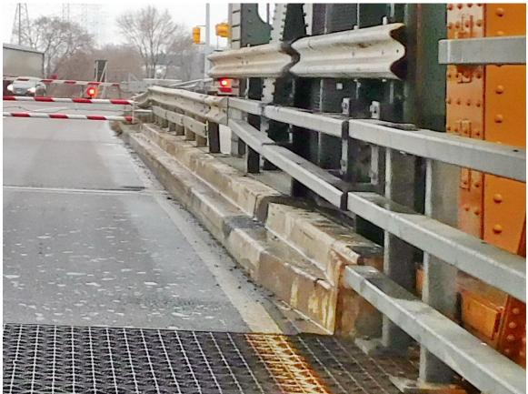
324 Typical Bent Steel Plate on South Tower & South Approach, looking South Page A2 [162] of A2 [169]
