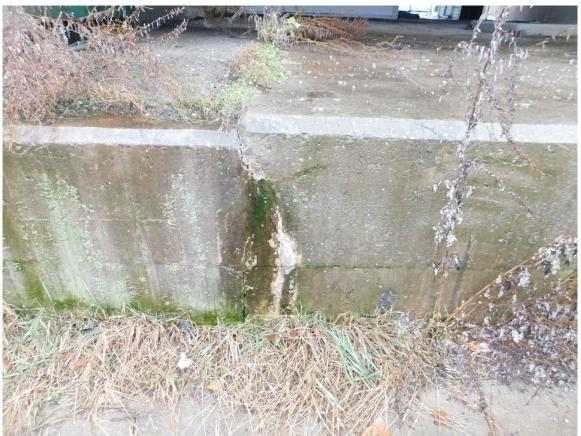
206 Wide Crack with Leakage at Construction Joint in North Concrete Pier (TYP) Page A2 [103] of A2 [169]
