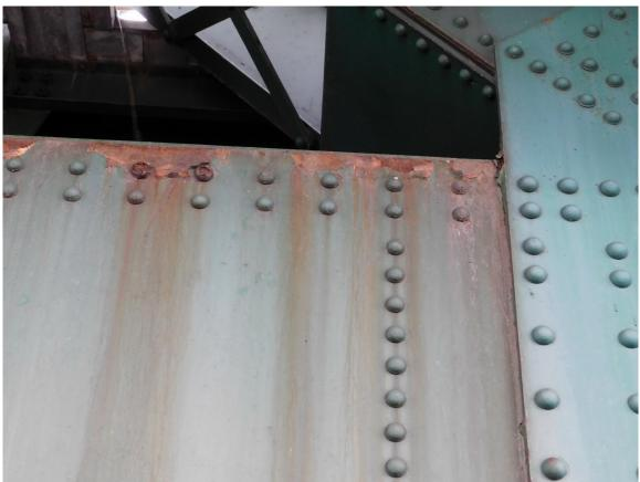
158 South Tower, Local Light Rust on top South Corner of West Jacking Girder Page A2 [79] of A2 [169]
