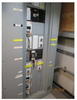
Photo E10 Main Switchboard No.2. This is the main distribution switchboard for the bridge electrical system. Note the yellow tapes and padlocks on the breakers. Some of the breakers are no longer in service and should be properly labeled as spare breakers and wires to the spare breakers removed.
