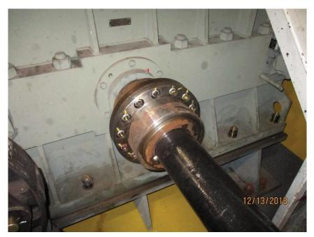
Photo M4 Coupling C2-NW. There is light corrosion on the hubs and sleeves. Corrosion was noted at all C1 and C2 couplings.
