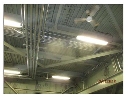
Photo E73 General Lighting and Smoke Detectors (South Tower Shown). The space lighting and fire system equipment have been adequately installed to provide a safe work place for inspection, maintenance and troubleshooting in the tower machinery spaces.
