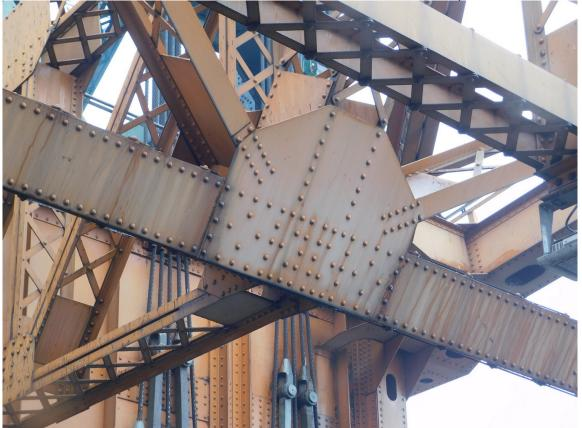
281 Typical Rust Stains & Light Corrosion on Portal Strut & Bracing, North Portal Shown
