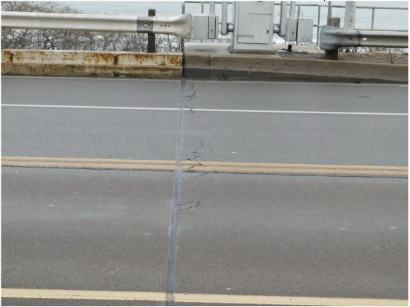
297 South Abutment Joint, Pattern Unsealed Cracks on Approach Asphalt at Joint, looking East
