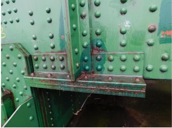
157 South Tower, Local Rust Jacking at Jacking Pad Plate at Bottom SE Section of East Jacking Girder
