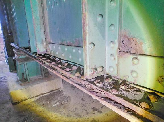
165 North Tower, Local Light-Medium Corrosion on Bottom East Section of Rear Floor Beam
