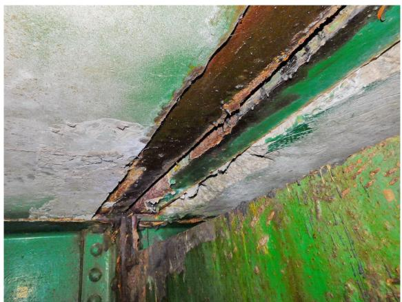
58 Local Spall on Soffit Adjacent to Expansion Joint between South Approach & South Tower Spans near Stringer 6 (TYP) Page A2 [29] of A2 [169]
