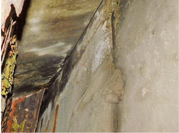
17 South Ballast Wall, Large Patch & Local Spall behind Diaphragm between Stringer 4&5
