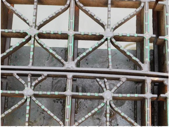
231 Cracked Grating at Central Section of Lift Span, Stringer 7 south of Floor Beam A7-B7
