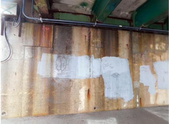
13 North Abutment, Heavy wet-Rust Stains, Medium-Wide Vertical Crack, and Local Delam on West Section of Wall
