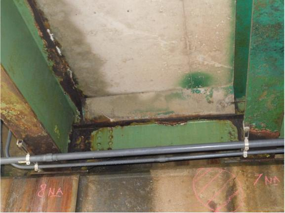
65 Heavy Wet Area on Soffit adjacent to West Stringer 8 at North Abutment (TYP)
