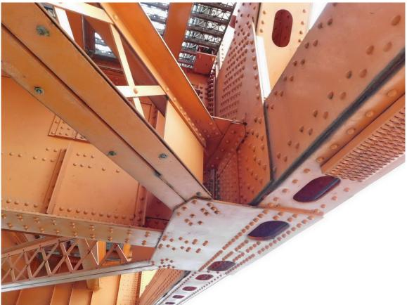
258 Typical Truss Bottom Chord Connection @ Main Floor Beam, Node Point A2 Shown Page A2 [129] of A2 [169]
