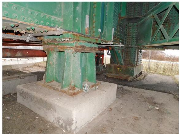
200 Typical Interior Steel Pedestal Bearing under East Section of Front Floor Beam, South Tower looking East Shown Page A2 [100] of A2 [169]
