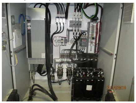
Photo E22 Typical VFD Drive System. The 200HP Danfoss VFD drive, 18 poles transformer and rectifier have been well installed inside the drive enclosure.
