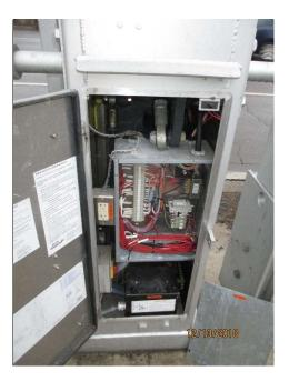
Photo E55 Typical Traffic Gate Enclosure. The equipment inside the gate enclosure was found to be in as-new condition.
