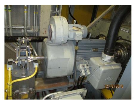
Photo E25 Northeast Motor Blower Nameplate. Similar to the last inspection, the blower nameplate was not affixed to the motor at the time of inspection.
