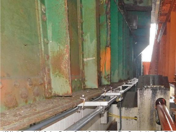
169 North Tower, Light Surface Rust on Central Section of Front Floor Beam looking East (TYP)
