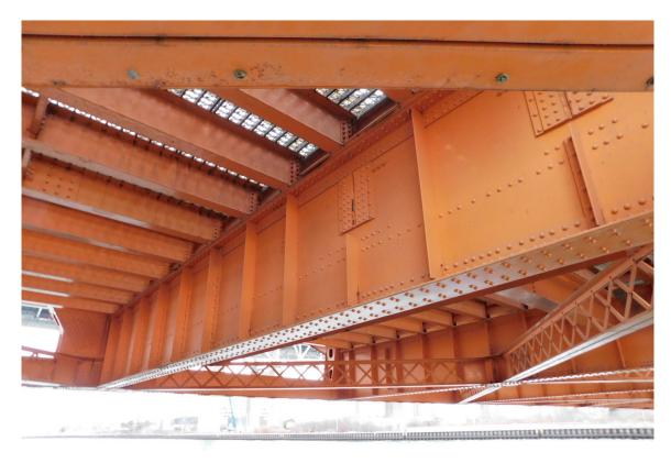
252 Typical Main Steel Floor Beam on underside of Lift Span, Beam A3-B3 looking West Shown Page A2 [126] of A2 [169]
