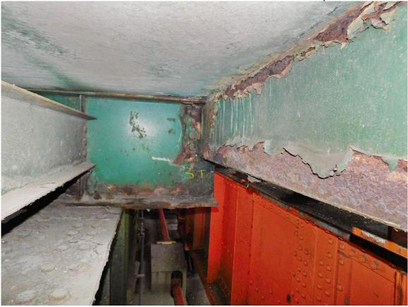
125 South Tower Span, Typical Heavy Corrosion on North Edge Diaphragm at Joint with Lift Span
