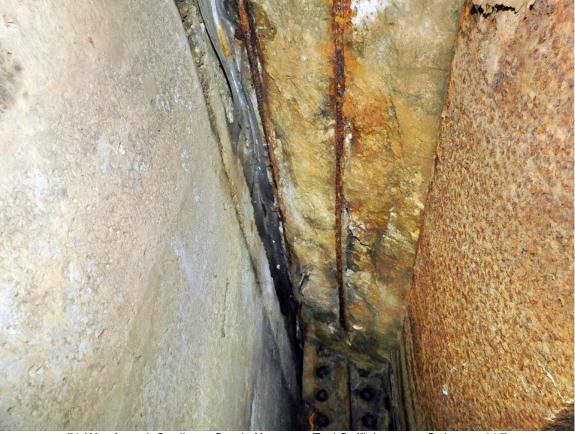
53 Wet Area & Spalls on South Abutment End Soffit between Stringers 6&7
