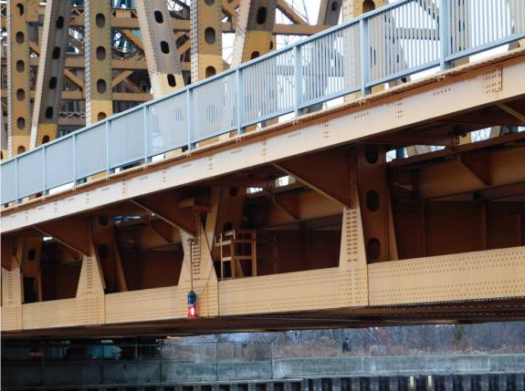
261 West Truss Bottom Chord Connections at Central Section of Lift Span, Node Points B6 to B9 looking North
