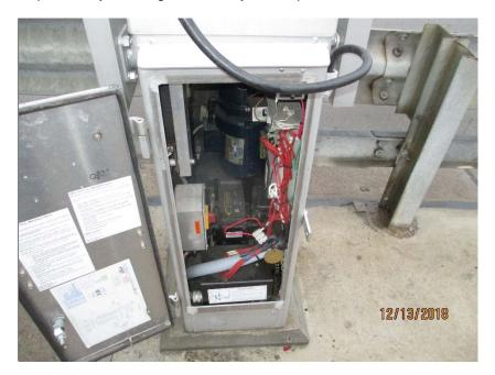
Photo E58 Typical Pedestrian Gate Enclosure. Note that the length of wires inside the gate are excessive and an improper wire splicing is used with unsecured terminal blocks at the time of inspection. Otherwise the gate is in as-new condition.
