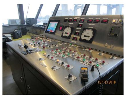
Photo E14 Main Control Console. New upgraded console top is provided during the recent motor and drive replacement project. The console is in excellent condition.
