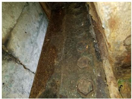
Girder web by abutment wall. Full height of the web is corroded/delaminated. This degree of corrosion is typical for all girders.
