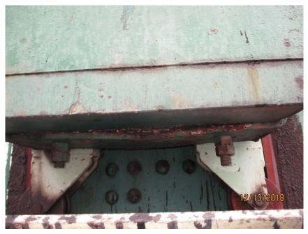
Photo M26 NE Auxiliary Counterweight. There is corrosion on the bottom support plate and bolts.
