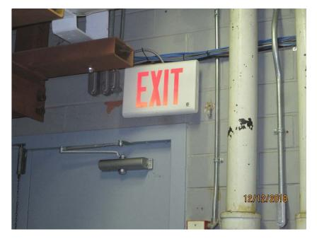
Photo E71 Exit Light. Typically, all exit lights are in working order and conform to code requirements.
