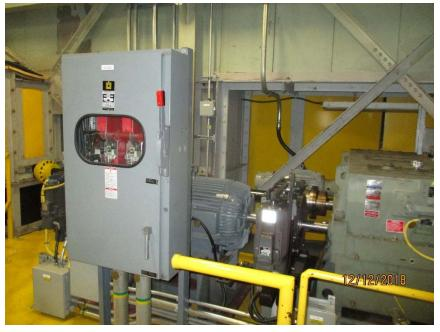
Photo E23 Typical Drive Motor Disconnect Switches. The drive motor disconnect switch was part of the original installation and have been reused to serve the new motors.
