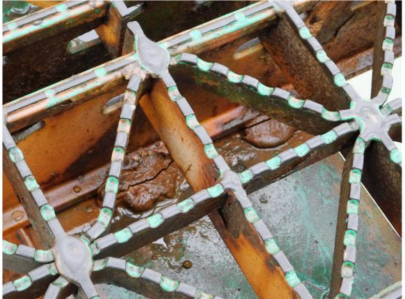
235 Cracked Hold-down Weld @ Grating to Stringer 9 South of 4th Floor Beam from South (Beam A4-B4)
