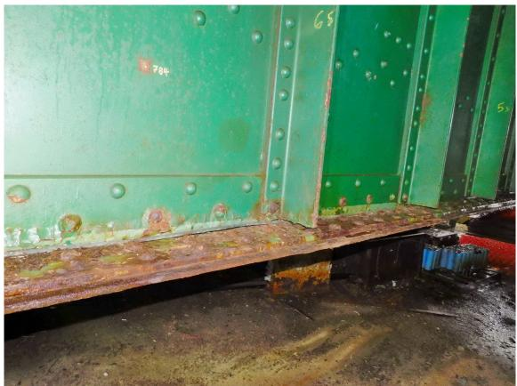
146 South Tower Span, Heavy Corrosion on Lower Section of Rear Floor Beam below Exp. Joint at North End of Span Page A2 [73] of A2 [169]
