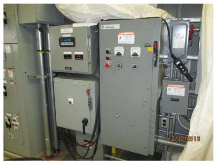
Photo E28 South Auxiliary Drive Controller and Span Height Indication Panel. The auxiliary drive was relocated along with the MTS and emergency power panelboard. They are all in good serviceable condition. Note the white plastic sheet cover over the units which is an indication of the roof leak in the area.
