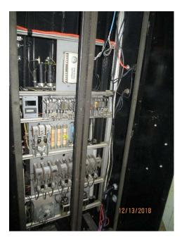
Photo E42 Typical Elevator Control Cabinet. The elevator control is in working and fair condition but reportedly requires periodic maintenance.
