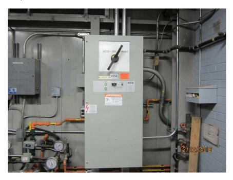
Photo E6 Automatic Transfer Switch (ATS). This ATS is used to transfer power from utility to auxiliary generator power. The ATS is configured to automatically start the auxiliary generator in the event of a power failure. The ATS is in good serviceable condition.
