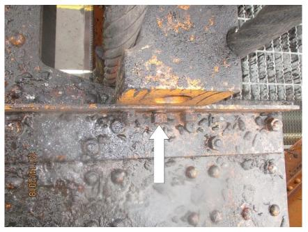
Photo M21 NW-OB Main Lift Girder Splay Casting. The middle nut is not fully seated at this location (arrow). Also note the light fretting at the rope/splay interface.
