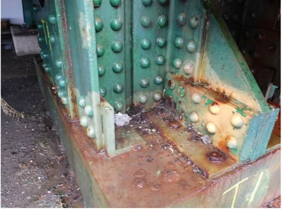
189 South Tower, Local Light Surface Rust on Top Surface of NE Column Anchorage Assembly (TYP)
