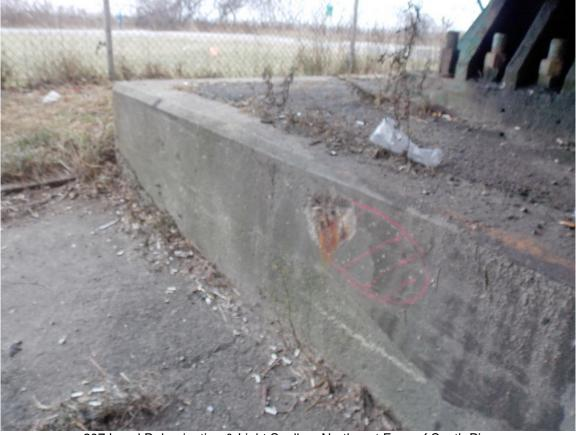
207 Local Delamination & Light Spall on Northeast Face of South Pier
