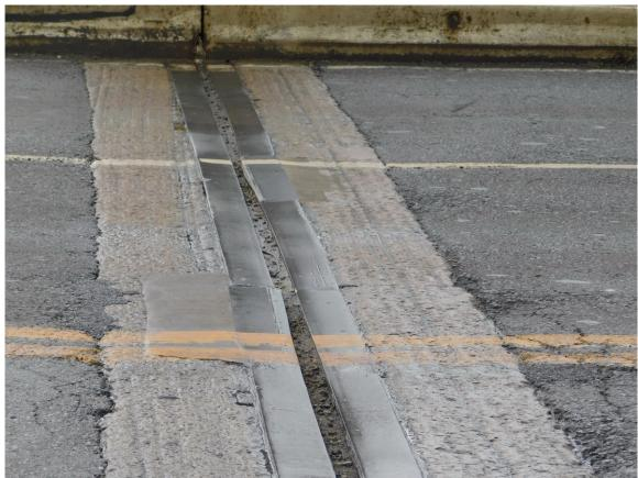
302 Typical Concrete-Asphalt Patches & Minor Spalls on End-Dams, Joint between North Approach & Tower Spans Page A2 [151] of A2 [169]
