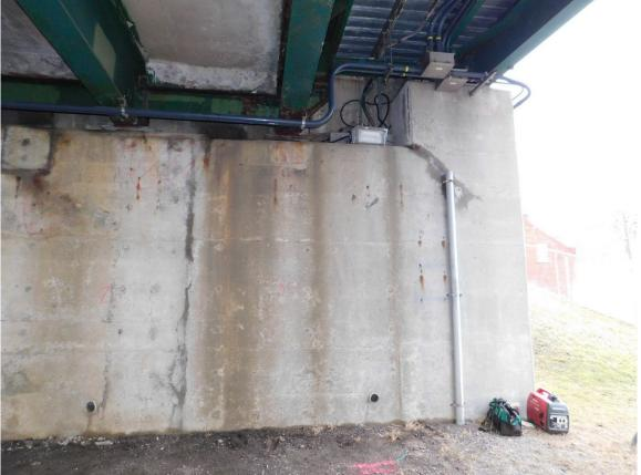
11 South Abutment, Stained Cracks & Local Delamination on Upper West Section of Wall
