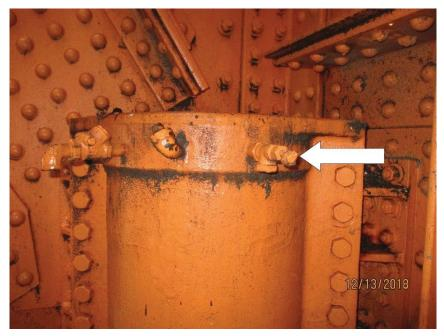
Photo M30 NW Span Air Buffer. The exhaust valve handle (arrow) is broken.
