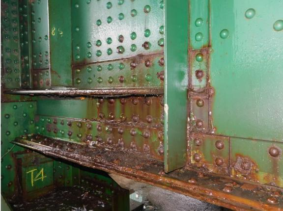
147 South Tower, Heavy Rust Stains on Bottom SW Section of Rear Floor Beam, looking West
