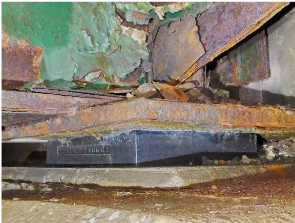
22 Laminated Bearing under Stringer 4 at South Abutment (TYP)
