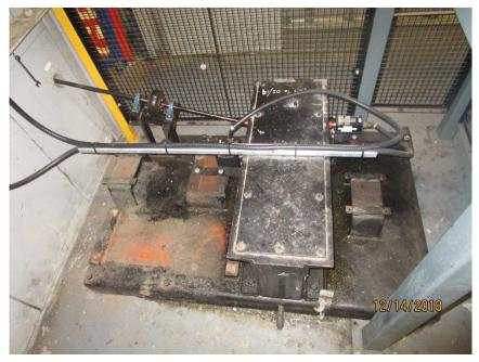
Photo M15 South Span Position Parallel Shaft Reducer. Note the light accumulation of oil around the reducer.
