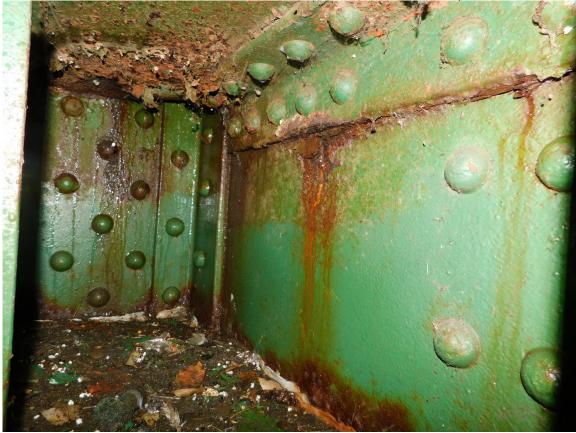
191 South Tower, Local Light Corrosion on interior Surface of T3 Anchorage Assembly
