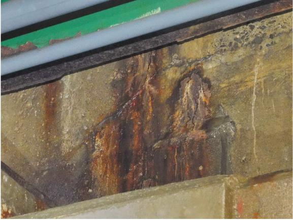
19 North Ballast Wall, Cracks with Heavy Rust Stains between Stringer 3&4
