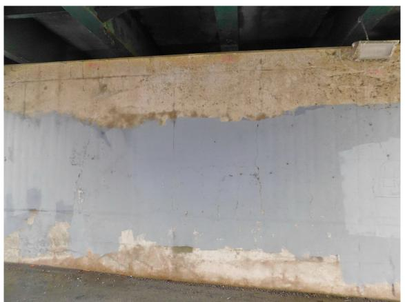
30 Typical Narrow-Medium Vertical Cracks on Curtain Wall, Central Section of North Wall Shown Page A2 [15] of A2 [169]
