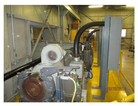
Photo E24 Typical Drive Machinery Arrangement. The span motors and motor brakes are in as-new condition. The machinery brakes were existing but have been provided with a new brake drum as part of the recent motor and drive replacement project.
