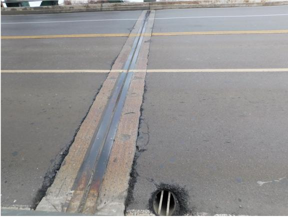
299 Compression Seal Expansion Joint at South Approach & South Tower Spans, looking East
