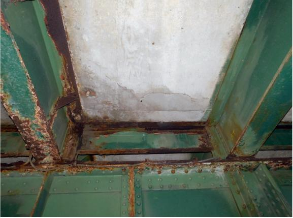
133 North Tower Span, Large Delamination Area at North End of Soffit between Stringers 3&4
