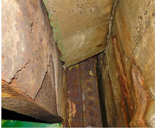
95 N Approach Span, Typical Severe Corrosion on Back Face of Diaphragm at North Abutment, Stringers 3&4 Shown
