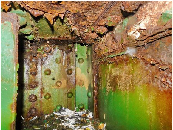
192 South Tower, Local Medium-Severe Corrosion on Interior T4 Anchorage Assembly Page A2 [96] of A2 [169]
