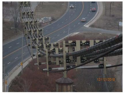
Photo E64 Typical Aerial Cable Spacer (East Shown). Note the aerial cable spacers were in as-new condition at the time of the inspection.
