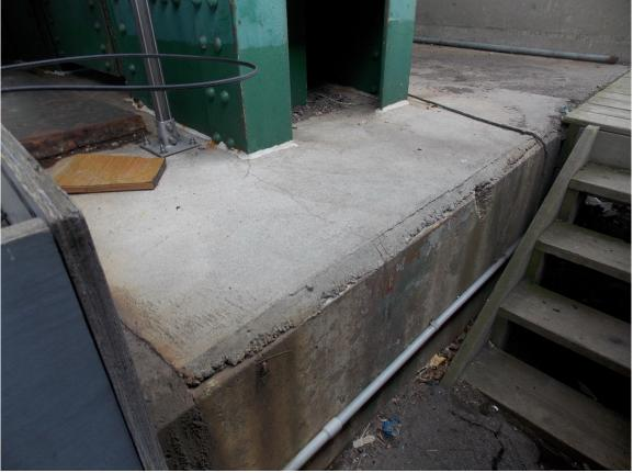
205 South Tower, Medium Crack on Resurfaced Concrete @ SW Column
