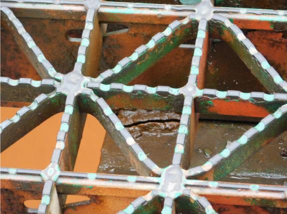
237 Cracked Hold-down Weld @ Grating to Stringer 9 in North Section of 4th Bay from South near Floor Beam A5-B5
