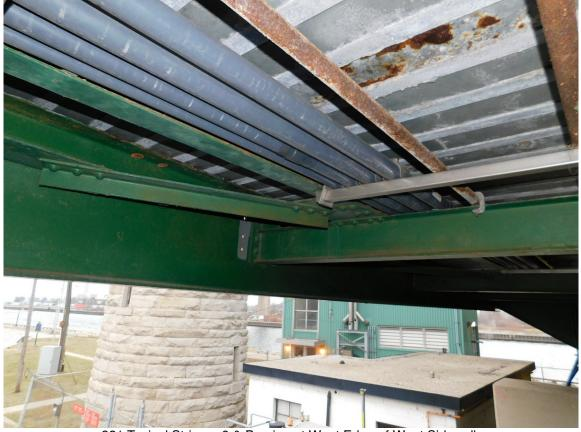
321 Typical Stringer 9 & Bracing at West Edge of West Sidewalk
