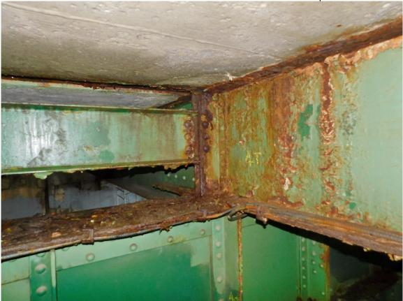
135 North Tower Span, Heavy Wet & Severe Corrosion on Stringer 4 at North End below Exp Joint with N Approach Span
