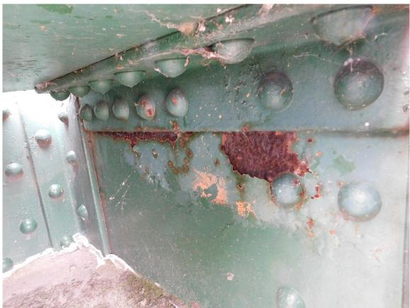
198 North Tower, Local Light Corrosion on Interior Surface of Anchor Assembly @ T1 Page A2 [99] of A2 [169]
