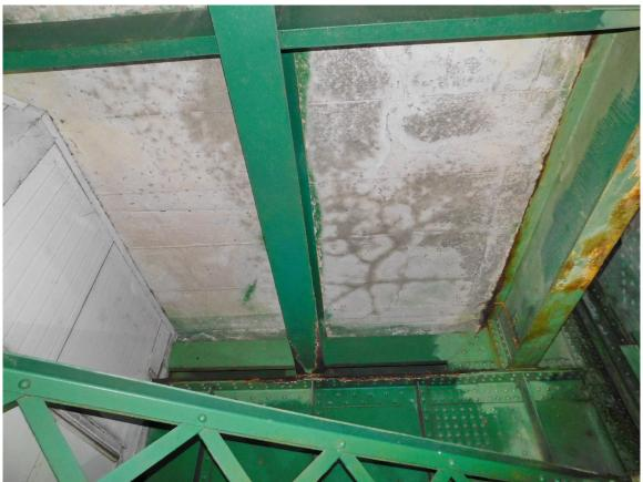
130 North Tower Span, Large Wet Area on SW Section of Soffit looking South Page A2 [65] of A2 [169]
