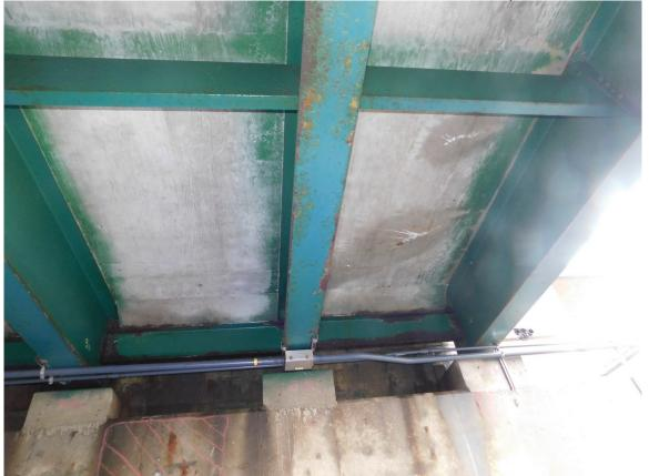
67 Cracks with Wet and Efflorescent Stains on NE Section of North Approach Span Soffit
