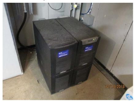
Photo E12 New UPS and UPS Distribution Panel. The UPS and its distribution panel is located next to the CP-2 and is in as new condition. Note the different type of laminated labels on the UPS distribution panel that are used to indicate the purposes of the breakers.
