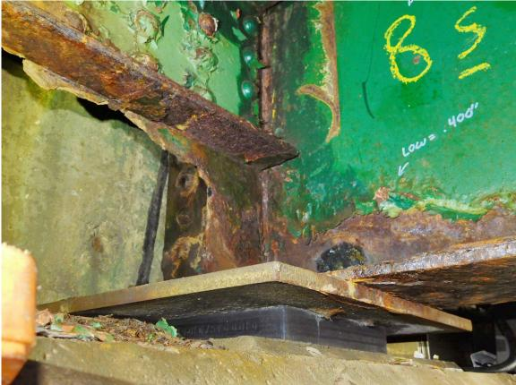
81 S Approach Span, Perforated Gusset & Severe Corrosion on Bottom Web & Flange at S Abutment End of Stringer 8
