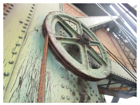
Photo M22 NW Auxiliary Counterweight Ropes. The auxiliary ropes and sheave have built up old lubricant.
