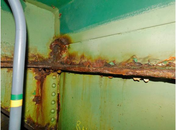
325 Typical Local Severe Corrosion on lower Section of Bent Curb Plate atop Stringer 8, North Abutment End Shown
