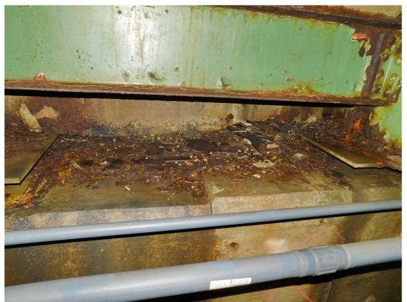
16 Typical Debris and Wet Area on Abutment Bearing Seat, North Abutment between Stringer 6&7 Shown Page A2 [8] of A2 [169]
