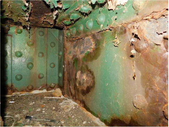
199 North Tower, Local Medium-Severe Corrosion on Interior Surface of Anchor Assembly @ T2 NW Rear Column
