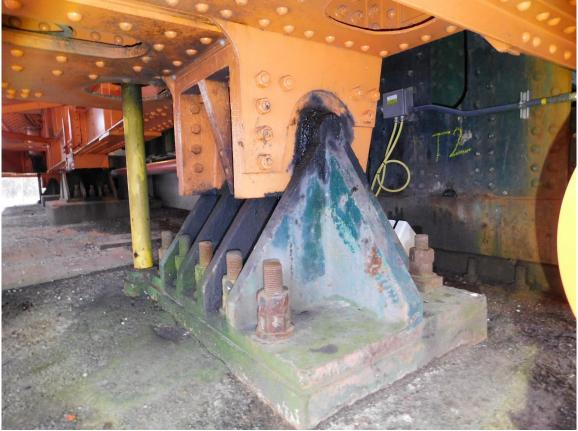
289 Steel Saddle Bearing @ Southwest Corner of Lift Span, looking East
