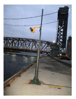
Photo E50 Small Craft Navigation Light. The small craft navigation lights one light has been installed on each side of the canal. Note the minor corrosion on the light mounting post.
