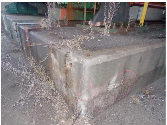
208 Large Delamination & Local Severe Spalls on SW Corner of Pier
