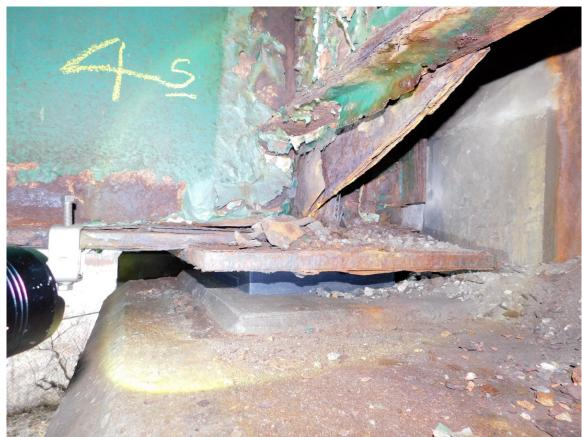
80 S Approach Span, Local Severe Corrosion on Bottom of Stringer 4, Gusset Plate, & Diaphragm at South Abutment Page A2 [40] of A2 [169]
