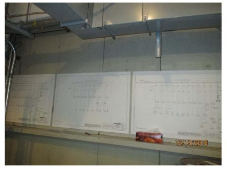
Photo E1 One Line Diagrams in Electrical Room. Note that the "As Built" one-line diagrams were updated as part of the recent motor and drive replacement project and are posted throughout the bridge.
