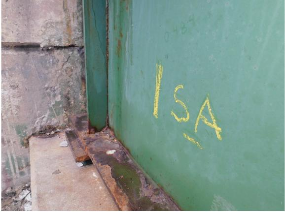
77 Local Peeled Paint showing Light Rust Surface Rust on Exterior Face at South End of Stringer 1
