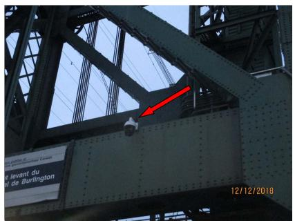
Photo E68 CCTV System. The CCTV cameras are strategically located throughout the bridge to monitor the roadway approaches, waterway approaches and main access areas to the bridge. The operation monitors all location from the operator's room via a CCTV monitor. The camera installation was found to provide good visual information and had been well installed.
