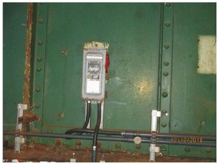
Photo E44 Typical Span Lock Motor Disconnect Switch (North Disconnect Switch Shown). The disconnect switch is rated NEMA 3R and exhibits severe corrosion on the enclosure and on disconnect handle.
