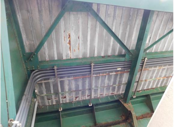
59 Local Light Surface Rust on Steel Decking under Sidewalk at NW Section of South Approach Span
