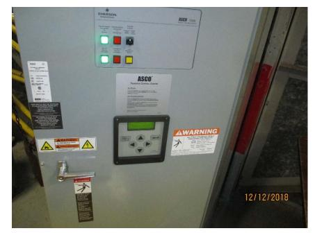
Photo E33 New Aerial Cable ATS in North Tower. The ATS was installed during the recent motor and drive replacement project.. It is used to automatically switch the aerial cable power feed between the east and west aerial installation. The ATS has been well installed and is in excellent operational condition.
