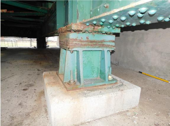
201 Typical Interior Steel Pedestal Bearing under East Section of Rear Floor Beam, North Tower looking West Shown
