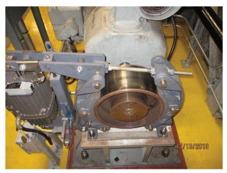
Photo M2 Motor Brake-NW. General view of a typical motor brake assembly. The brake wheel hubs and fasteners are unpainted.
