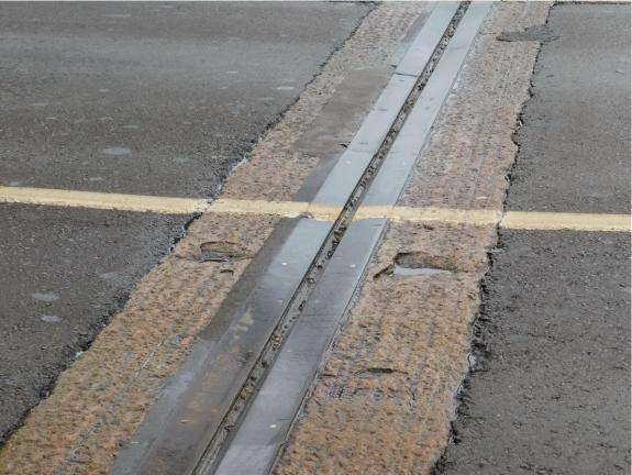
301 Typical Rough & Local Spalls on Concrete End-dams for Compression Seal Expansion Joint, South Joint Shown
