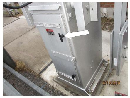
Photo M33 North Oncoming Warning Gate. The front door top latch (arrow) cannot be unlocked for inspection.
