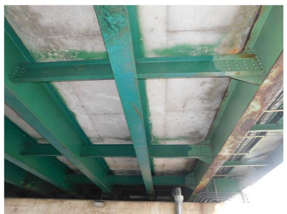
64 Large Wet Areas on West Section of North Approach Span Soffit, looking South Page A2 [32] of A2 [169]
