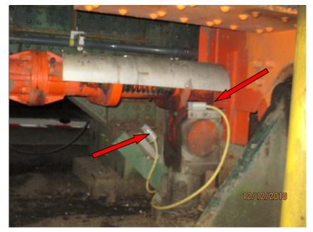
Photo E45 Typical Span Lock Limit Switches at the Lock Bar. These limit switches were installed as part of the recent motor and drive replacement project and were found to be in good physical and operational condition.
