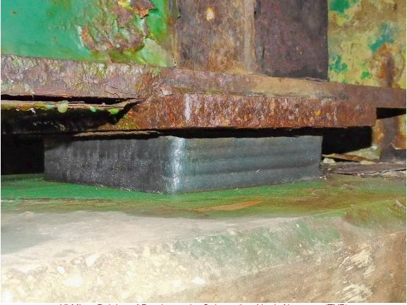
25 Minor Bulging of Bearing under Stringer 2 at North Abutment (TYP)
