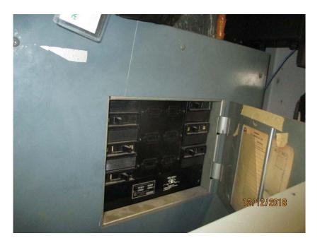
Photo E35 Typical Tower Heater Distribution Panel. This panel was part of the existing installation and was found to be in good operating condition at the time of the inspection.
