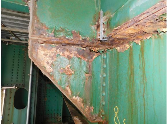
89 S Approach Span, Severe Corrosion on Top Flange of Stringer 8 at Central North Section of Span
