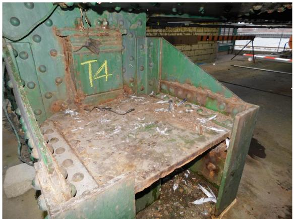
190 South Tower, Local Corrosion on Top Exposed Surface of Anchor Assembly at T4 Page A2 [95] of A2 [169]
