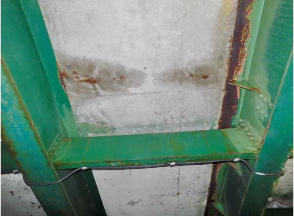
131 North Tower Span, Stained Crack with Wet and Rust Stains on North Central Section of Soffit between Stringers 3&4
