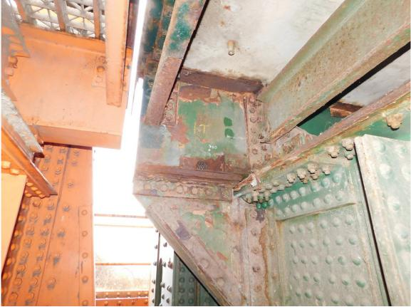
123 South Tower Span, Heavy Corrosion at North End Section of Stringer 1 (TYP)
