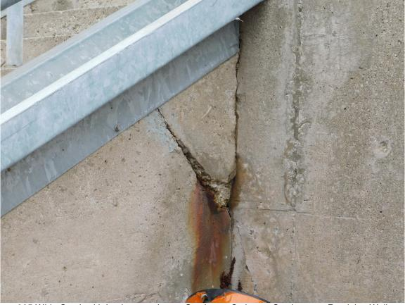
335 Wide Crack with Leakage on Lower Southwest Staircase Section near Retaining Wall
