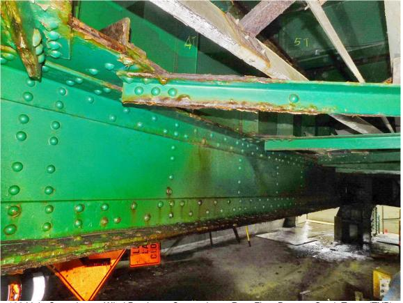
183 Light Corrosion on Wind Bracing at Connection to Rear Floor Beam at South Tower (TYP)
