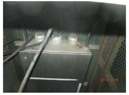
Photo E37 Abandoned Cables (typical). Abandoned cables have not been completely removed from the junction boxes/raceway system but left in place.
