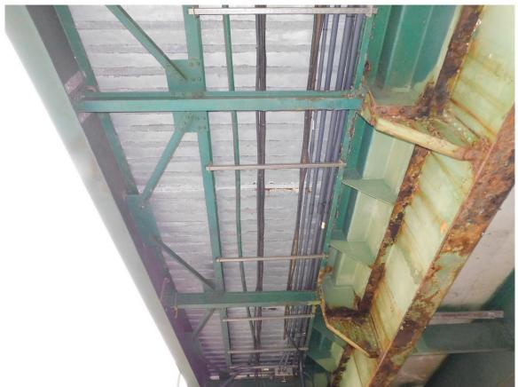
76 Local Light Rust on Steel Decking under West Sidewalk at North Approach Span, looking North Page A2 [38] of A2 [169]
