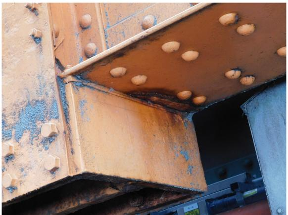
268 Local Light Surface Rust on Bottom of North Floor Beam A13-B 13 @ Centering Shoe Page A2 [134] of A2 [169]
