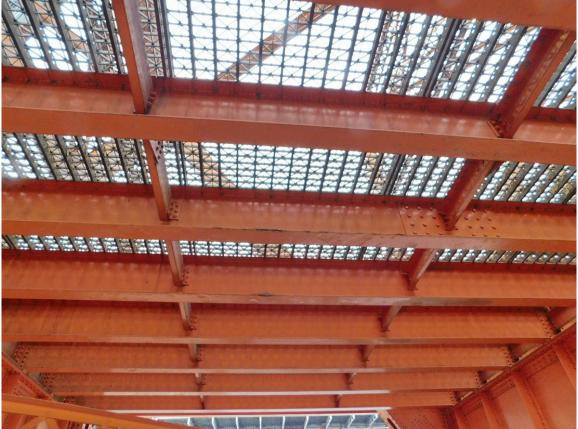
249 Steel Stringers in Bay 2 below Deck Grating in Lift Span, looking West (TYP)
