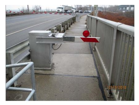
Photo E57 Typical Pedestrian Gate. The pedestrian gate is used to stop pedestrian traffic during the bridge operation. The Pedestrian gates were found to be in as-new condition. Note that the pedestrian gate and signal control are not included in the traffic control sequence. The operator is able to stop pedestrian traffic independently of bridge control system operation.
