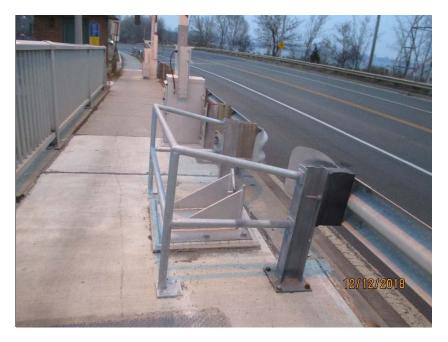
Photo E60 Barrier Gate Receiver. Note the newly installed permanent railing has been provided to keep pedestrian traffic from the barrier receiver pocket.
