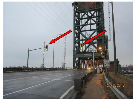
Photo E51 Traffic Signals (South Approach). Typically, traffic signals are in good physical and operational condition. The light bulbs are LED which extend the life of the bulbs.
