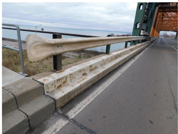
308 Typical Steel Beam Guiderail on Approach Span, East Guiderail on North Approach looking South Shown Page A2 [154] of A2 [169]
