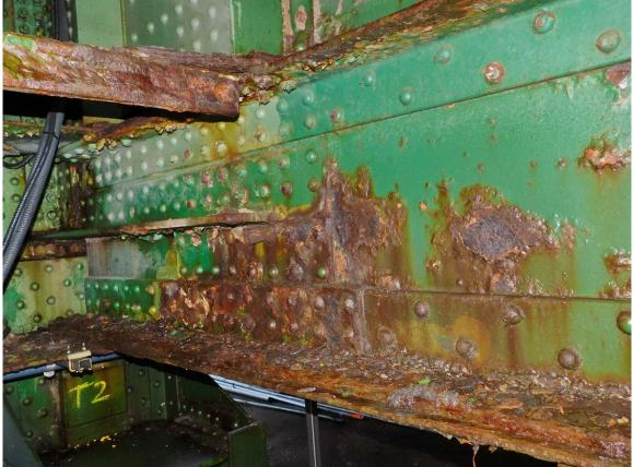
167 North Tower, Large Severe Corrosion Area on lower South Face of Rear Floor Beam below Stringers 7&8
