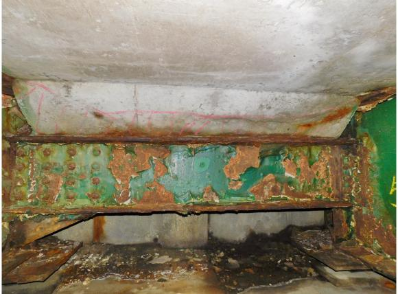
51 Heavy Wet with Local Severe Delamination at South Abutment End of Soffit between Stringers 4&5 (TYP)
