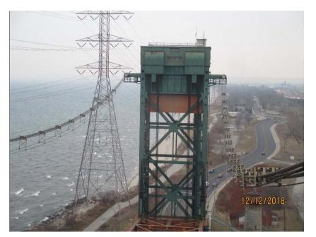
Photo E63 Typical New Aerial Cables. The aerial cables were replaced during the recent motor and drive replacement project and was found to be in good condition.
