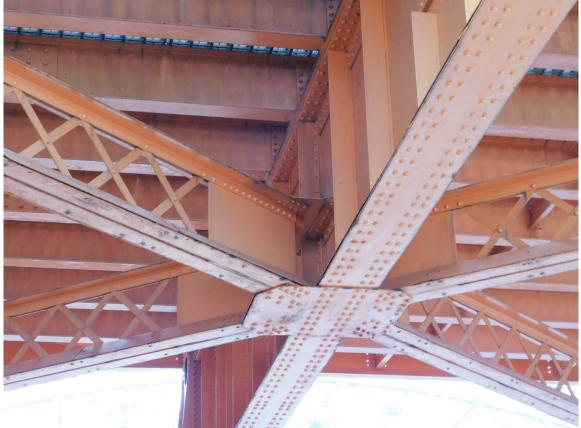
263 Typical Lateral Bracing at Intermediate Floor Beam, Beam A2-B2 looking West Shown
