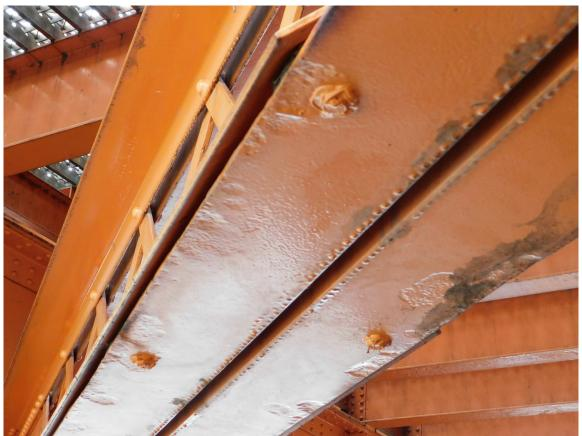
274 Painted-over Pitted Bottom Surface of Lateral Bracing in Bay 12 (TYP) Page A2 [137] of A2 [169]
