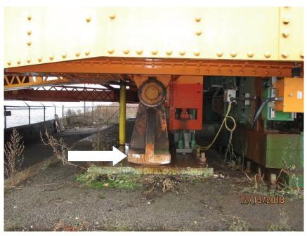
Photo M28 NW Live Load Rocker. The live load rocker was unable to be freely rotated. NE Live Load Rocker was similar.
