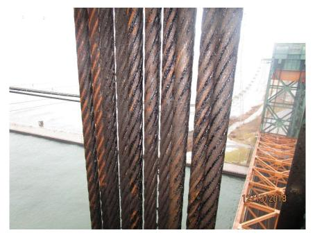
Photo M19 NE-OB Counterweight Ropes. View of the section of the ropes that contact the sheave grooves. Note the surface corrosion due to inadequate lubricant.
