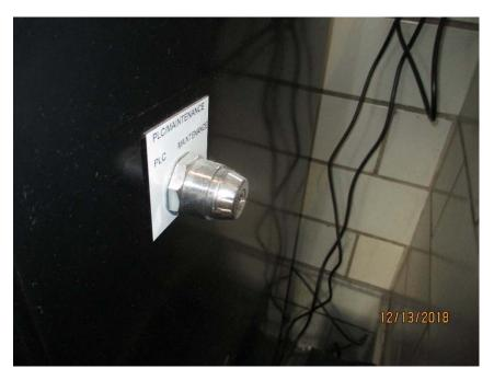
Photo E16 Traffic Control Bypass. A keyed selector switch for PLC and Maintenance select has been installed on the side of the console cabinet as part of the new control system. Note that relay mode for traffic control does not have any interlocks per the recent motor and drive replacement project design.
