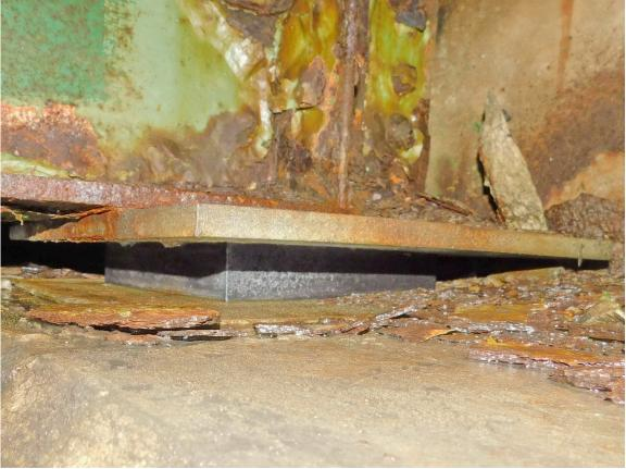
23 Laminated Bearing under Stringer 7 at North Abutment (TYP)
