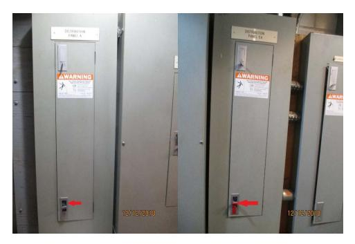
Photo E13 Broken Locks/levers on Panelboards. Note the indicated panel lock/levers were found to be broken on both Panel A and Panel EA inside the electrical room at the time of the inspection.
