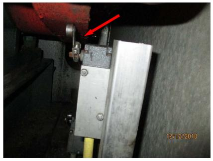
Photo E46 Typical Span Lock Limit Switches at the Center of Lock Machinery. A set of limit switches were installed at the center of the span lock rotation machinery. These limit switches were installed as part of the recent motor and drive replacement project and are now used in place of the original rotary cam limit switch installed to perform a similar function.
