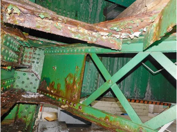
181 Typical Light Rust on Bracing Members at Connection to Tower Members, South Tower at SW Column Shown
