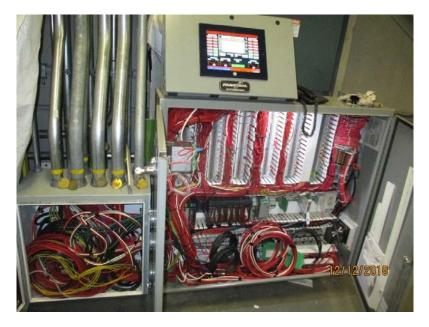
Photo E30 Inside of Pull Box and CP-3 Cabinet. Although the pull box was installed in addition to the control cabinet, both enclosures are over filled in accordance with code.
