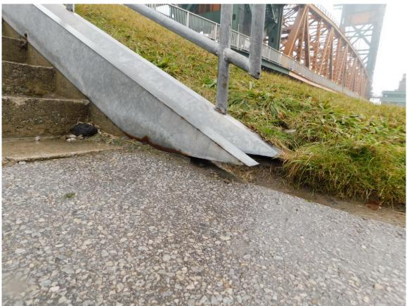
334 Puncture Hazard from Settled Walkway at bottom of Bike Rail at NW Stairs Page A2 [167] of A2 [169]
