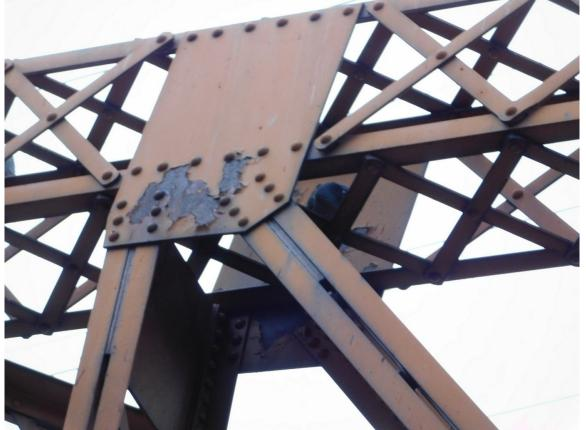
283 Peeled Coating & Light Corrosion on Gusset Plate @ South Portal Bracing (TYP)
