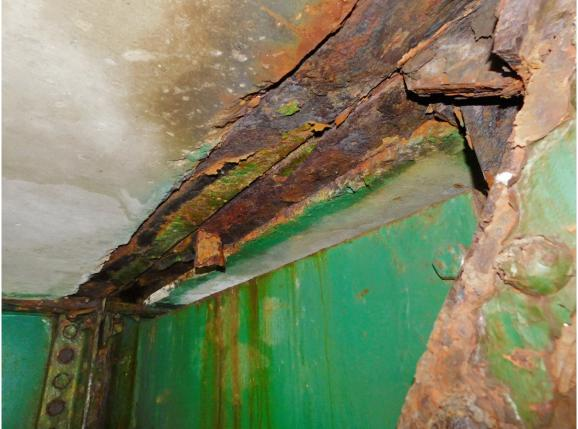
57 Typical Wet & Heavy Corrosion on Steel Angle at North End of South Span Soffit, Stringers 1&2 Section Shown
