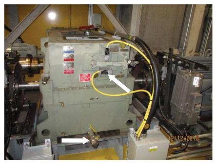
Photo M14 North Span Drive Reducer. There is evidence of a small oil leak at the north index spline lower limit switch mounting bracket (upper arrow) and the drain valve (lower arrow).
