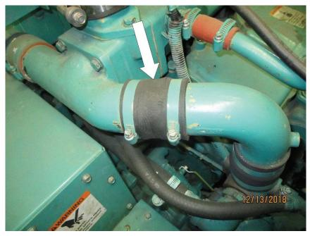
Photo M38 Main Generator. A coolant hose (arrow) exhibits dry rot and is cracked.
