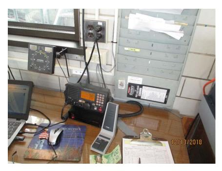
Photo E19 Wind Speed Indicator and Marine Radio. Both units were part of the bridge installation prior to the recent motor and drive replacement project and are in good serviceable condition.
