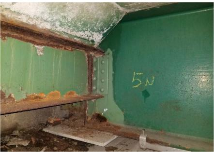
Example of a girder-to-diaphragm connection. Small patches of corrosion can be seen. The most severe locations were tested and compared against what was measured to be "nominal".
