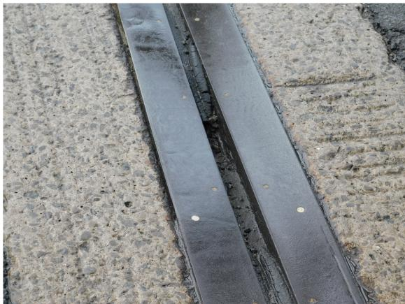
304 Loose Compression Seal in West Section of Expansion Joint between North Approach & North Tower Span Page A2 [152] of A2 [169]
