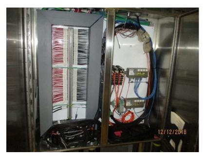
Photo E32 South Tower Aerial Cable Control Termination Box. The network switches and fiber patch boxes are also installed inside the termination box as indicated. Note the looped cables inside the box which are the spare conductors and communication cables. Their condition has not changed from the 2017 inspection.
