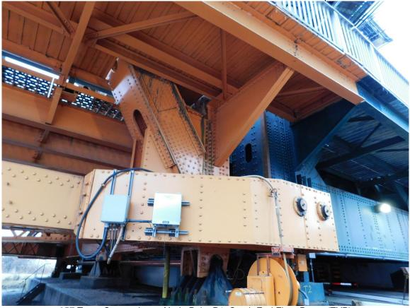
257 Truss Connection at Node Point B1, South End Floor Beam (TYP)
