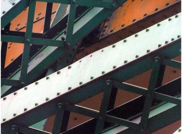
215 South Tower, Missing Rivets on Mid-Section of West Horizontal Member between Panel 5&6 West Face
