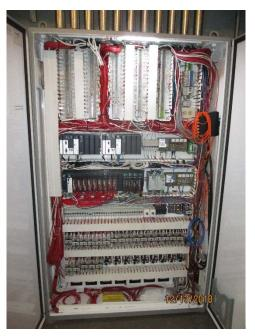
Photo E11 New CP-2 Control Panel. New free-standing control panel was installed as part of the recent bridge motor and drive replacement project. The redundant PLC system and control devices have been properly installed inside the panel. Note that the wireway cover cannot be mounted over the enclosure due to over filling of wires in the wireway in some area.
