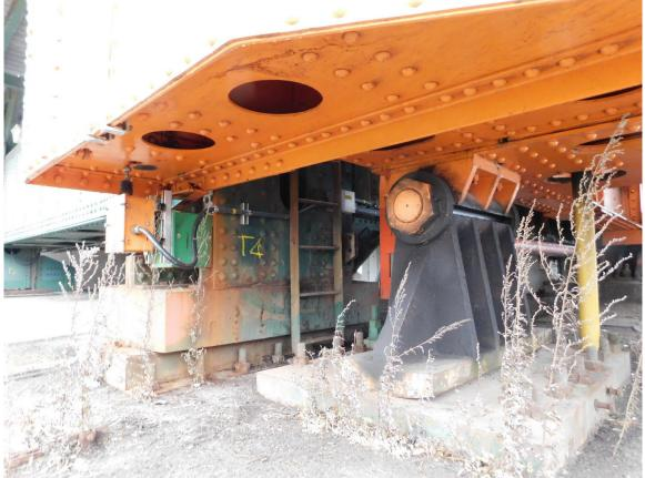
291 Steel Rocker Bearing @ Northwest Corner of Lift Span
