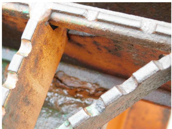
234 Cracked Hold-down Weld @ Grating to Stringer 8 South of 3rd Floor Beam from South (Beam A3-B3) Page A2 [117] of A2 [169]
