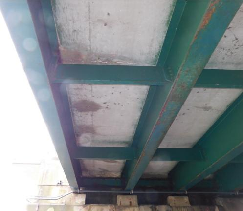
47 Large Wet with Stained Cracks and Local Severe Delamination on East Section of South Approach Soffit, looking S
