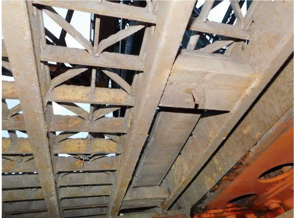
241 Wooden Blocks on Underside of Deck Grating at Central North End of Lift Span, between Stringers 6 & 7
