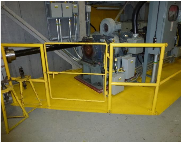
Photo 21: South tower yellow paint on bollards
