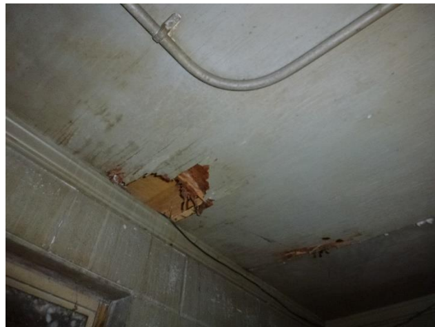
Photo 18: Gate house ceiling & wall LCM
