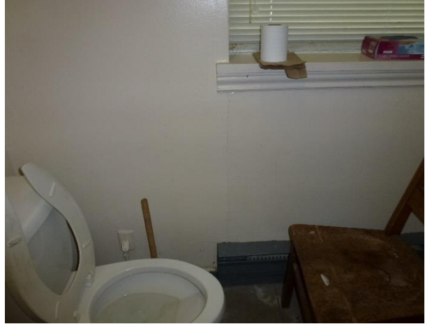
Photo 8: Old workshop ACM drywall joint compound
