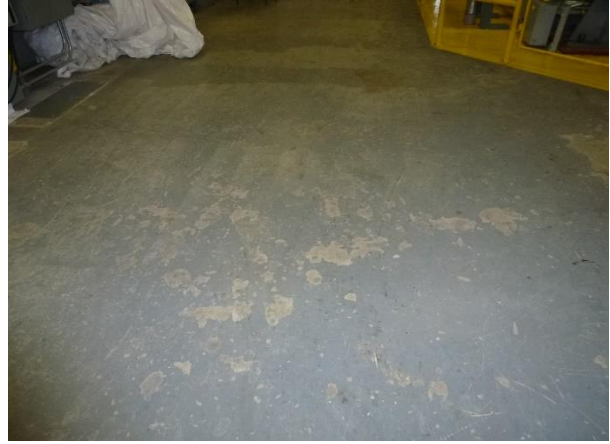
Photo 20: South tower interior floor paint.
