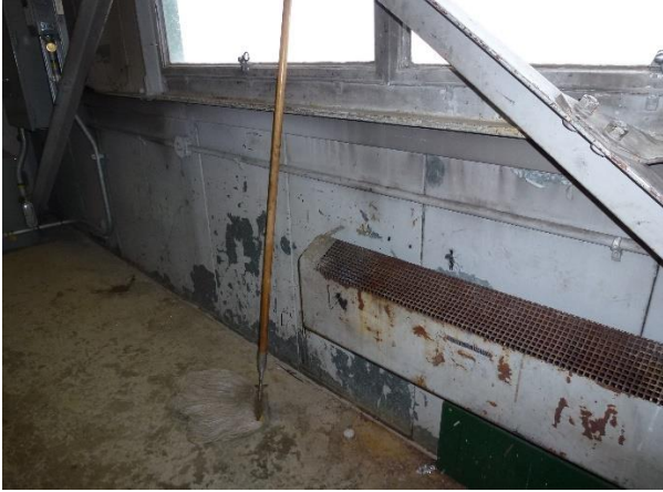
Photo 19: South tower interior grey wall paint.
