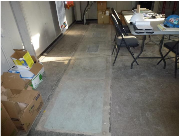
Photo 5: Vinyl tiles (ACM) removed electrical room
