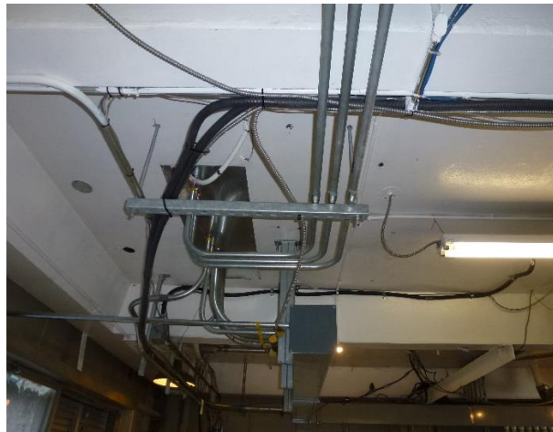
Photo 6: ACM high voltage cables removed
