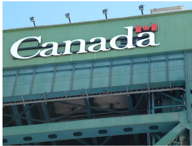
Photo 22: North tower machine room exterior
