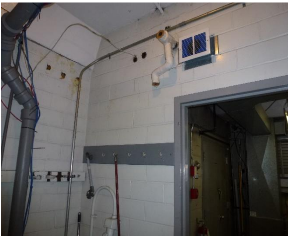
Photo 17: Control house 2 nd floor white wall paint
