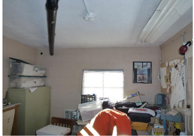
Photo 14: Beige wall paint old workshop
