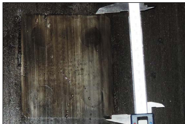
PHOTO 1-4: 130 MM SQUARE PATCH PLATE ON WEST RAM
