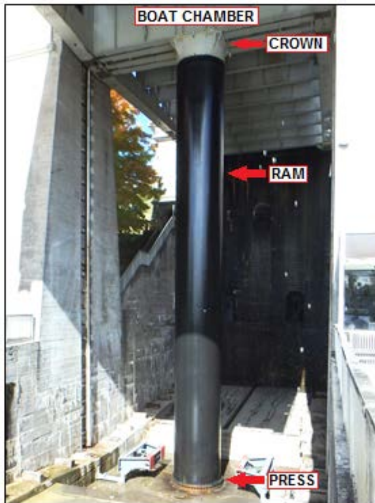
PHOTO 1-2: PRESS, RAM AND CROWN
