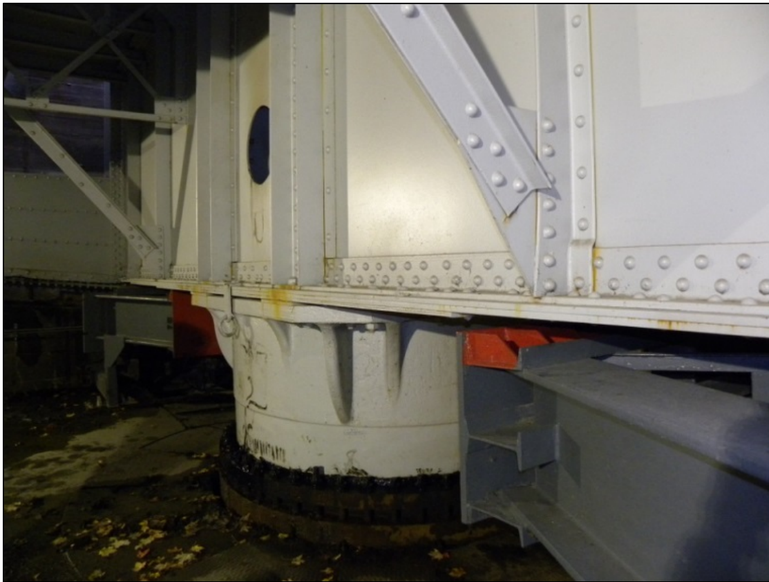
PHOTO 1-6: CHAMBER/RAM IN FULL DOWN POSITION
