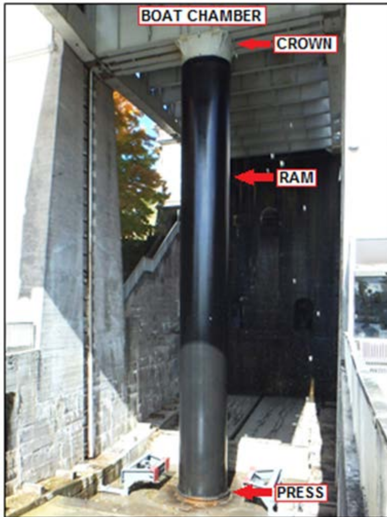
PHOTO 2: PRESS, RAM AND CROWN
