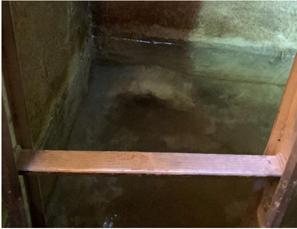
7: 4" drainpipe located at the bottom of cell 1
