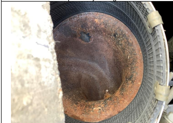
21: View of 6" overflow in cell 1 in good condition
