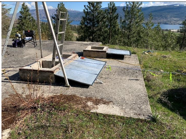
2: View of entrances to tank cells
