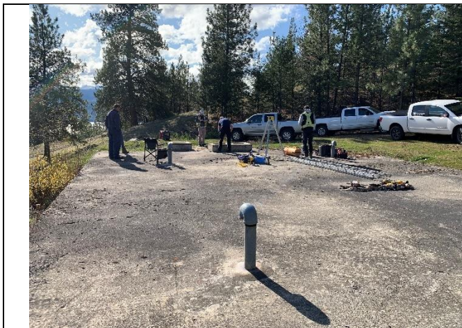
1: View of tank facing south
