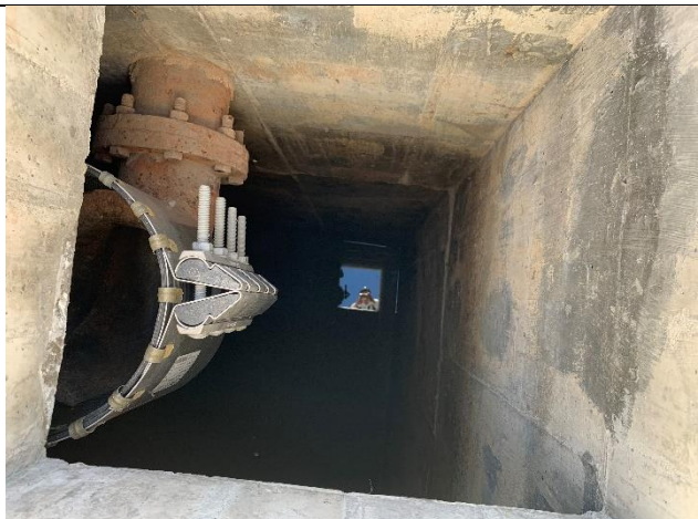
6: View of entrance to cell 2. Access ladder not present
