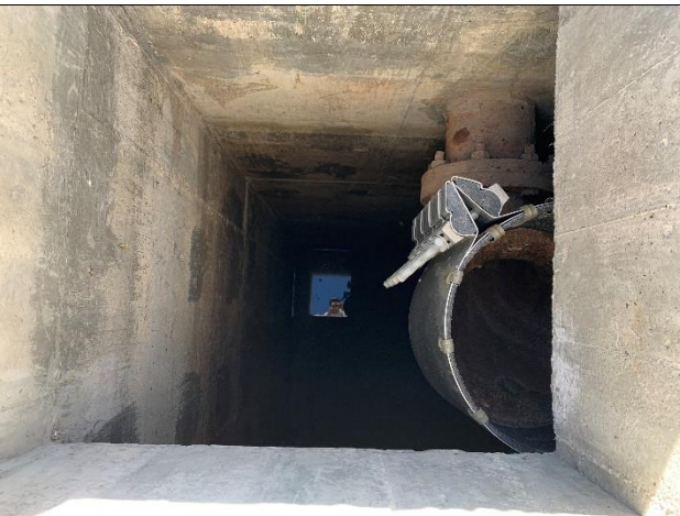
5: View of entrance to cell 1. Access ladder not present
