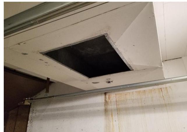
View of the access point of the south interior duct in the firing range.
