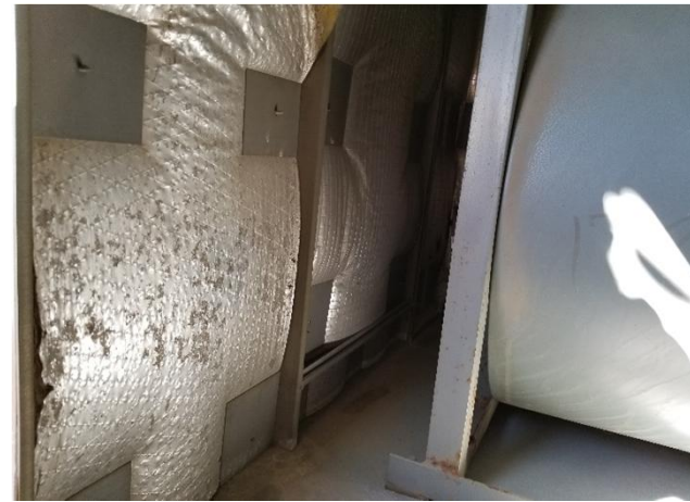
Sample LW-02 swipe from the wall of the duct in the north rooftop air handling unit was determined to have a total lead concentration of 542\mu\text{g}/100\text{cm}^2 .
