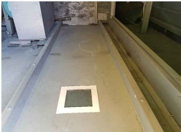
Sample LW-01 swipe from the base of the metal duct in the north rooftop air handling unit was determined to have a total lead concentration of 1240\mu\text{g}/100\text{cm}^2 .
