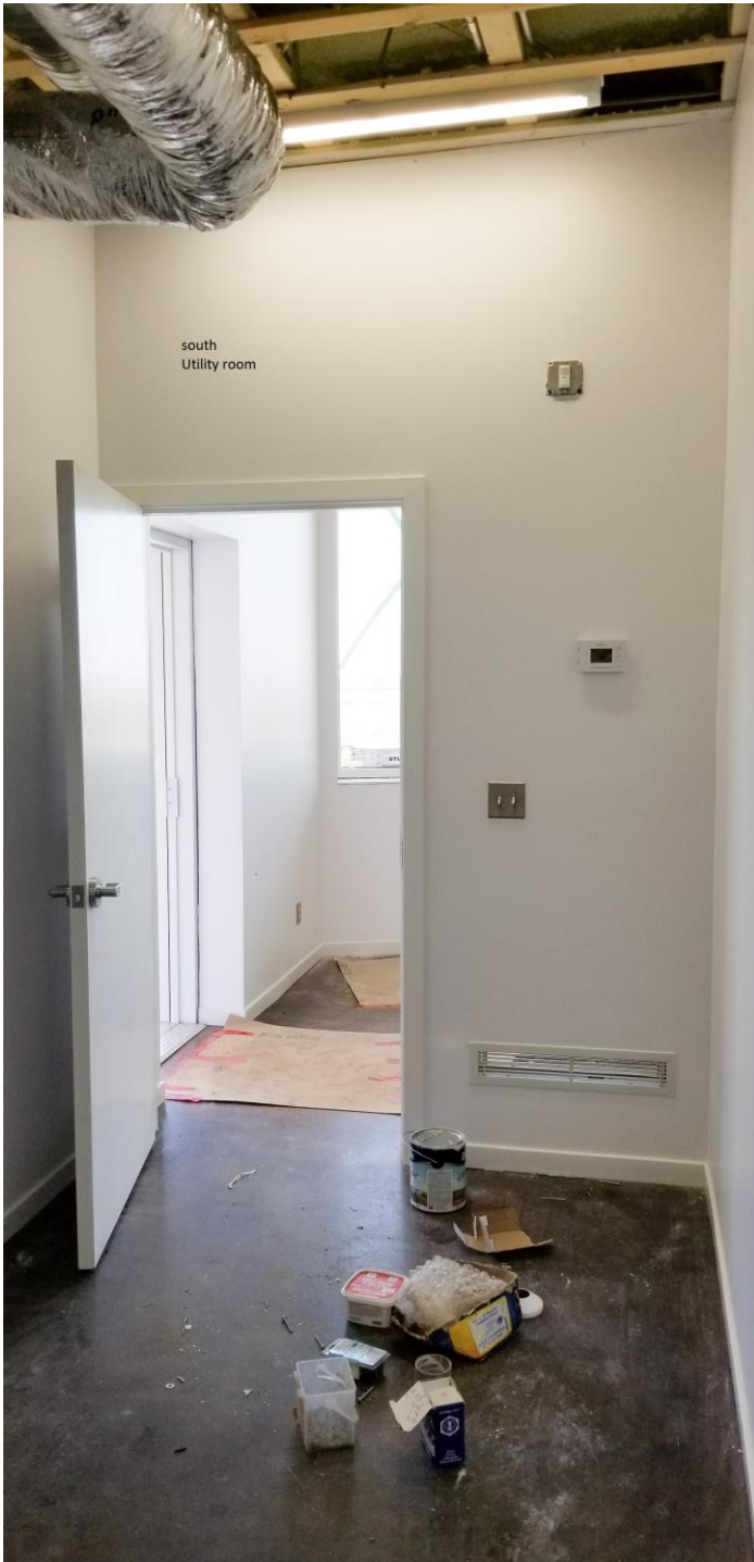
Photo 14: Pavilion – Utility Room facing South
