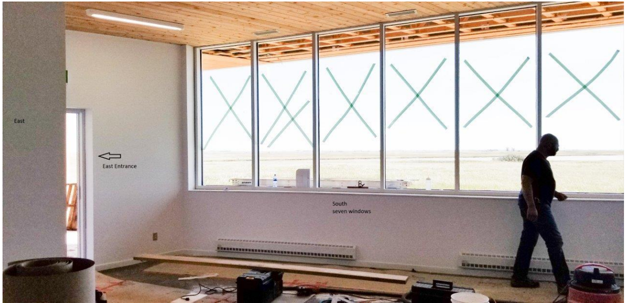
Photo 7: Pavilion - View of South Windows
