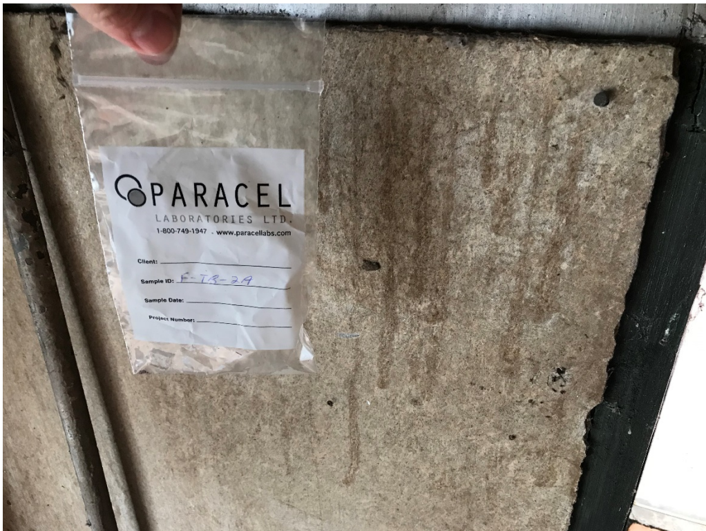
Photo 4: Asbestos-containing transite board. See sample F-TB-2A.
