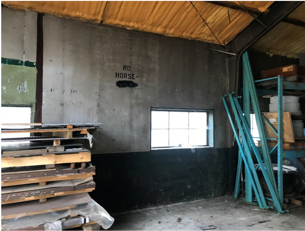
Photo 3: Subject building interior representative finishes.
