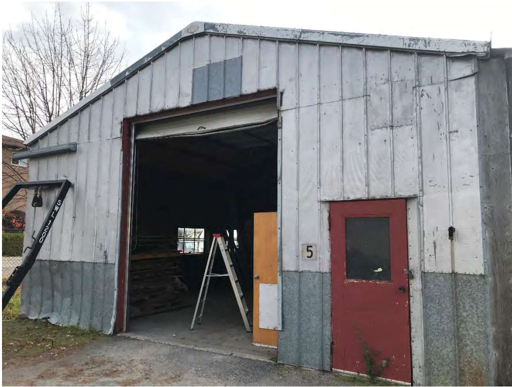
Photo 1: Subject site front view looking south.
