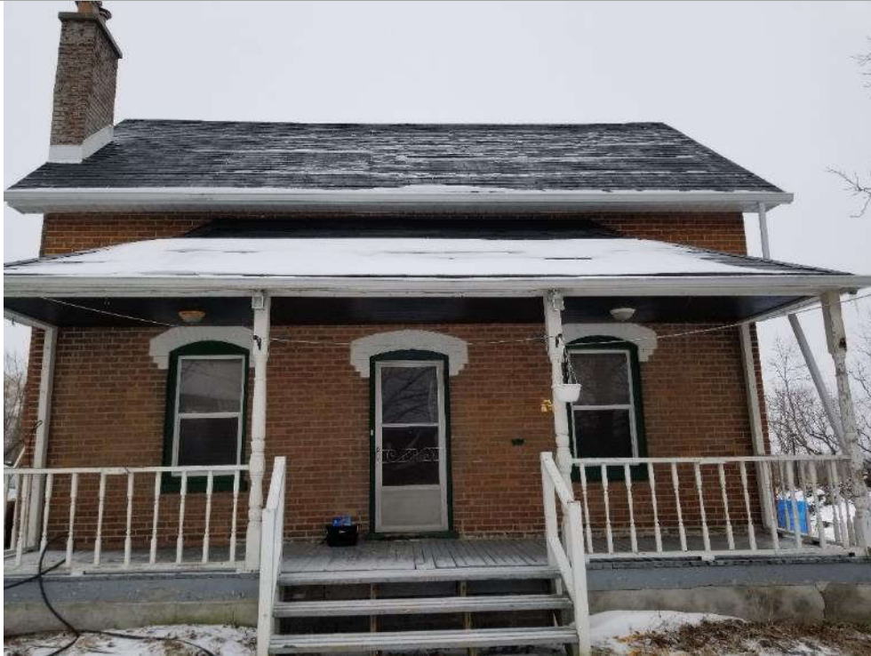
Photo 1: View of the exterior of the residential dwelling.
