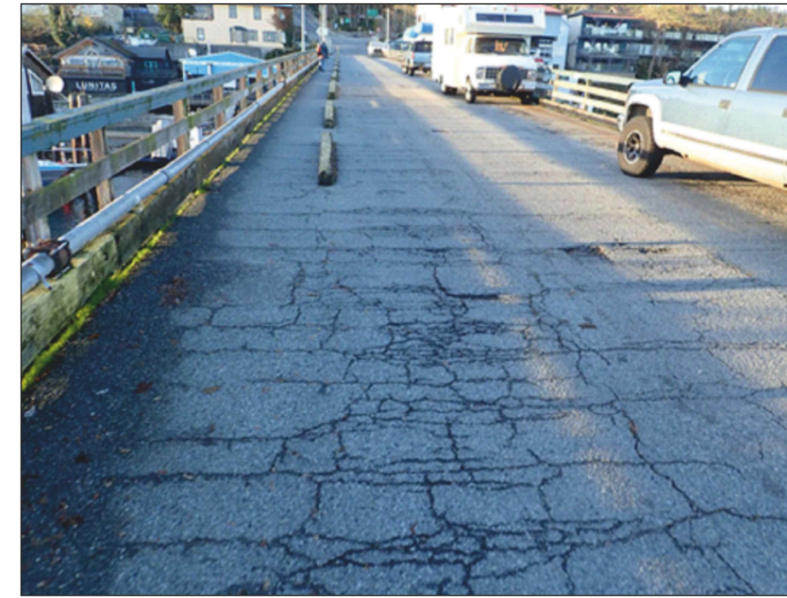
K TYPICAL ASPHALT DECKING CONDITION SCALE: NTS
