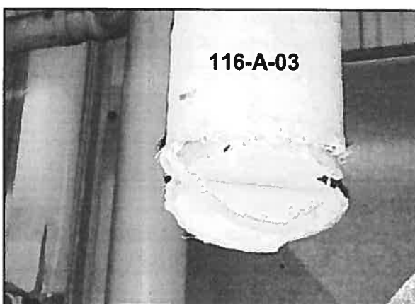
Photo 18.7: Parging cement - no asbestos.
