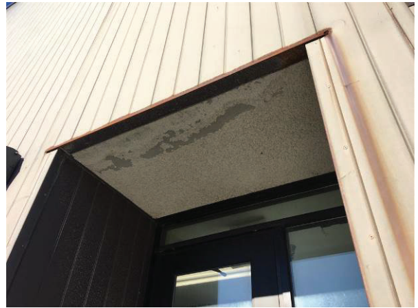
Photo 4: Asbestos-containing exterior texture coat (BS034A & 34B) on PACM cement board
