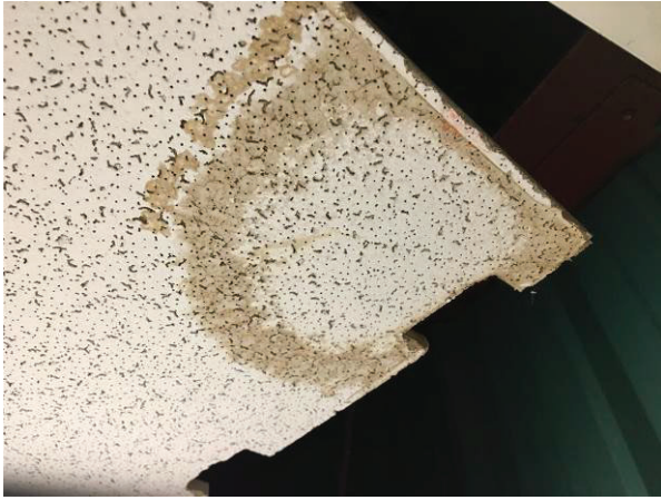
Photo 13: Water damage on acoustic ceiling tile – typical example
