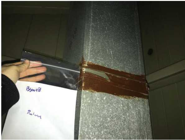
Photo 7: Asbestos-containing sealant (brown) associated with ductwork (BS004B)
