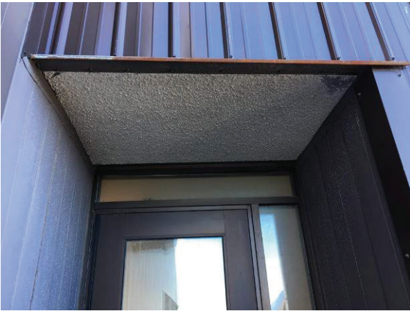
Photo 3: Asbestos-containing exterior texture coat (BS034C) on PACM cement board
