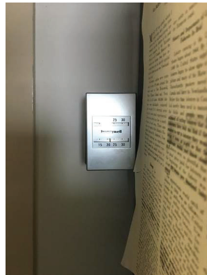
Photo 18: Potential mercury-containing Thermostat
