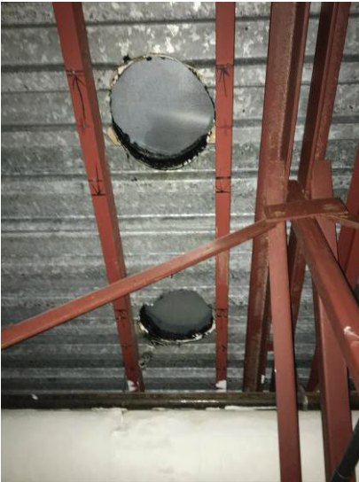
Photo 5: Asbestos-containing tar (black) associated with historical roof vents (BS015)
