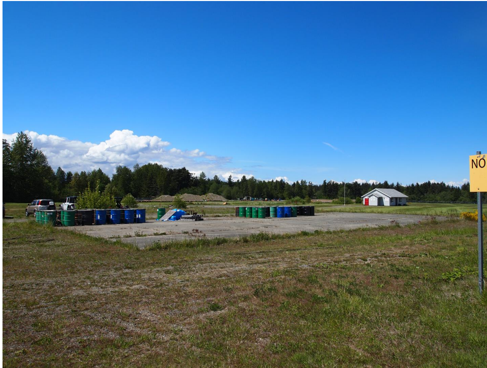
Photo 5: View facing Northwest and situated East of the concrete pad, which is to be removed by the Contractor (May 2020). Drums to be removed.
