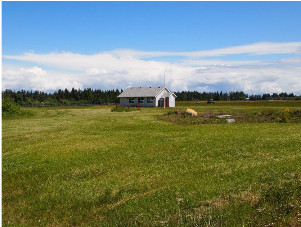
Photo 1: View of FFTA area facing Northeast towards the B:276: Gas Hut (May 2020).
