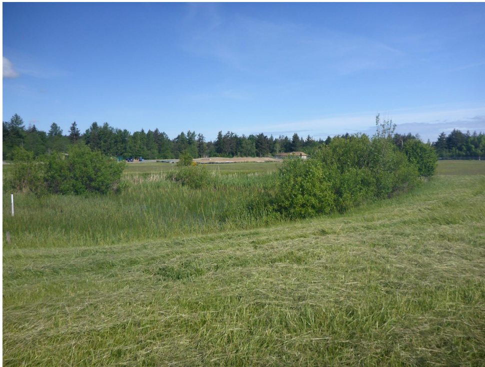
Photo 9: View facing Northwest of the Retention Pond (May 2020).
