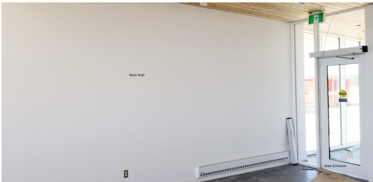
Photo 10: Pavilion - View facing West
