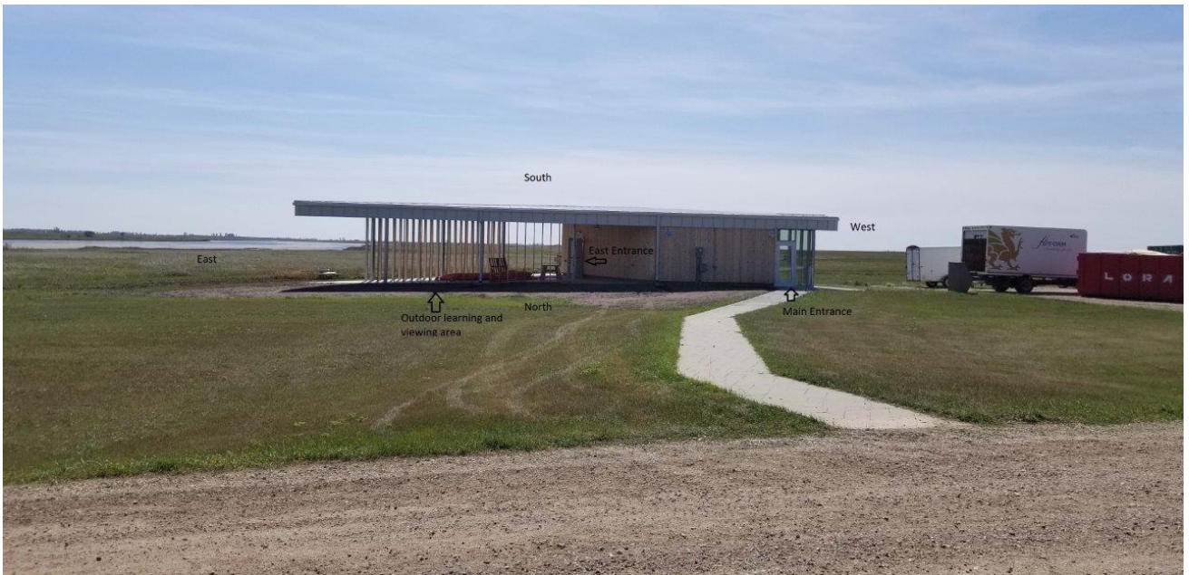
Photo 1: Pavilion - View from North
