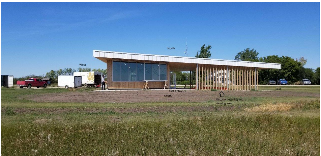
Photo 2: Pavilion - View from South
