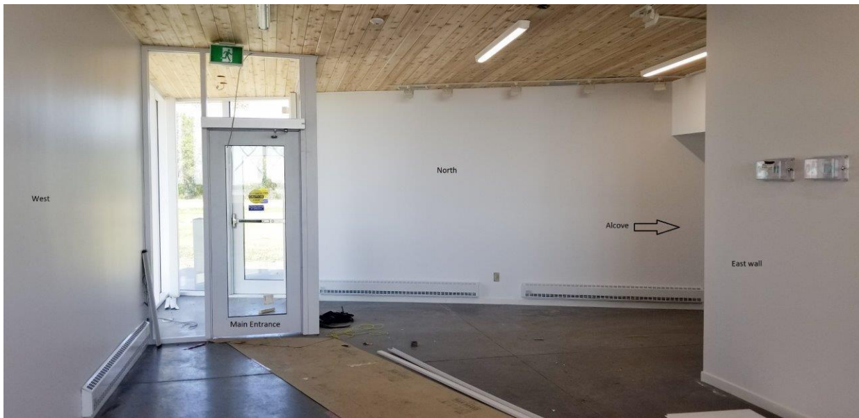
Photo 8: Pavilion - View of Main Doorway facing North
