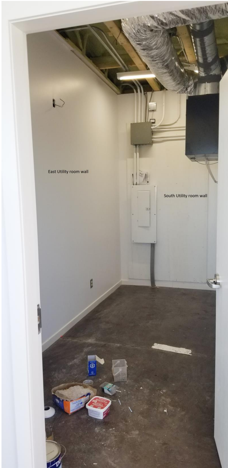
Photo 15: Pavilion – Utility Room facing *North*
