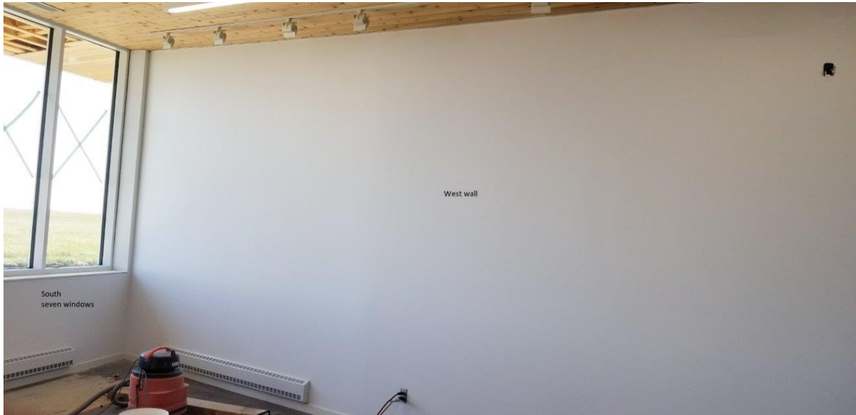
Photo 9: Pavilion - View facing West
