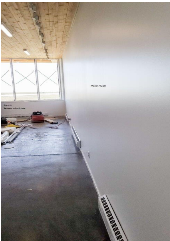
Photo 12: Pavilion – View facing South along West Wall
