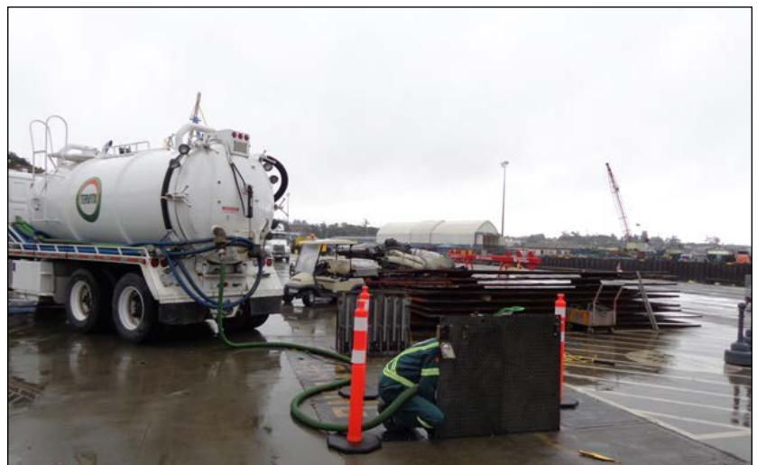
Lift Station Maintenance.
