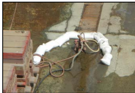
Sand bags used on dock bottom to divert and filter excess water.
