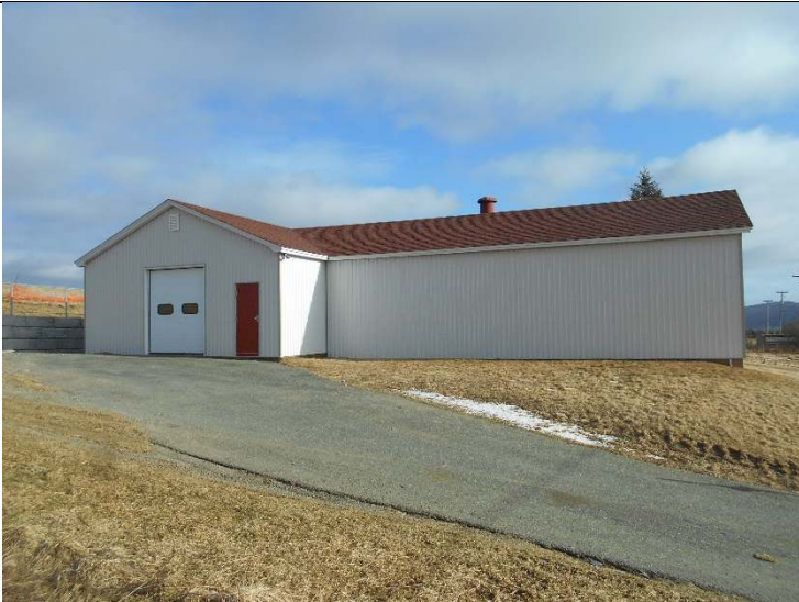
Photo 17-1: View of Building 32 facing east
