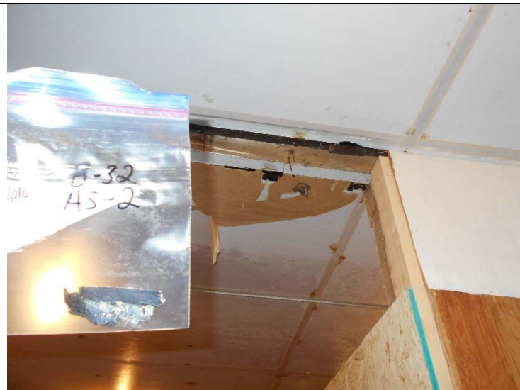
Photo 17-24: View of bulk material sample B-32 AS-2
