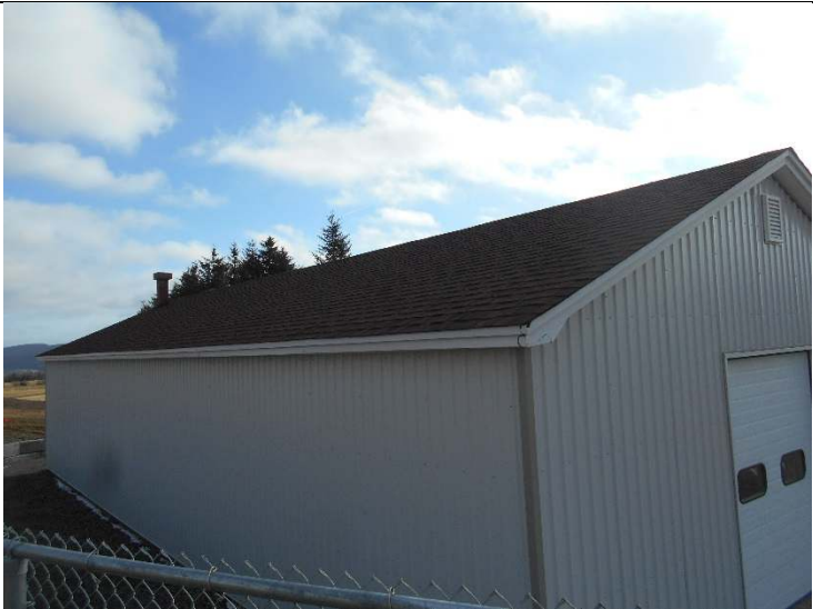
Photo 17-5: View of building 32 facing southeast
