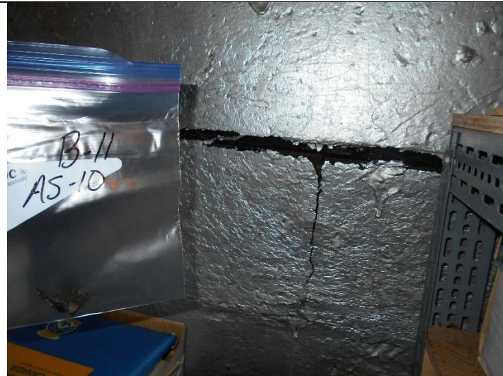
Photo 7-44: View of bulk material sample B-11 AS-10
