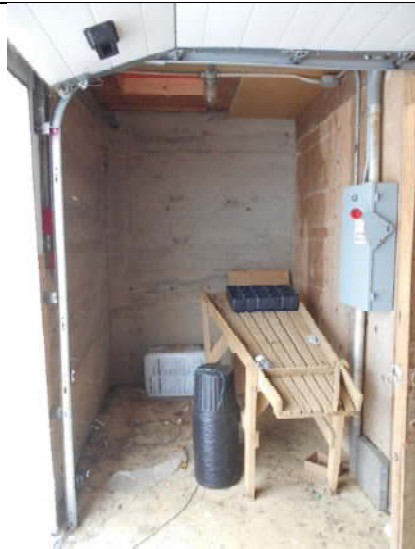
Photo 17-17: View of Room 3 (Basement)
