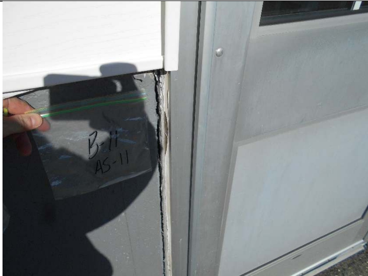
Photo 7-45: View of bulk material sample B-11 AS-11
