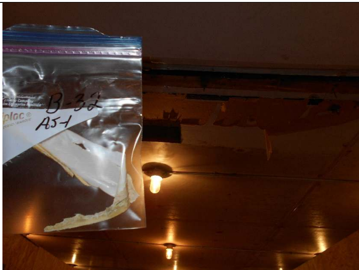
Photo 17-23: View of bulk material sample B-32 AS-1
