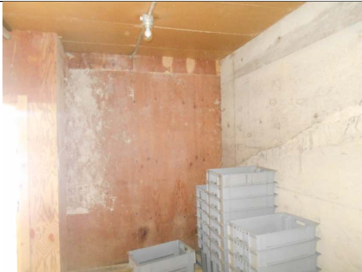
Photo 17-21: View of Room 3 (Basement)
