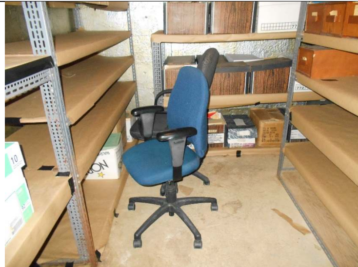
Photo 7-32: View of Room 13 (Cold Storage)
