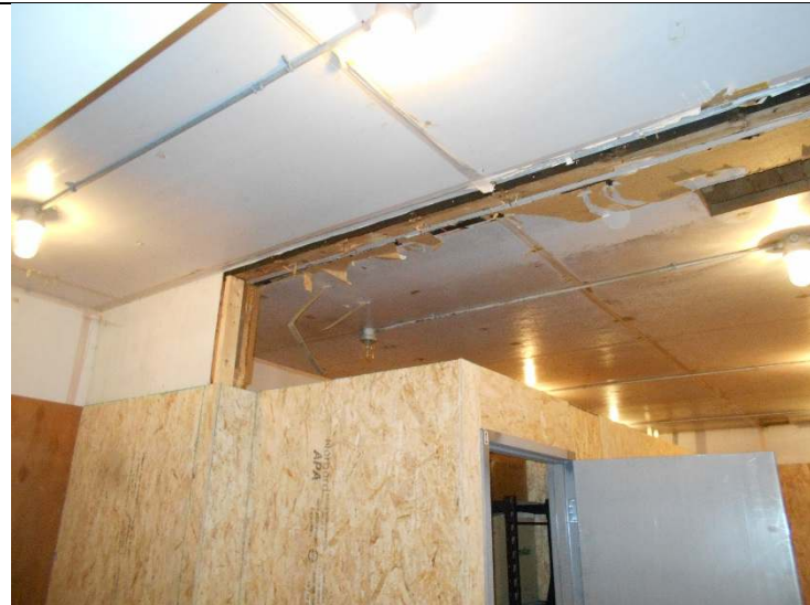
Photo 17-12: View of ceiling in Room 1
