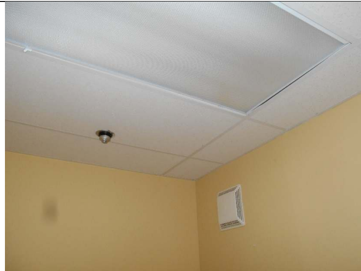
Photo 7-28: View of Room 11 (Washroom)
