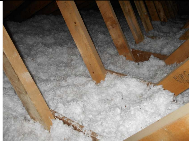
Photo 7-14: View of insulation above Room 4
