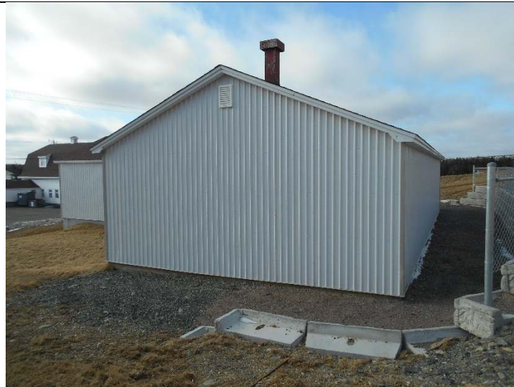
Photo 17-4: View of building 32 facing west
