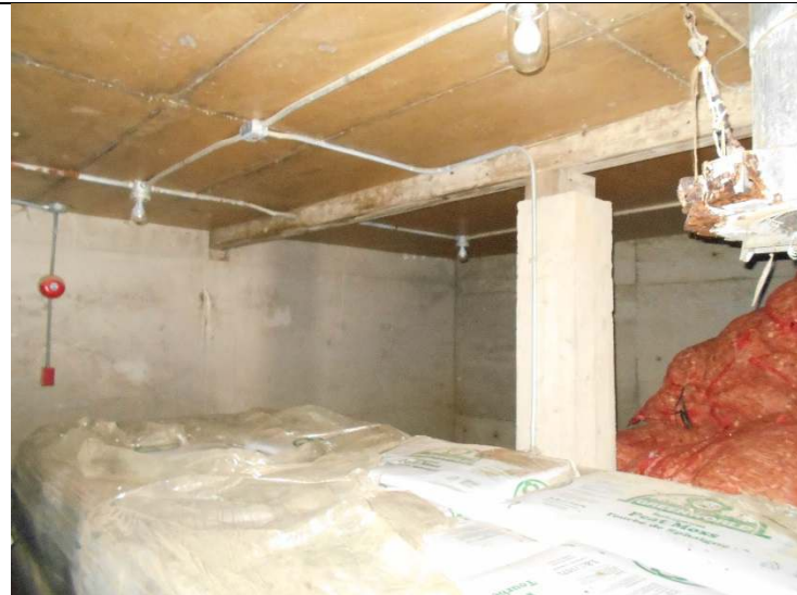
Photo 17-20: View of Room 3 (Basement)
