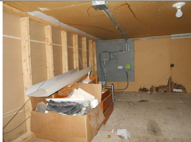
Photo 7-12: View of Room 4 (Attic)
