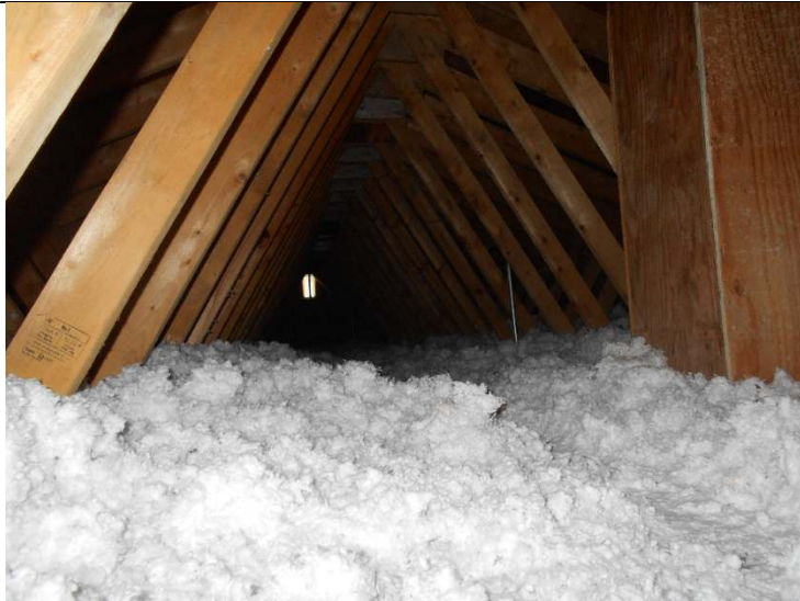
Photo 7-13: View of insulation above Room 4
