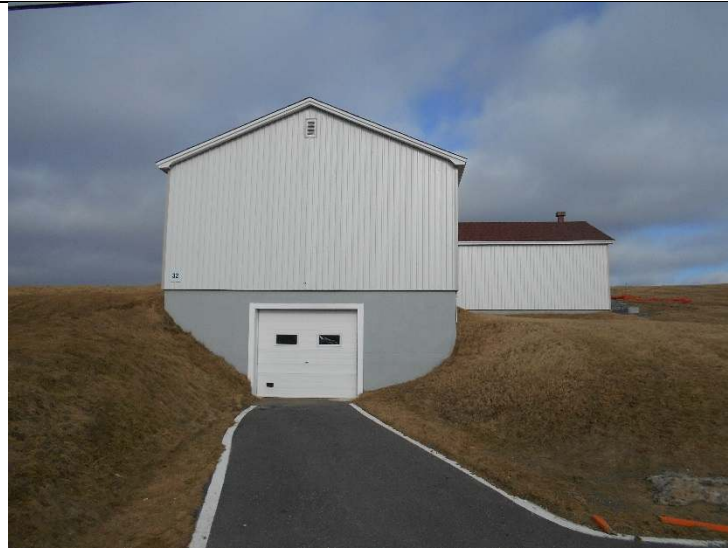
Photo 17-2: View of Building 32 facing north
