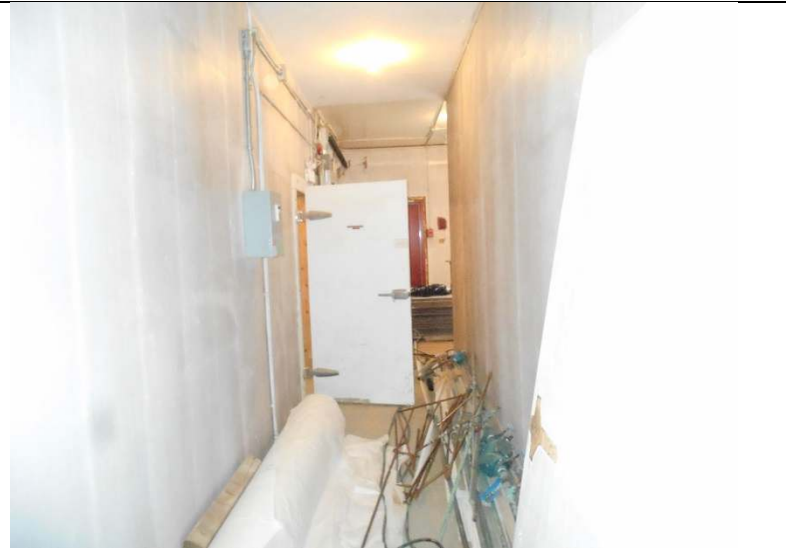
Photo 17-10: View of Room 1 (Cool Room)
