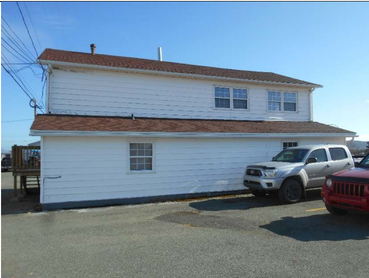
Photo 7-3: View of Building 11 facing east
