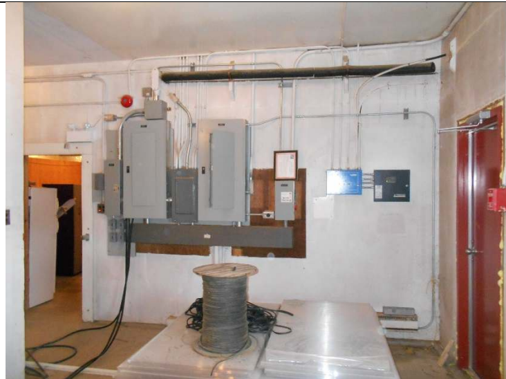
Photo 17-8: View of Room 1 (Cool Room)
