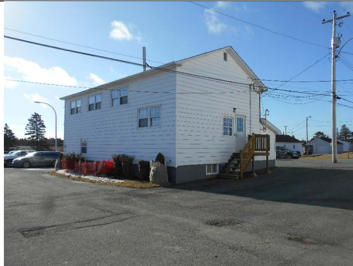
Photo 7-2: View of Building 11 facing south-west
