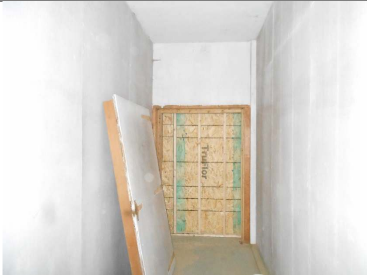
Photo 17-9: View of Room 1 (Cool Room)
