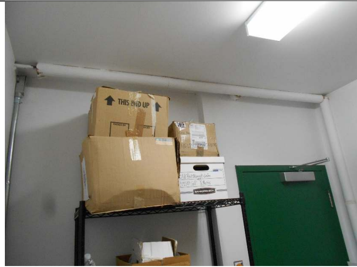
Photo 7-10: View of Room 3 (Office)
