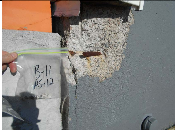
Photo 7-46: View of bulk material sample B-11 AS-12
