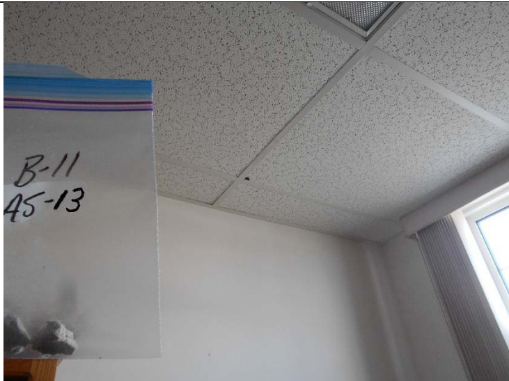
Photo 7-47: View of bulk material sample B-11 AS-13
