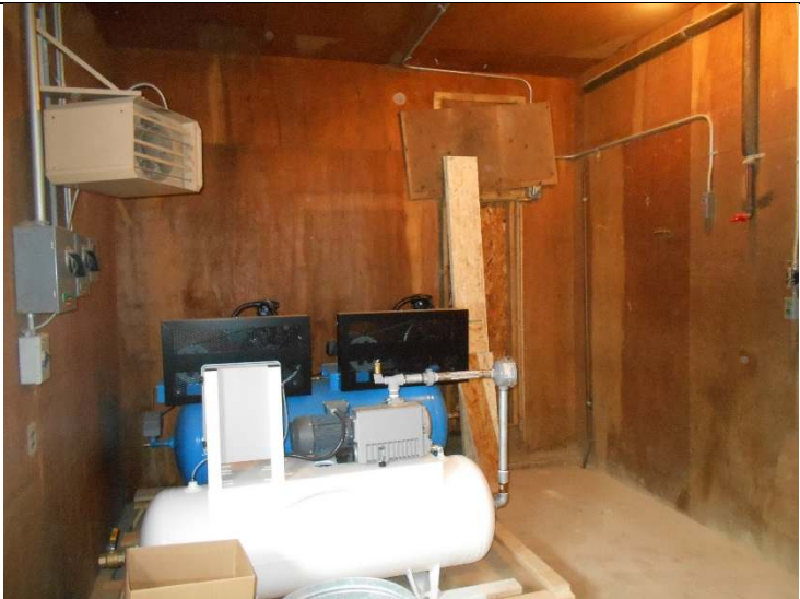
Photo 17-7: View of Room 1 (Cool Room)
