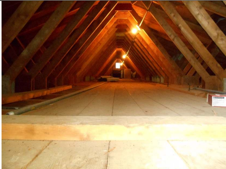
Photo 17-13: View above ceiling in Room 1
