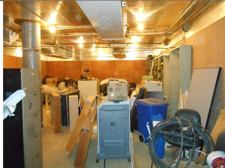
Photo 17-14: View of Room 2 (Cool Room)
