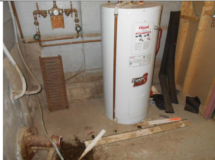
Photo 7-20: View of Room 7 (Janitor Closet)
