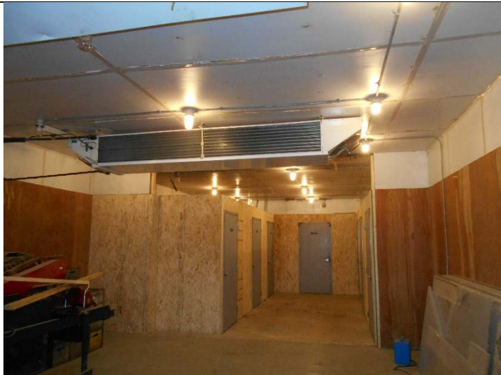
Photo 17-11: View of Room 1 (Cool Room)
