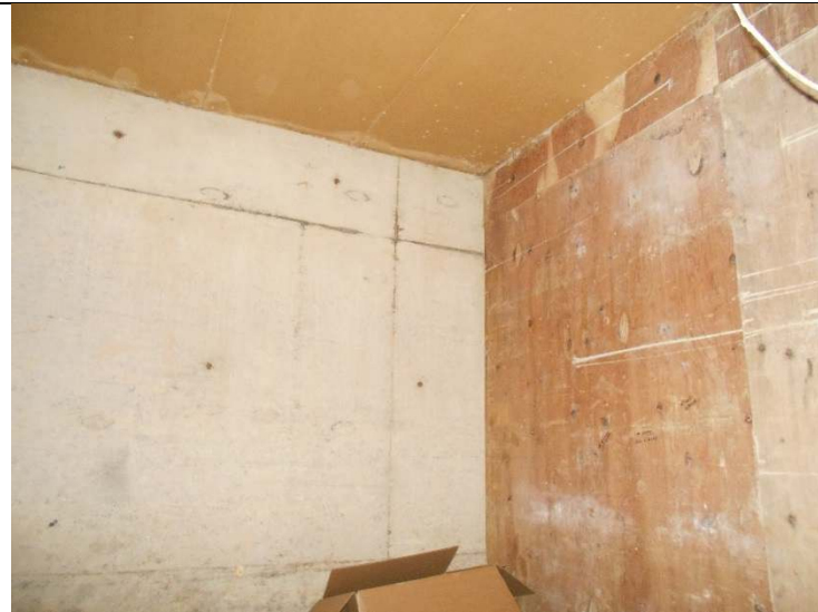
Photo 17-22: View of Room 3 (Basement)
