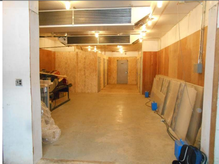
Photo 17-6: View of Room 1 (Cool Room)
