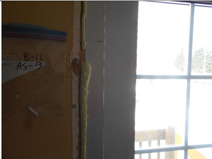
Photo 7-43: View of bulk material sample B-11 AS-9
