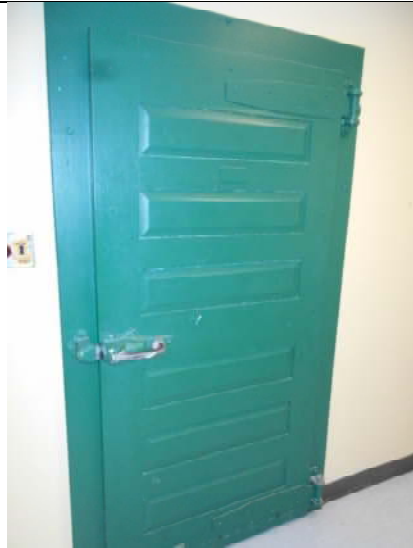
Photo 7-33: View of door to Room 13
