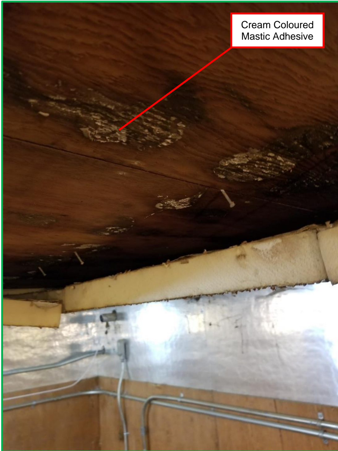
Photograph #1: Sample NL7687-A04 sample location. Cream coloured insulation panel adhesive. Photo taken on November 16, 2020.
