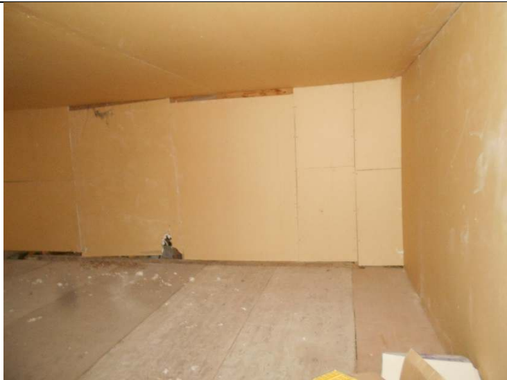
Photo 7-11: View of Room 4 (Attic)
