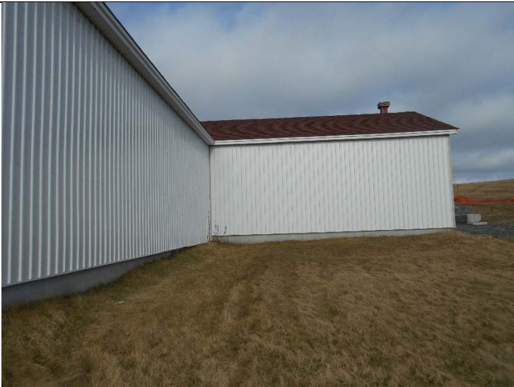
Photo 17-3: View of building 32 facing north
