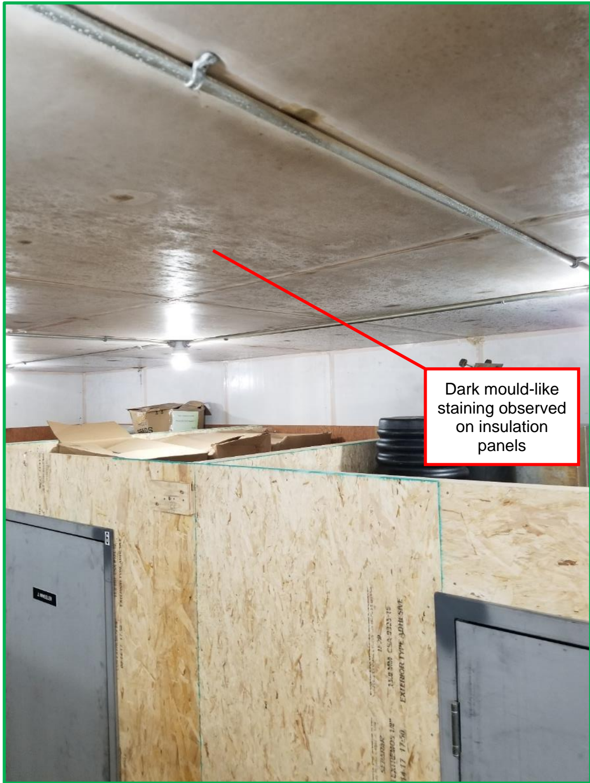
Photograph #3: Dark mould-like staining observed on the insulation panels within the Main Cooler/Storage Area on the Main Floor of the Building. Photo taken on November 16, 2020.
