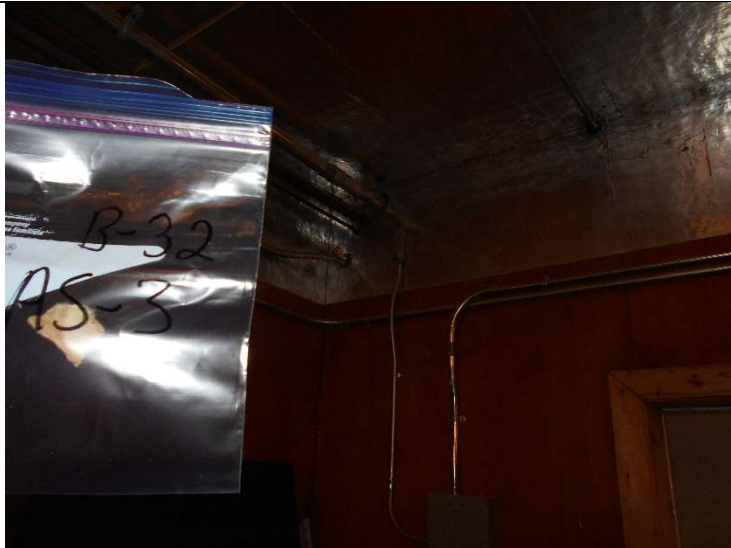
Photo 17-25: View of bulk material sample B-32 AS-3
