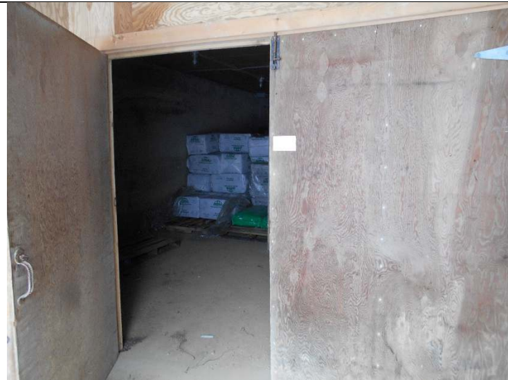
Photo 17-18: View of Room 3 (Basement)
