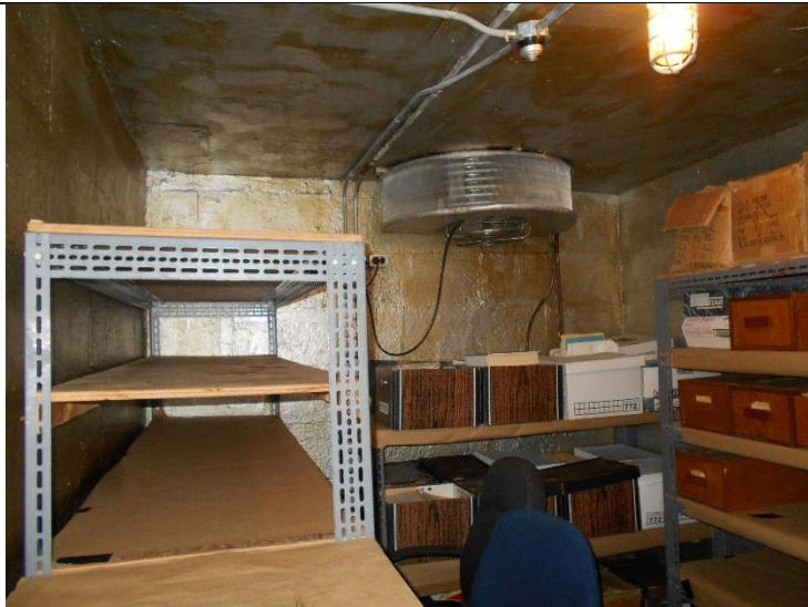
Photo 7-31: View of Room 13 (Cold Storage)
