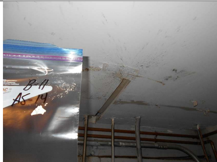
Photo 7-48: View of bulk material sample B-11 AS-14
