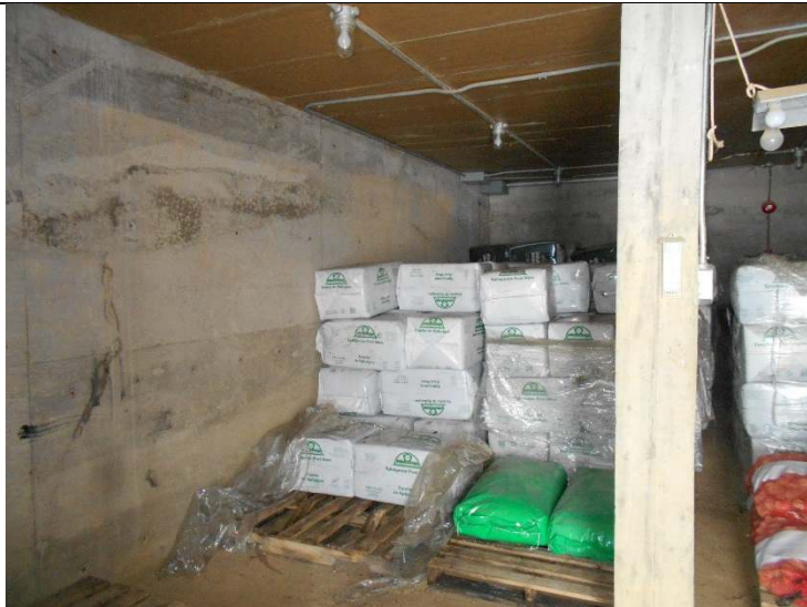
Photo 17-19: View of Room 3 (Basement)
