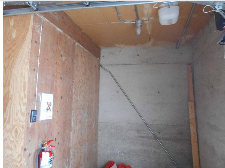
Photo 17-16: View of Room 3 (Basement)
