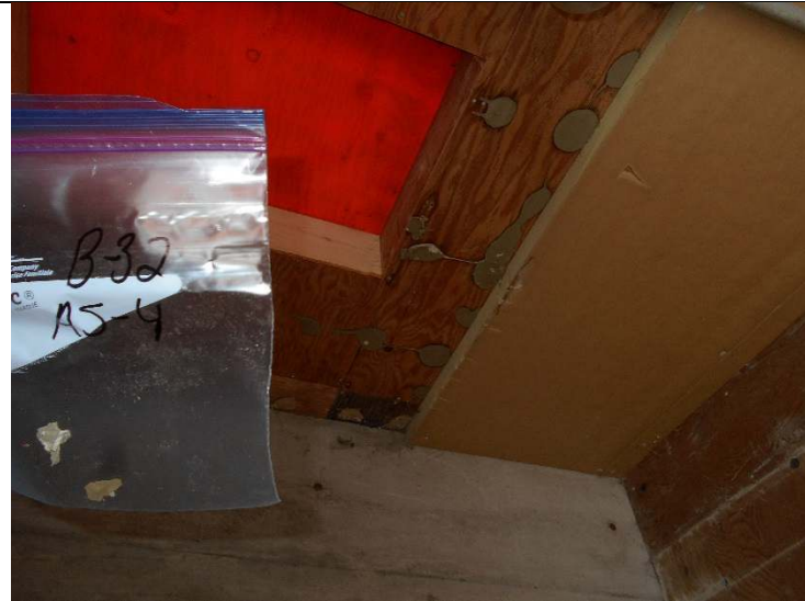
Photo 17-26: View of bulk material sample B-32 AS-4
