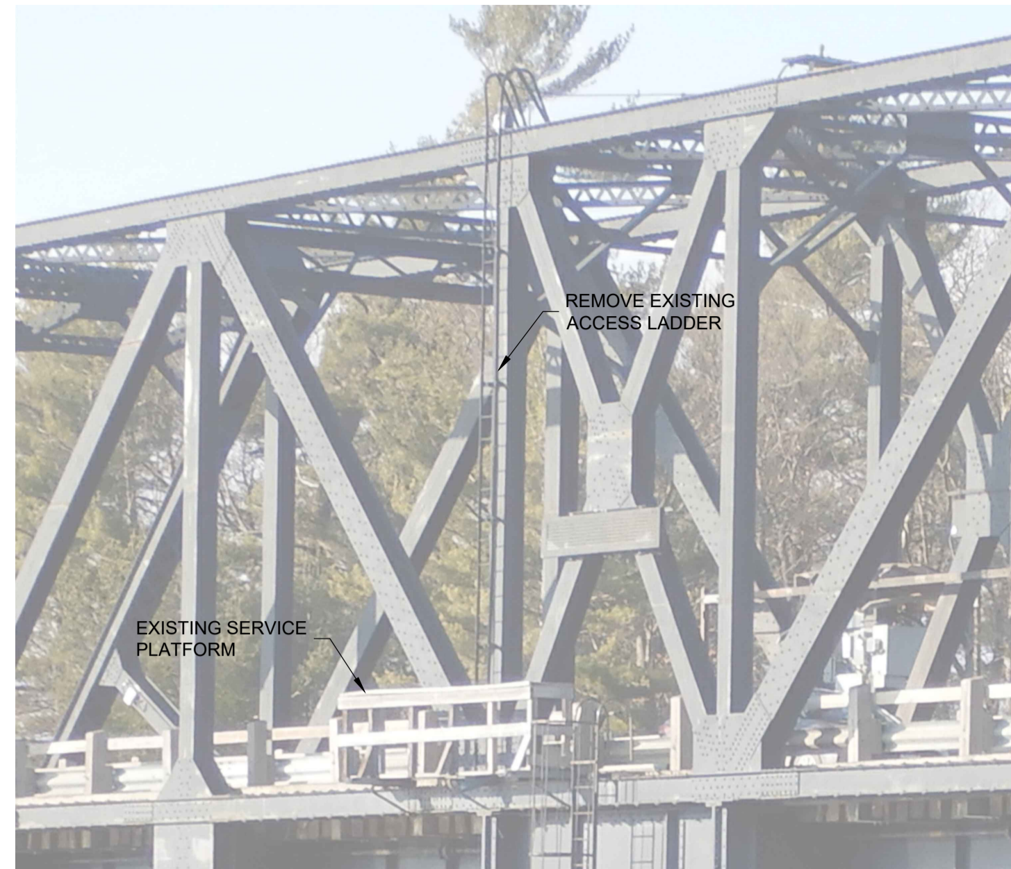
SOUTH ELEVATION - EXISTING ACCESS LADDER
