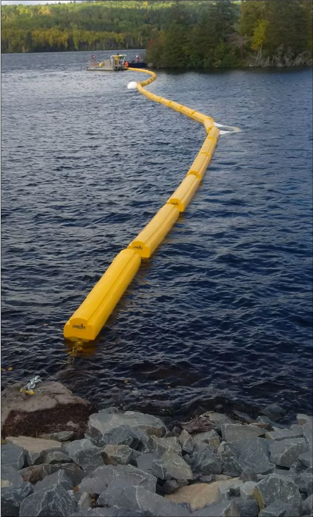
Figure 7: Existing waterway barrier during its installation, looking from right shore towards spit.
