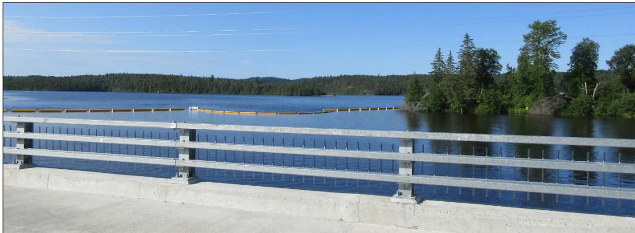
Figure 4: View of existing waterway barrier, looking upstream from deck of Latchford Dam.
