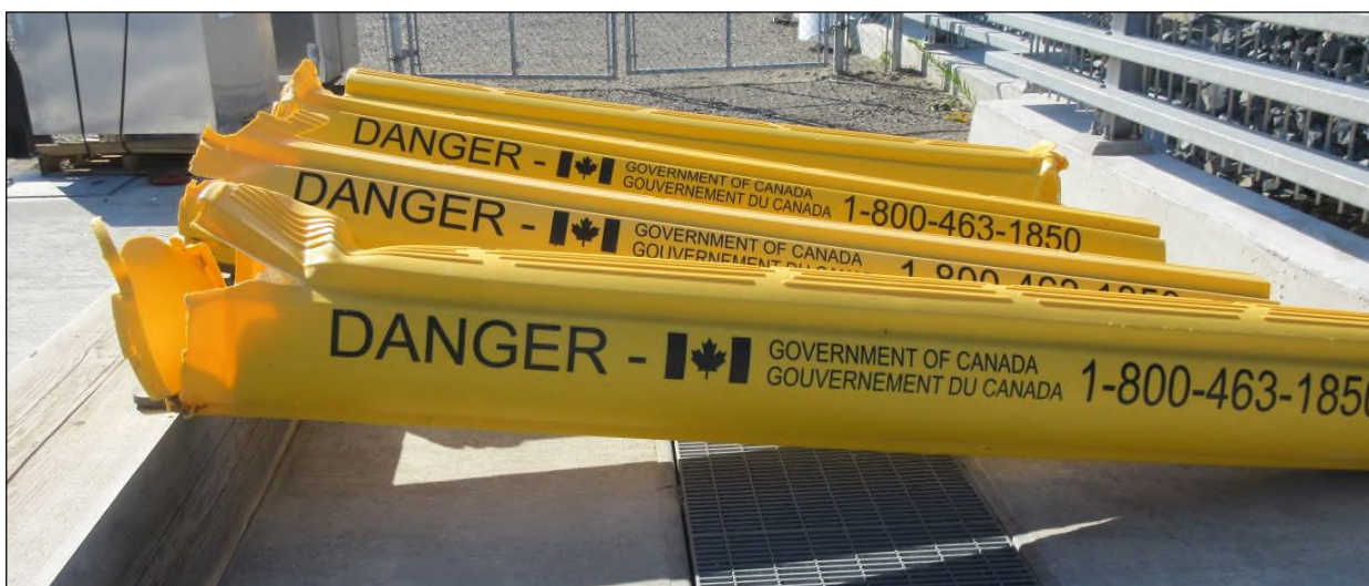
Figure 5: Close-up view of warning message and contact information on existing waterway barrier. These floats shown were those that had been damaged by ice.
