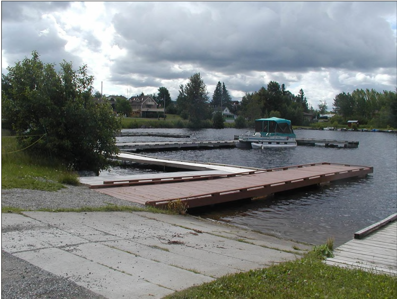
Figure 9: Boat launch at Marina in Town of Latchford, upstream of Latchford Dam.
