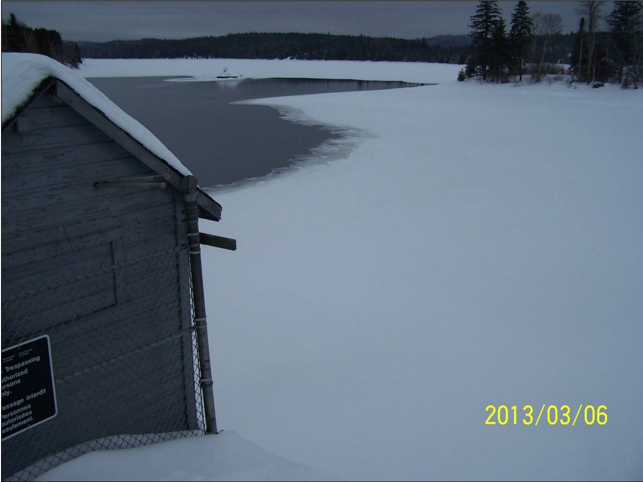
Figure 10: Ice conditions upstream of Latchford Dam (typical). The spit of land upon which the left anchor is located is visible in the upper right of the photograph.
