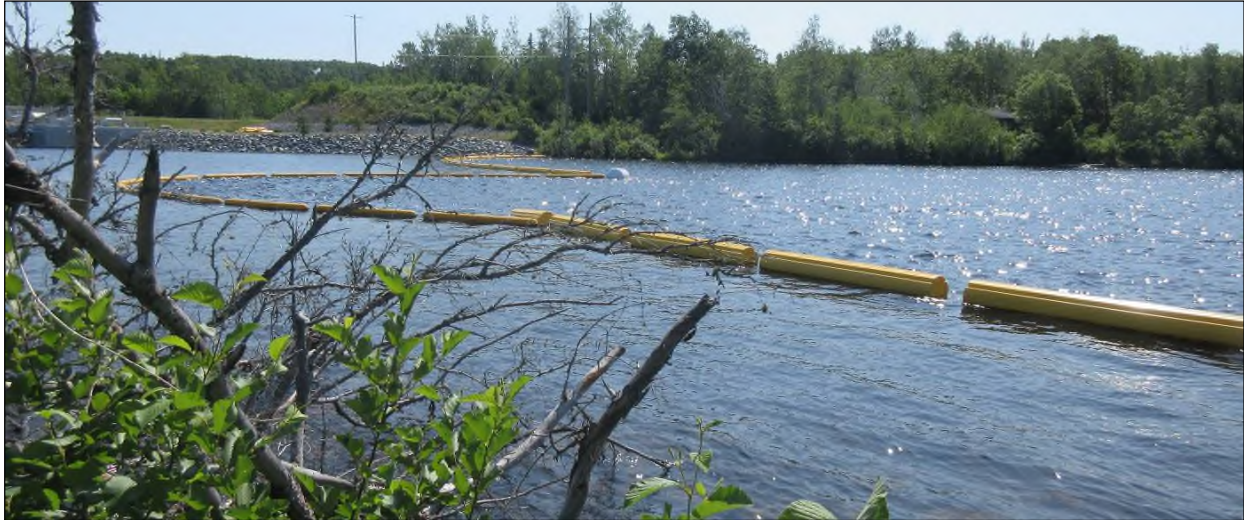
Figure 8: Existing waterway barrier, in position, after ice damage occurred.
