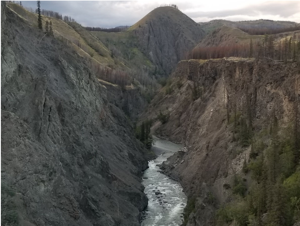
Photo 1: Tahltan River and slide site, looking north
