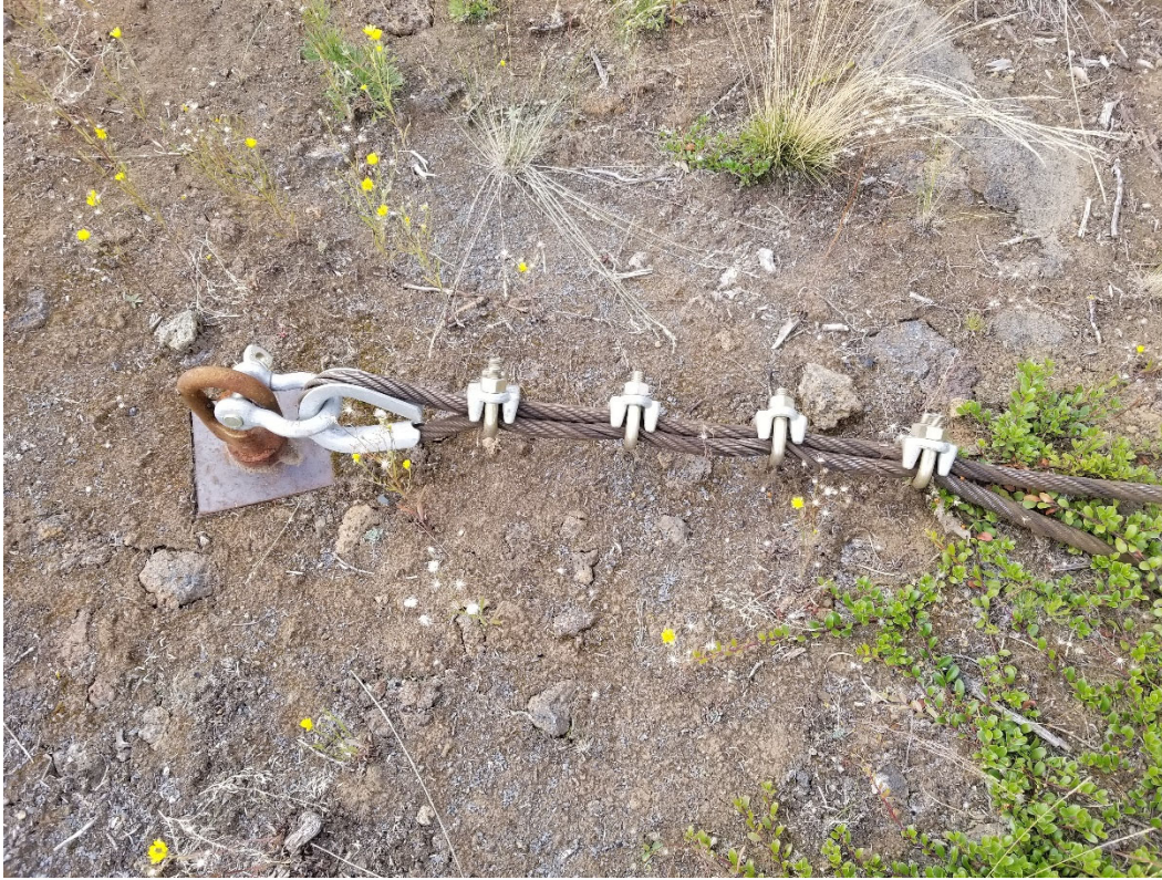
Photo 5: Mesh anchor assembly
