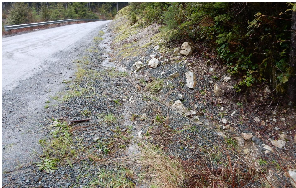
Photo 3-4 Road Run-off Observed Downslope of the Mapped Location of Pretty Tributary 1
