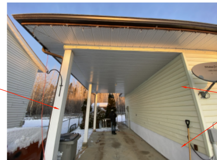
5. VIEW OF CARPORT
