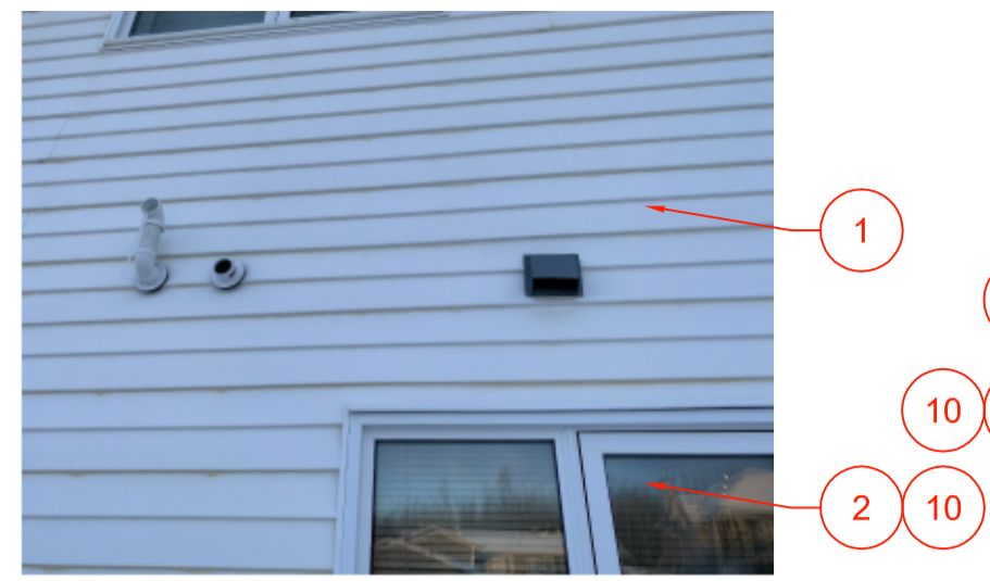
5. SERVICE PENETRATIONS AT THE BACK
