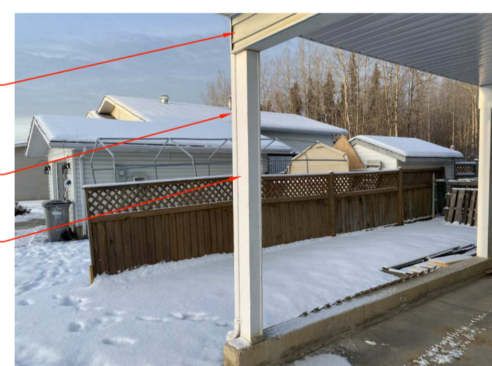
8. STRUCTURE ABOVE CARPORT
