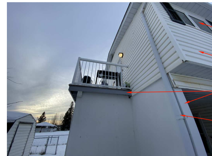
6. DECK AND SEMI-ENCLOSED CARPORT
