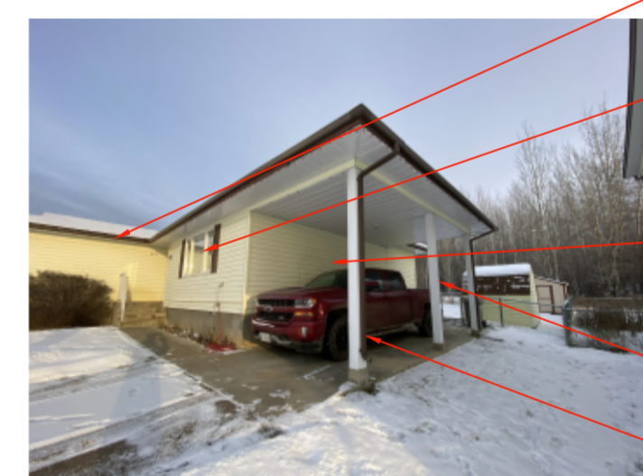
10. VIEW OF WALL BESIDE CARPORT
