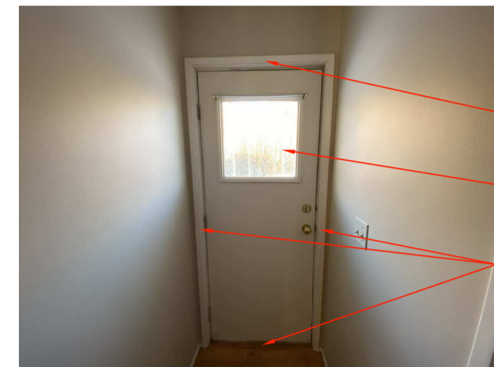
11. INTERIOR VIEW OF DOOR
