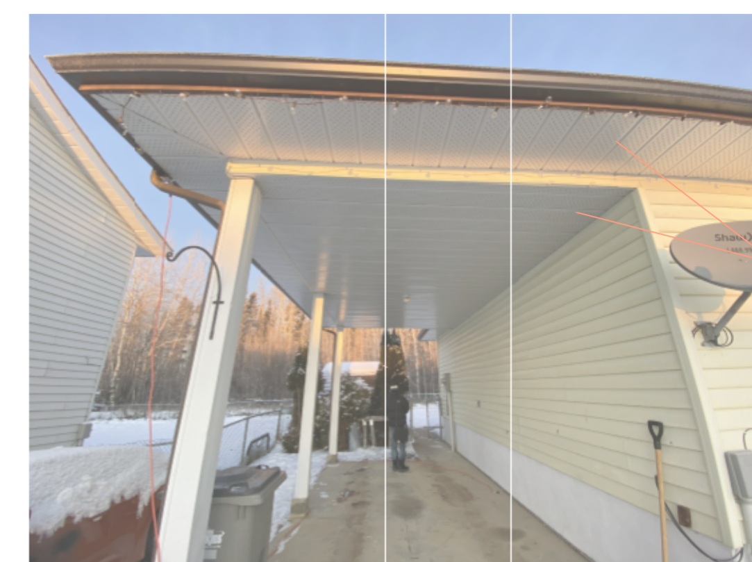
EXISTING SOFFIT TO REMAIN
