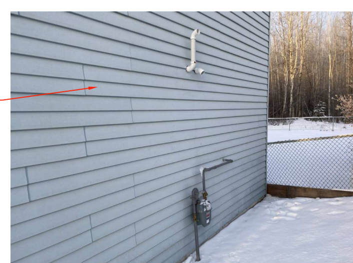
9. SIDE VIEW WITH SERVICE PENETRATIONS
