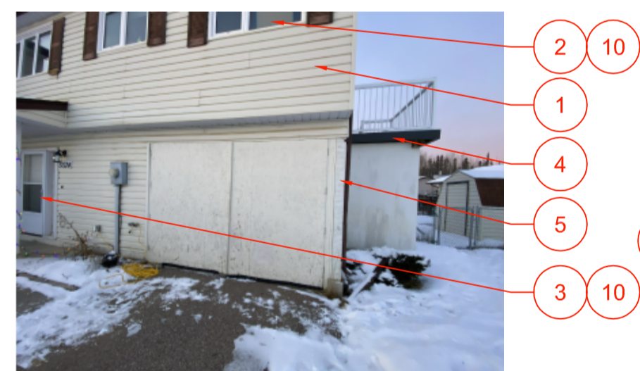
1. FRONT VIEW OF ENCLOSED CARPORT
