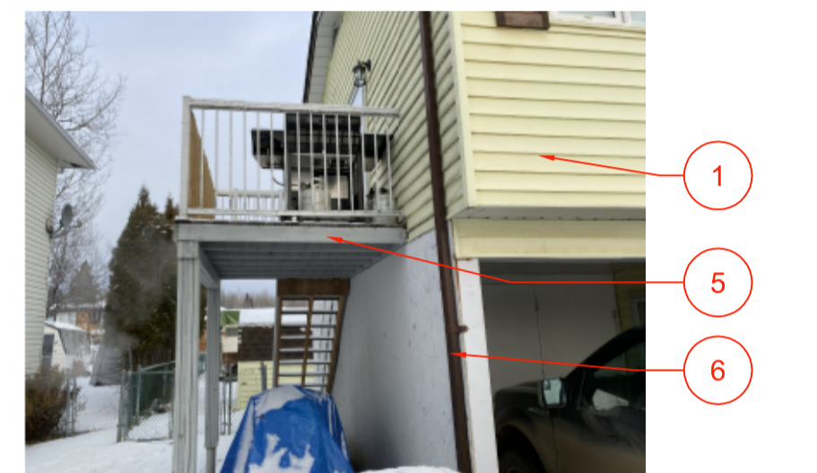
9. VIEW OF DECK AND SEMI-ENCLOSED CARPORT
