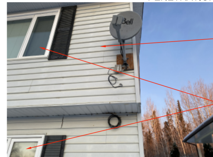
3. SATELLITE DISH AND CABLE PENETRATION
