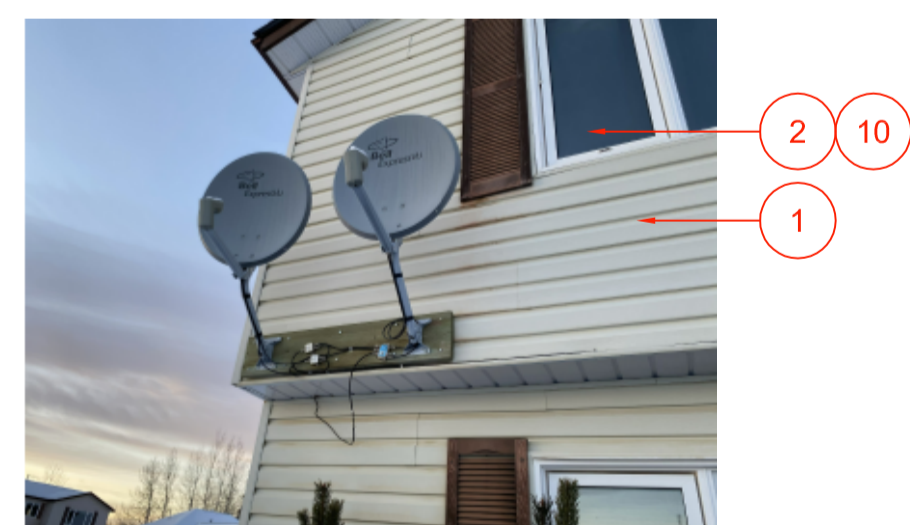
5. VIEW OF SATELLITE DISHES AT FRONT
