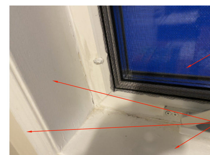
11. INTERIOR VIEW OF WINDOW
