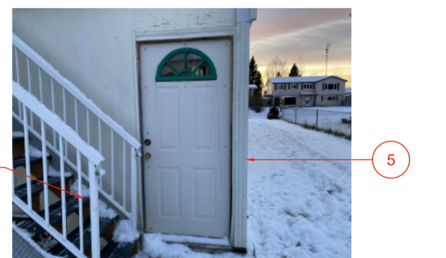
4. VIEW OF DOOR TO ENCLOSED CARPORT
