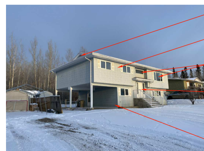
1. VIEW OF CARPORT AND ENTRY
