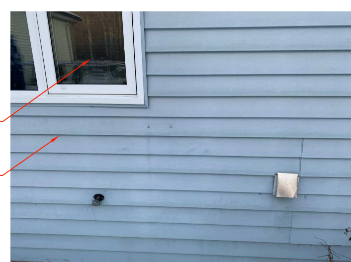
6. VIEW OF SERVICE PENETRATIONS AT BACK
