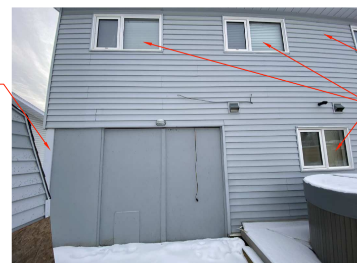
5. VIEW OF ENCLOSED CARPORT FROM BACK
