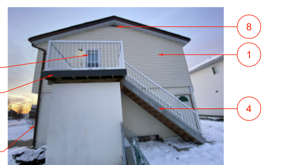
6. VIEW OF ENCLOSED CARPORT BELOW DECK
