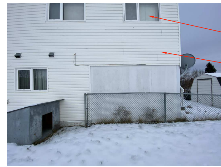
4. VIEW OF SEMI-ENCLOSED CARPORT FROM BACK
