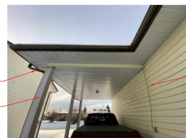
9. VIEW OF CARPORT AND SOFFIT ABOVE
