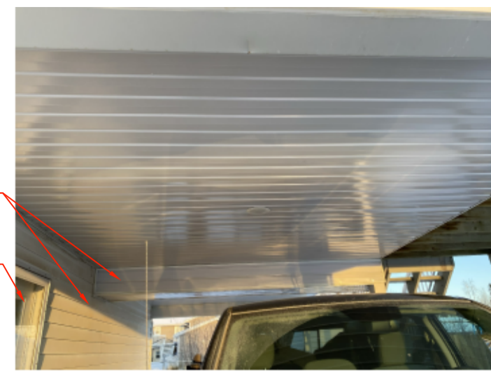
9. VIEW OF SOFFIT ABOVE CARPORT
