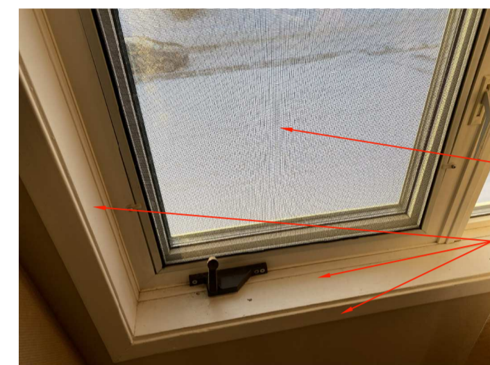
12. INTERIOR VIEW OF TYPICAL WINDOW
