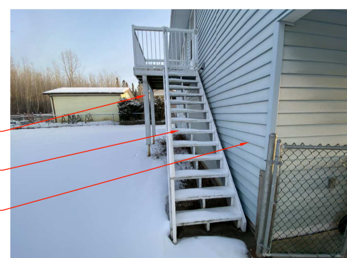
5. STAIR TO DECK
