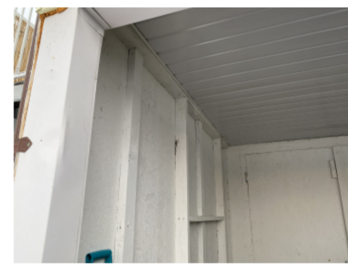
7. VIEW OF CARPORT ENCLOSING WALL
