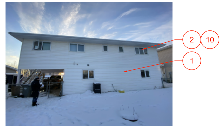
3. BACK VIEW WITH SERVICE PENETRATIONS
