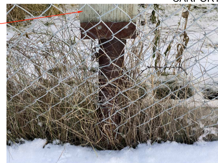
9. SUPPORT OF DECK STRUCTURE
