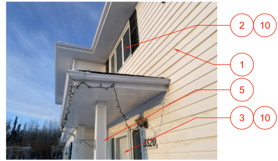
8. VIEW OF CANOPY ABOVE ENTRY
