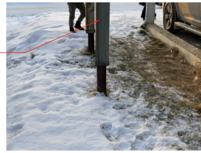
10. SUPPORT OF DECK STRUCTURE
