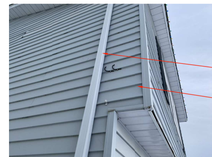
7. CABLE PENETRATION AT SIDE
