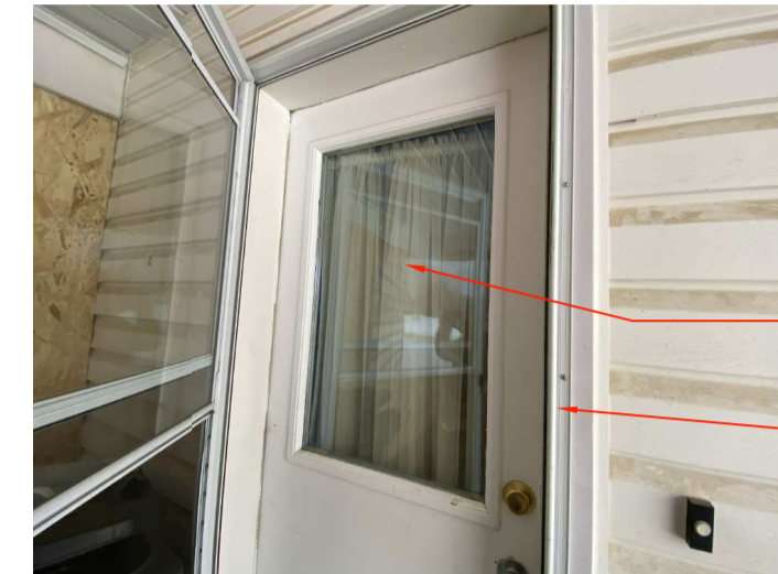
8. DOOR TO INTERIOR FROM CARPORT
