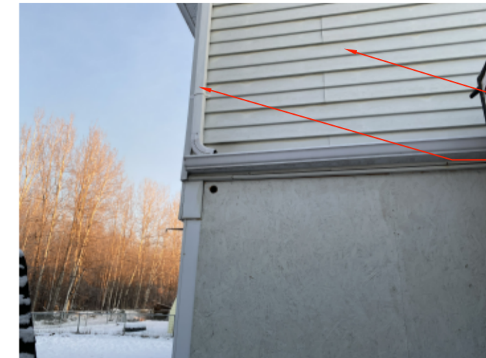
10. WALL ENCLOSING CARPORT
