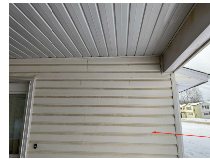
7. WALL FINISHES IN CARPORT
