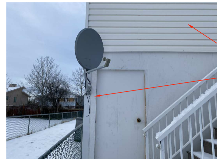
3. DOOR TO CARPORT AT BOTTOM OF STAIR
