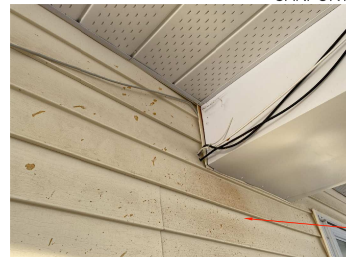
8. CABLE PENETRATION AT CEILING OF CARPORT
