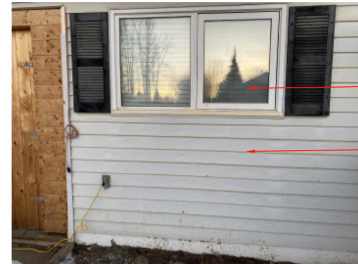
2. CARPORT DOOR AND SERVICE PENETRATION
