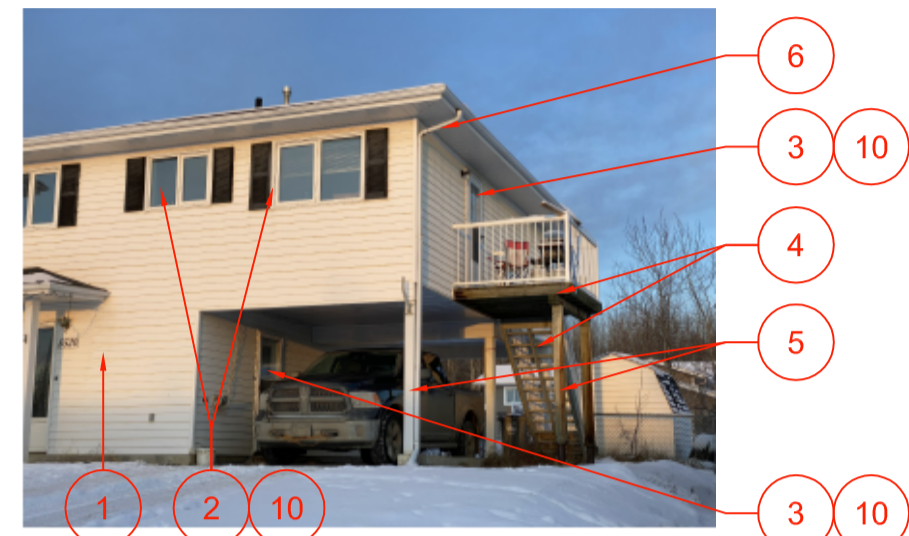
2. VIEW OF CARPORT
