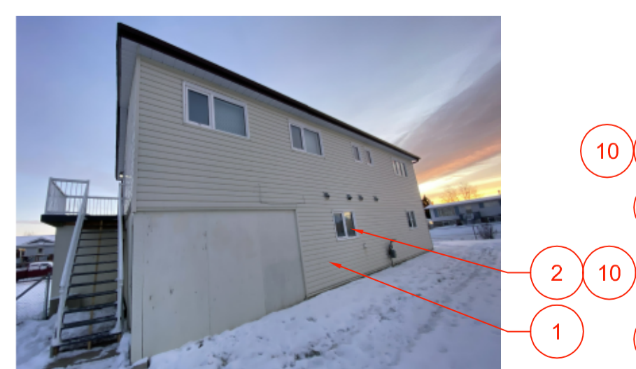
3. BACK VIEW OF ENCLOSED CARPORT AND SERVICE PENETRATIONS
