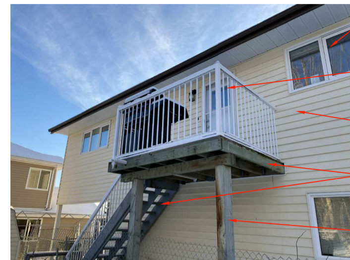
5. VIEW OF DECK
