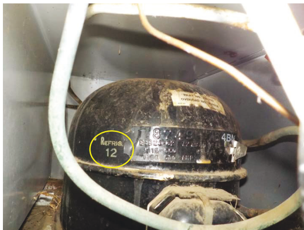
Photograph 19: The compressor of the Viking-branded freezer located in the east room. While the manufacturer's tag could not be accessed, the compressor clearly states that R12 is contained within the unit.
