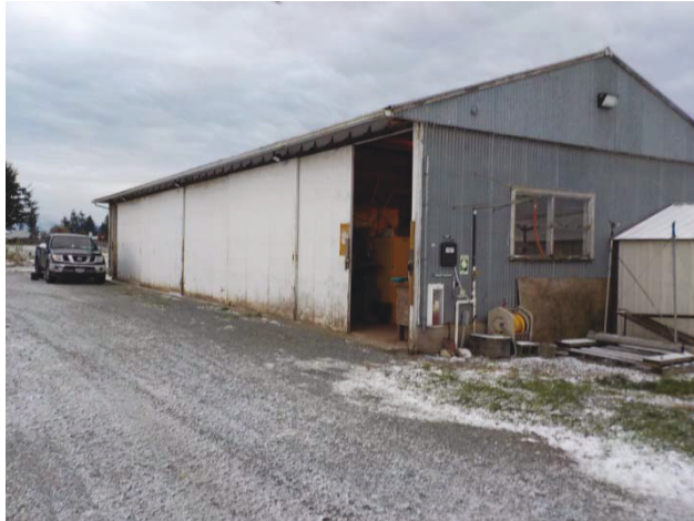
Photograph 1: Exterior of the Building looking southeast. The white paint on the sliding doors was sampled by Stantec and is lead-containing. Note the high-intensity discharge lights over the access doors and on the west side of the Building.
