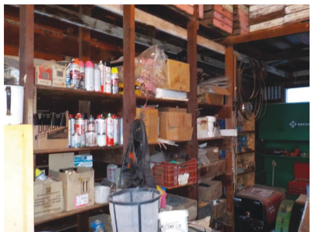
Photograph 12: Paint and paint sundries were identified on the shelving in the west room of the Building. Also note the containers of engine oil stored on the shelves.
