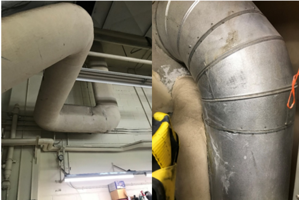
Photo 12 & 13: Aircell pipe insulation and insulated pipe fittings were observed within the cage in room 101A on the DCW line at deck level. The room was inaccessible at the time of the survey.
