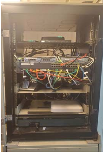
VSAT Gear Bridge Electronic Room
