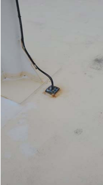
Dome Mid-Ship Cable Penetration
