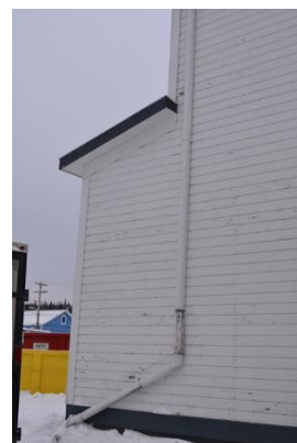
Exterior – Siding and Downspout
