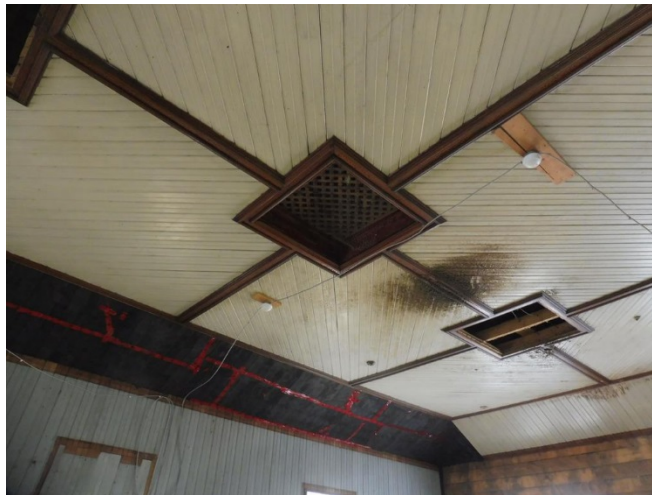
Figure 2 – Typical Courtroom initiating devices and surface mount wiring
