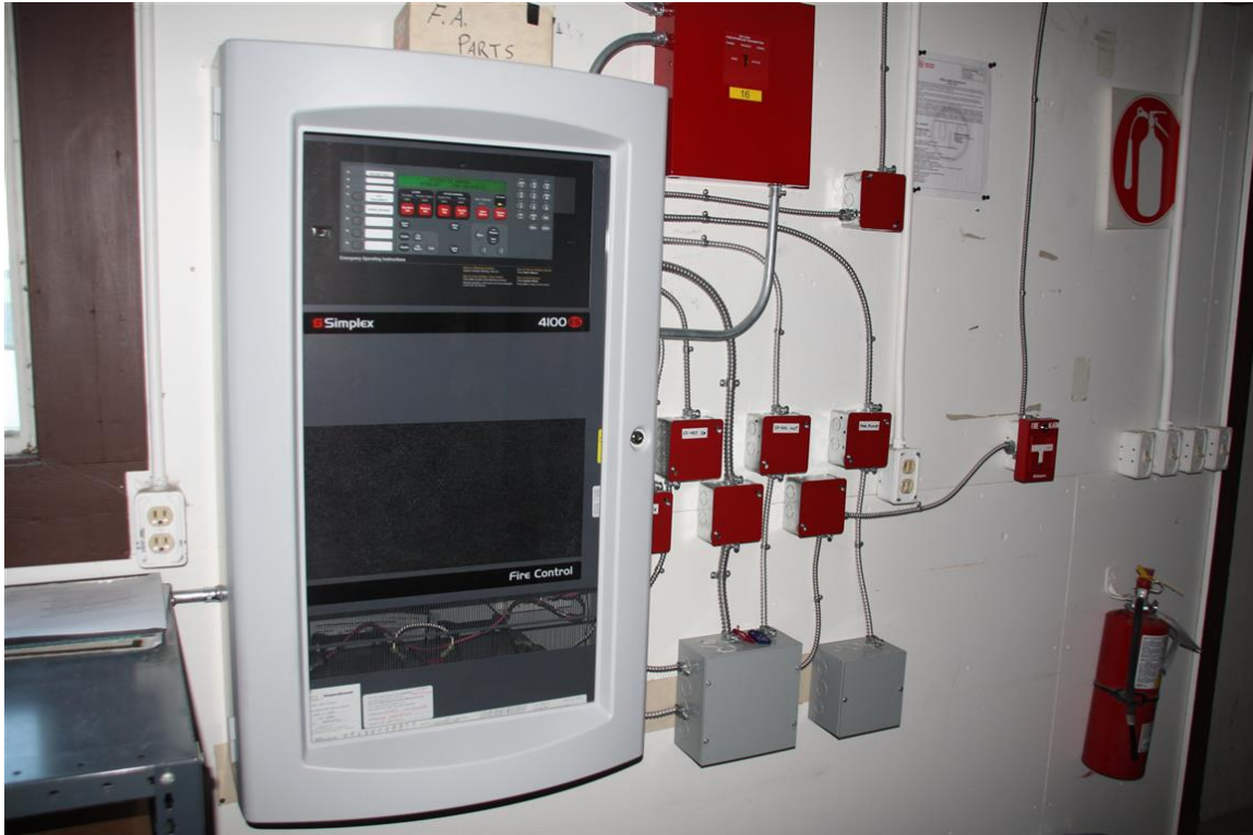
Figure 3 – Main fire alarm panel and alarm communicator located in Carriage Shed
