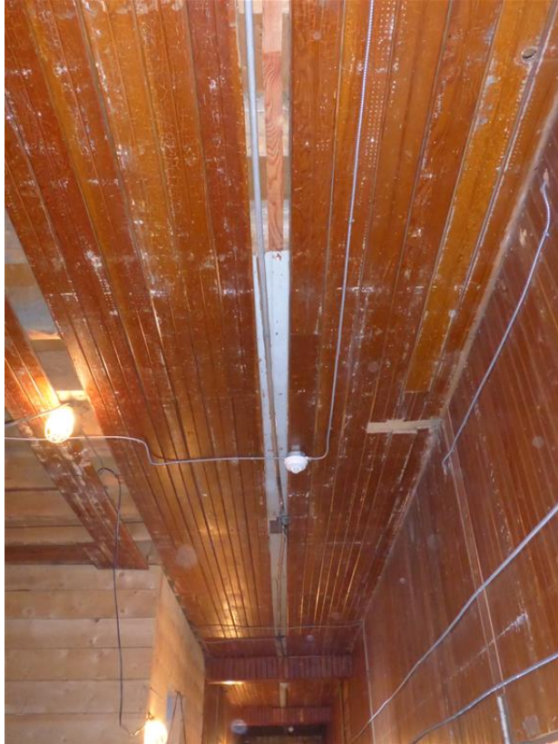
Figure 1 – Typical initiating device and surface mount wiring
