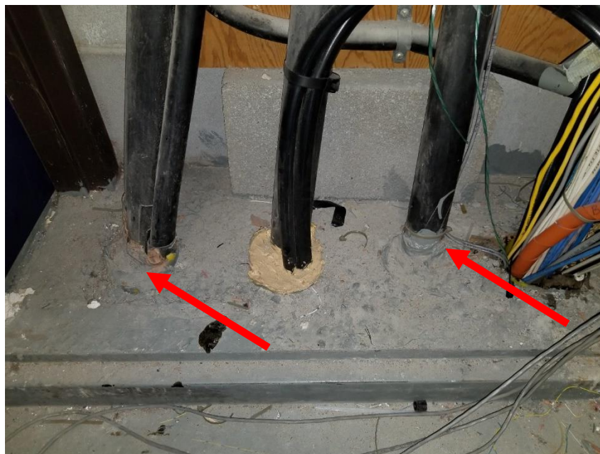
Photo 8: Non-friable cementitious material, intermixed with peach coloured (painted grey), soft caulking, observed in the south-west computer room- conveyor room north end, floor level pipe penetrations was confirmed to contain 1% Chrysotile asbestos (DST Sample ID 34916-32B).
