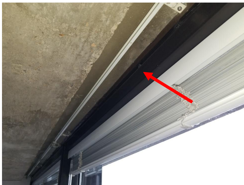
Photo 4: Non-friable, rigid, brown joint caulking, observed at the joint between windows and the concrete bulkhead was confirmed to contain 1% Chrysotile asbestos (DST Sample ID 34916-09A). the material was observed throughout the north, east and south office blocks.
