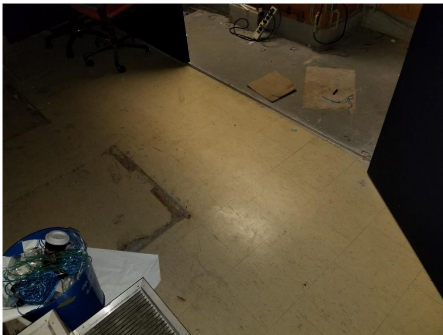
Photo 7: Non-friable 12"X12" vinyl floor tiles, beige with black streaks observed in the south-west computer room- conveyor room was confirmed to contain 3% Chrysotile asbestos (DST Sample IDs 34916-31A-C).
