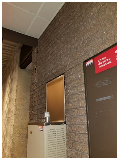
Photo 10: Halocarbons are assumed to be present as a coolant in water fountains observed in the elevator lobby.
