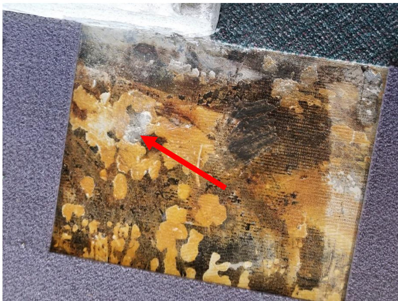
Photo 3: Non-friable floor leveling compound, was confirmed to contain 1% Chrysotile asbestos (DST Sample ID 34916-01B). The material was observed throughout the north, east and south office blocks often concealed under carpeting.
