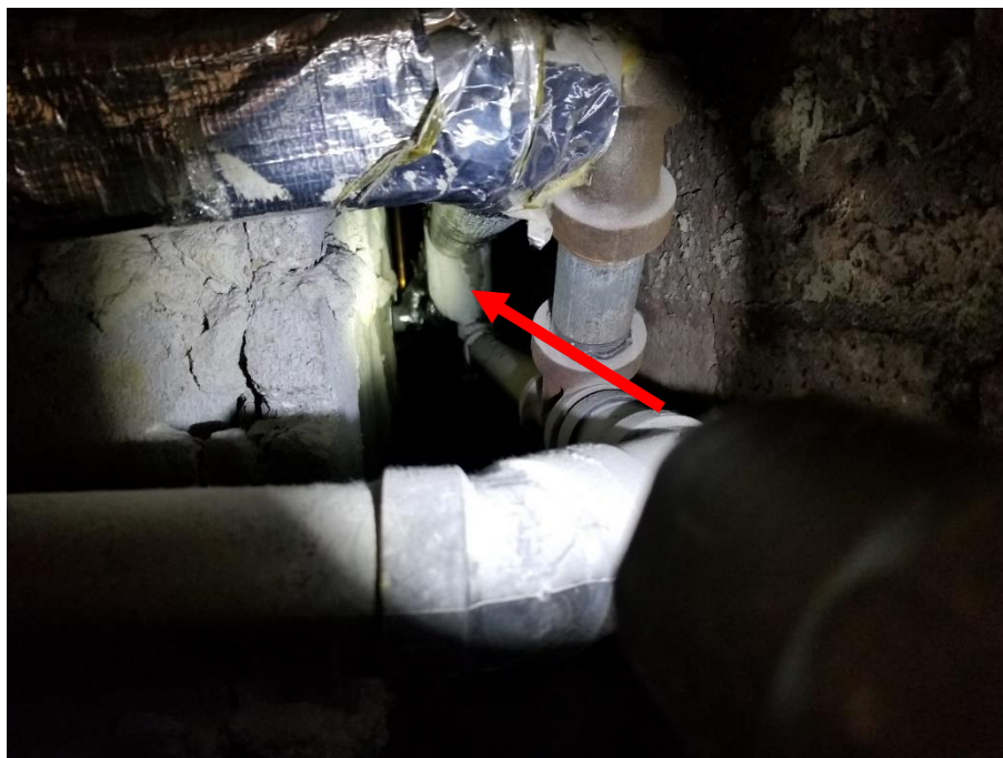
Photo 9: One (1) grey cement compound (GCC) pipe fitting was observed in the pipe chase adjacent the men's washroom in the elevator lobby. The material was inaccessible for bulk sampling, but is assumed to contain asbestos based on appearance.
