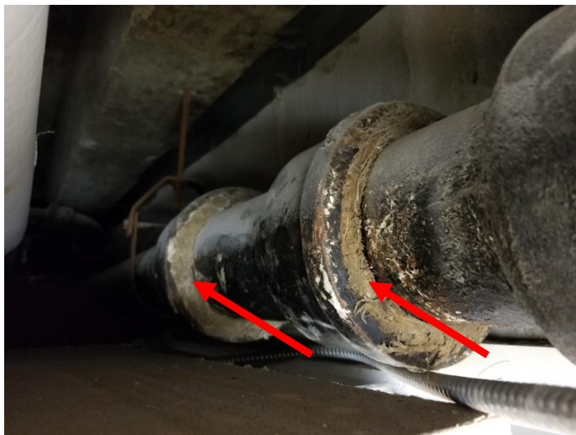
Photo 5: Friable, cast iron joint filler (oakum), observed on a black, cast iron drain pipe above the dropped ceiling in men's washroom in the elevator lobby was confirmed to contain 75% Amosite asbestos (DST Sample ID 34916-25A).
