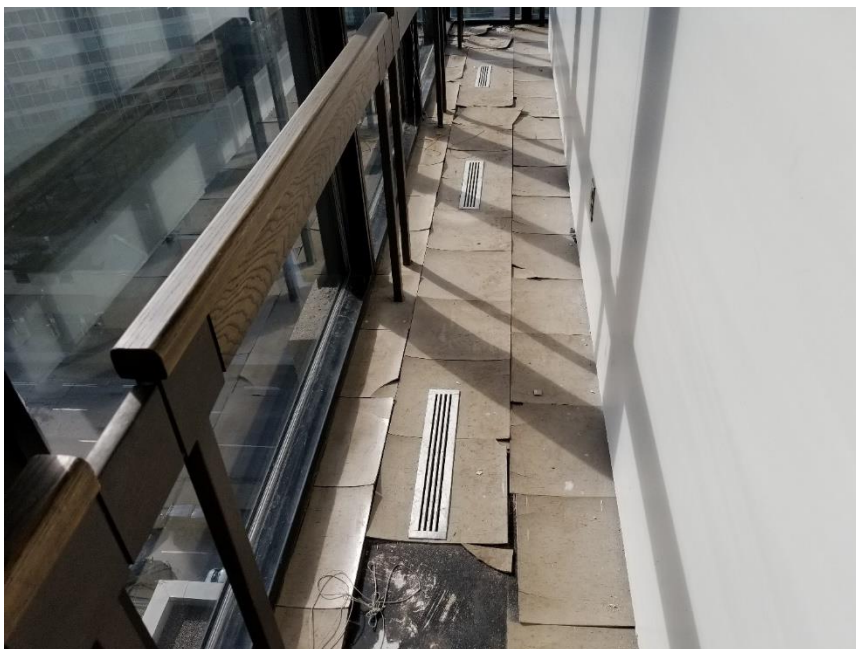
Photo 6: Non-friable 12"X12" vinyl floor tiles, beige with black streaks pictured in the observed in the narrow corridor around the south and north-west computer rooms was confirmed to contain 3% Chrysotile asbestos (DST Sample IDs 34916-31A-C).
