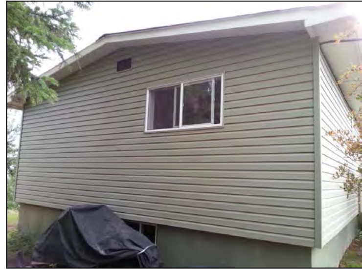
Photo 2: View of the eastern side of the residence.
