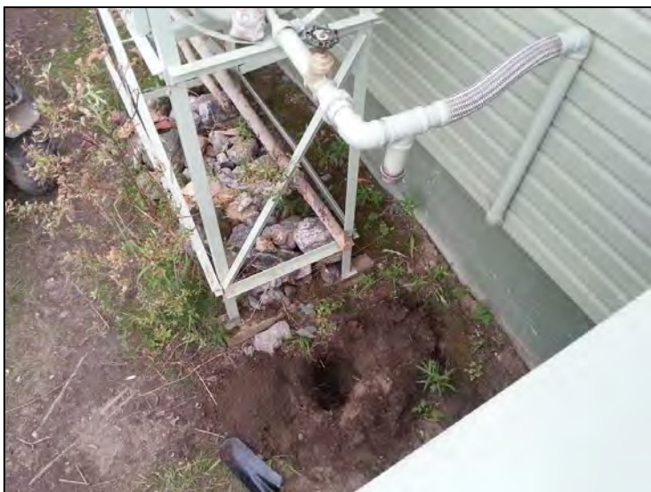
Photo 27: View of the test pit and piping.
