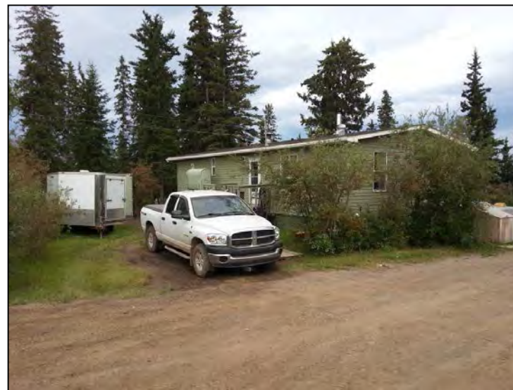
Photo 6: View of the storage trailer and residence.
