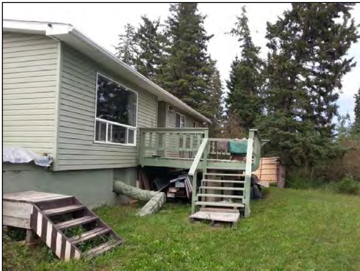
Photo 3: View of the southern side of the residence.
