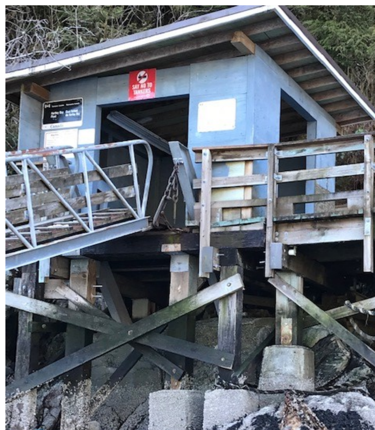
EXISTING WOOD FRAME SHELTER TO BE REMOVED
