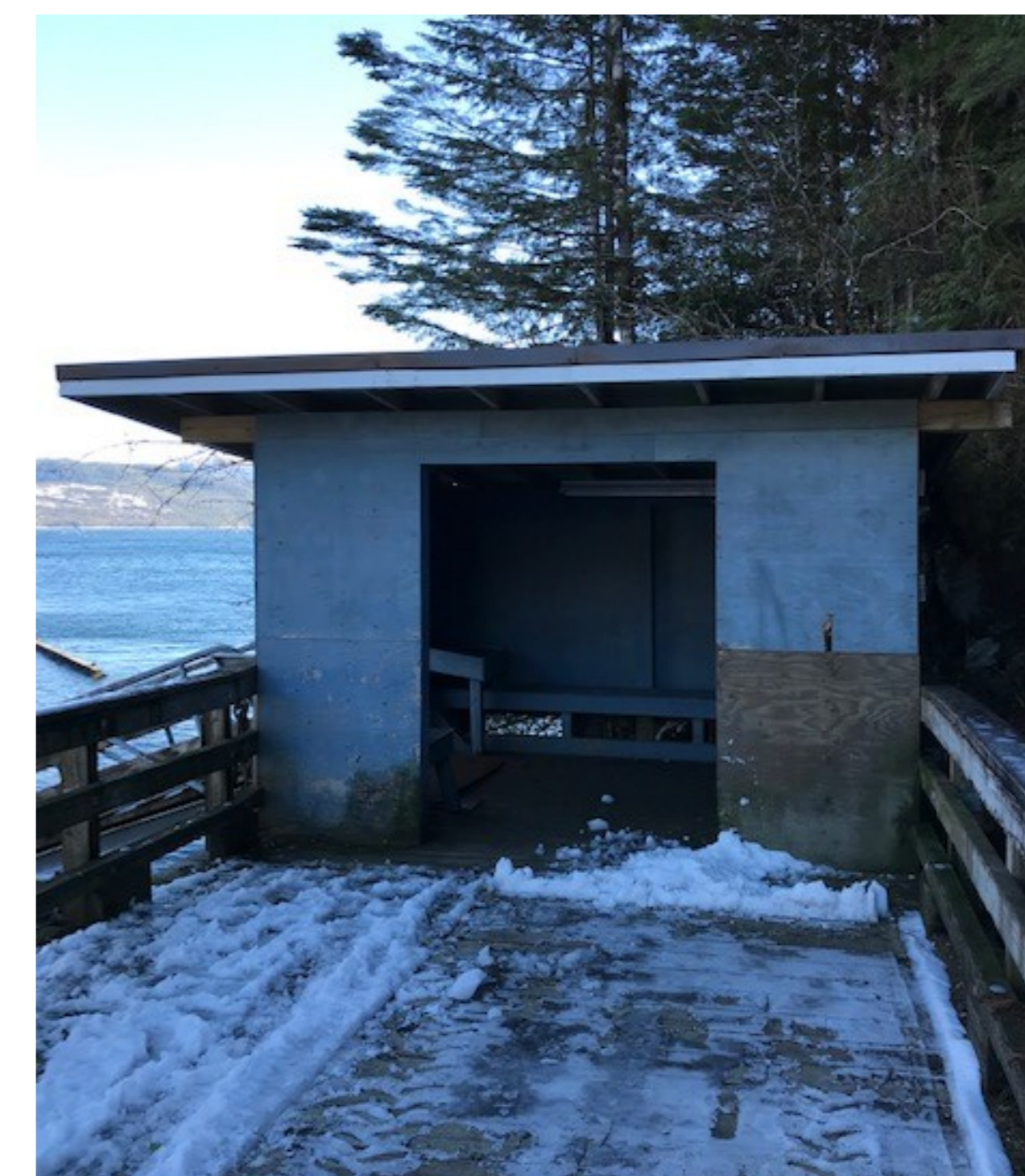
EXISTING WOOD FRAME SHELTER TO BE REMOVED
