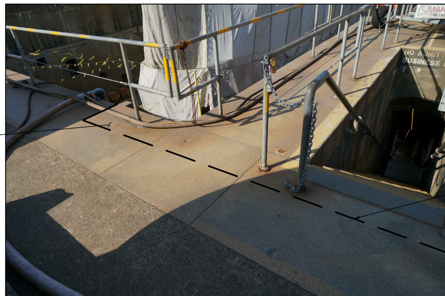
7a. REMOVE GRANITE COPING AT NORTHEAST AND SOUTH EAST CORNERS
