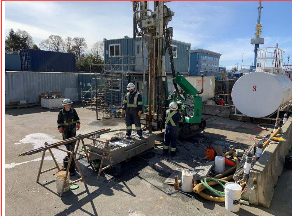
Photo 8: HQ3 drilling of bedrock in progress for BH20-04.
