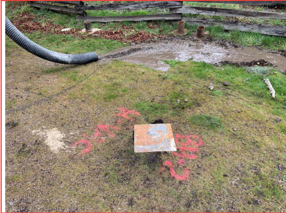
Photo 5: Open hydro-vac holes covered with road plates until backfilling is completed.
