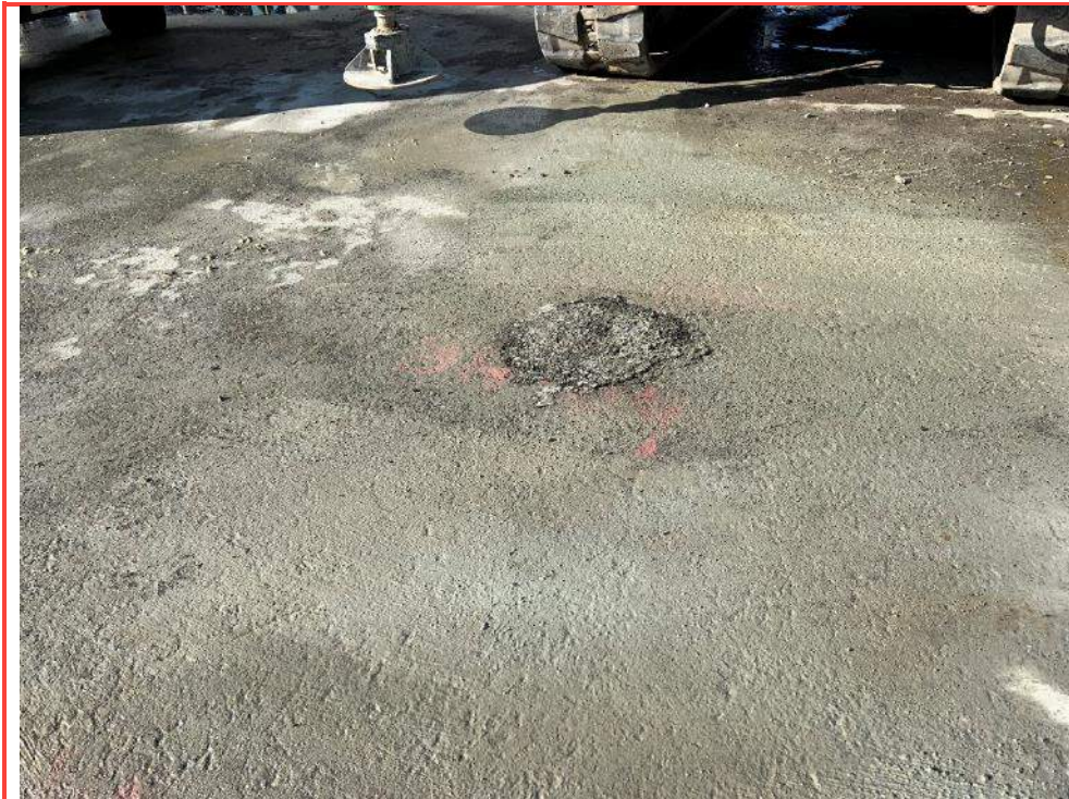
Photo 21: BH20-04 backfilled and asphalt pavement patched.
