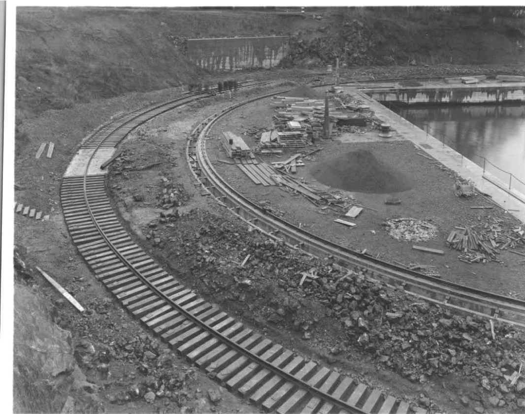
ORIGINAL CRANE RAILS AROUND EAST END APRON (JAN 1927)
