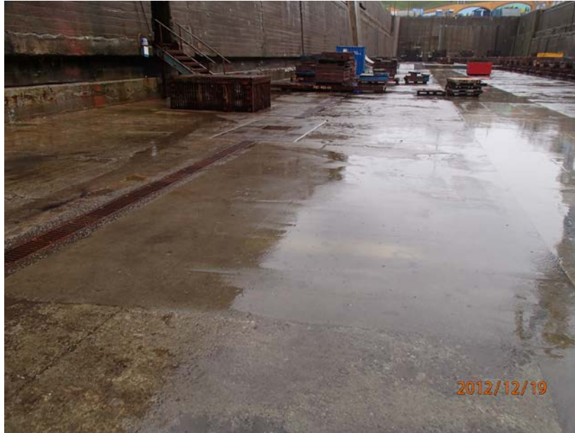
Photo 5: Patch repairs
