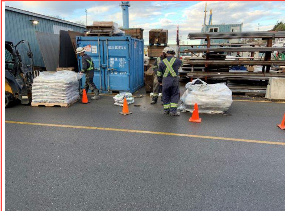
Photo 20: Boreholes typically backfilled with bentonite chips up to underside of pavement.
