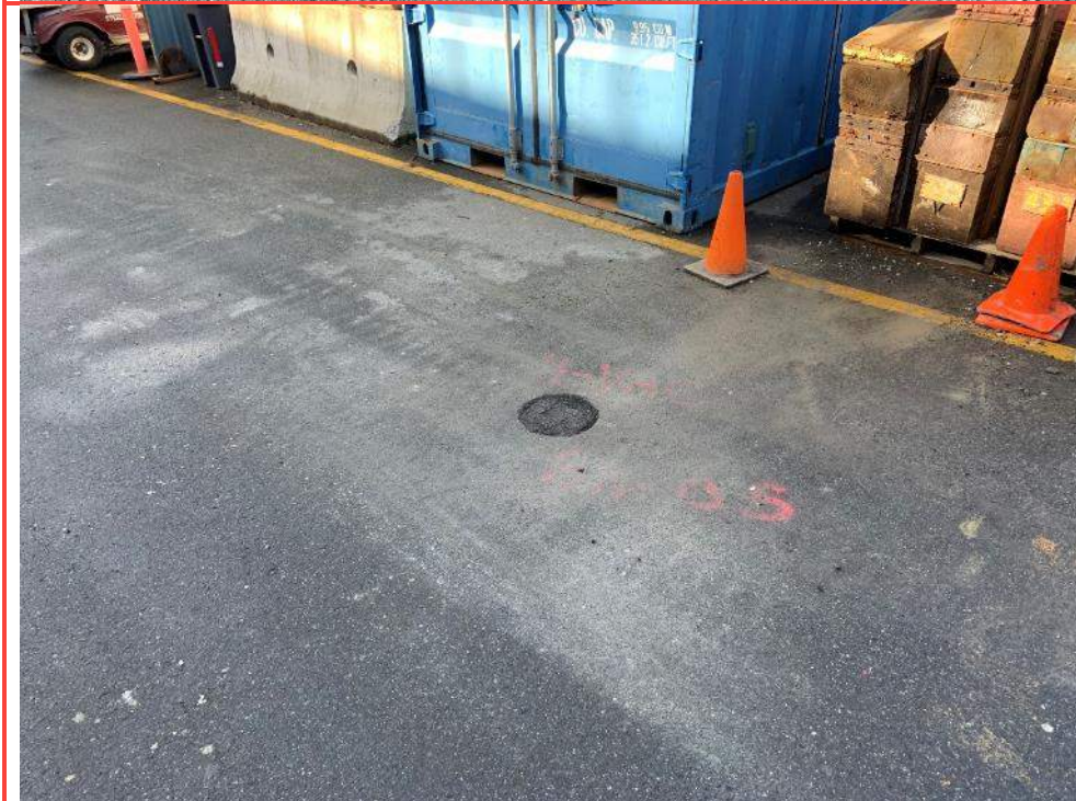
Photo 22: BH20-05 backfilled and asphalt pavement patched.
