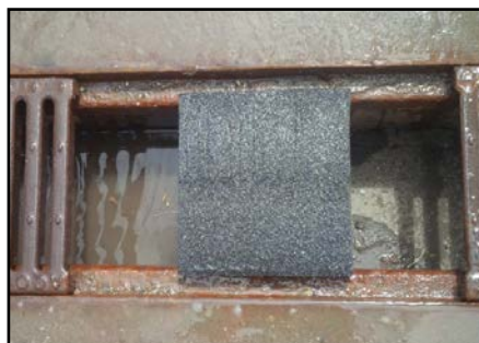
Example of high density styrofoam blocks used as a drain blocker on the NLW.
