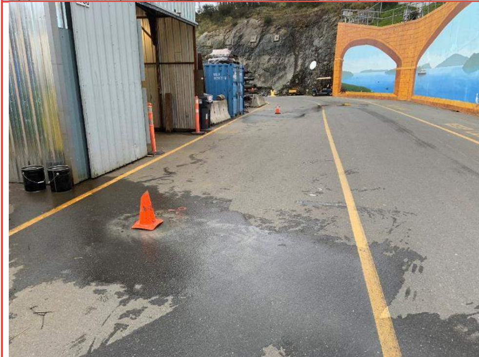
Photo 18: Overview of Enviro Boreholes BH20-05 and BH20-06 locations.
