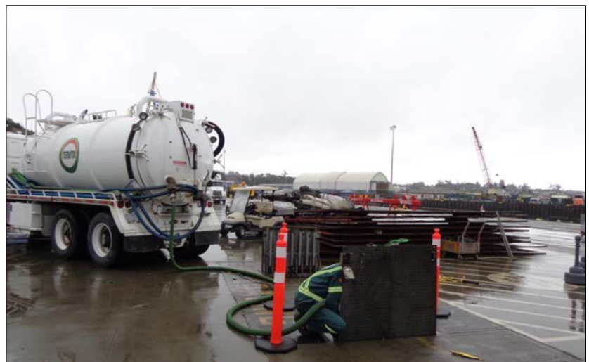
Lift Station Maintenance.
