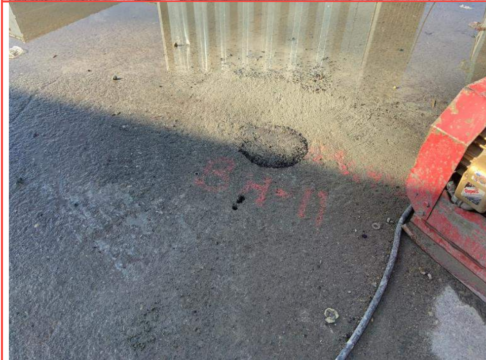
Photo 26: BH20-11 backfilled and asphalt pavement patched.
