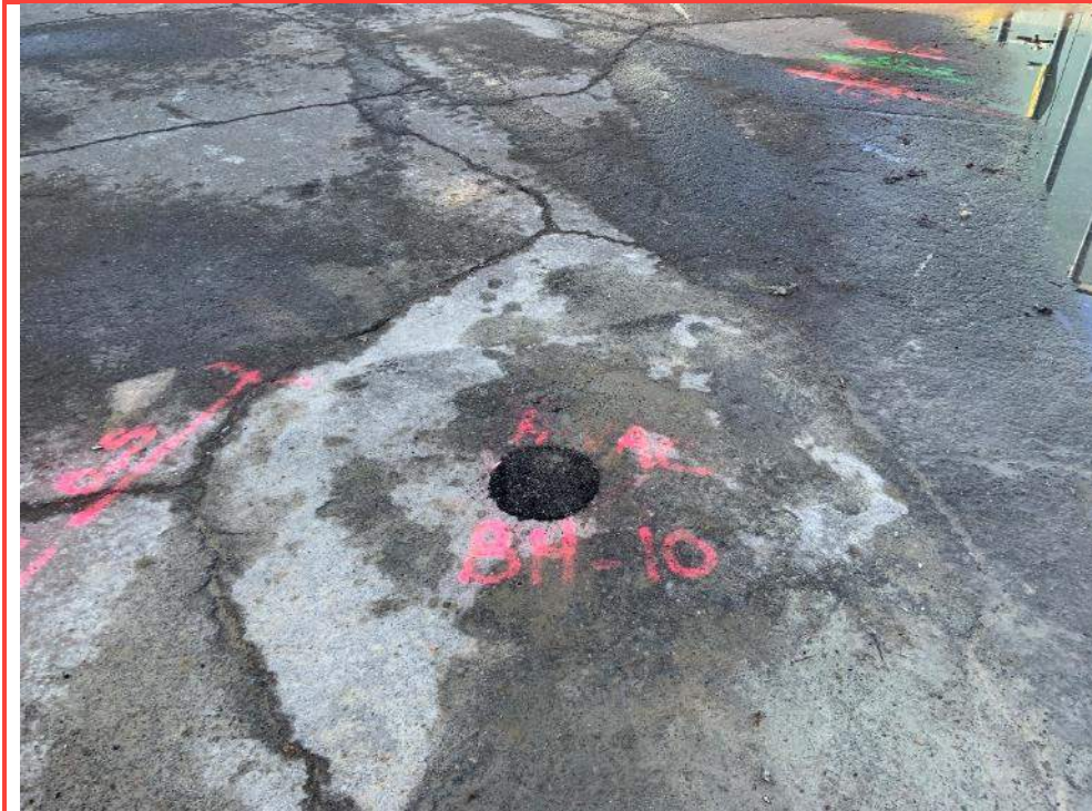
Photo 25: BH20-10 backfilled and asphalt pavement patched.
