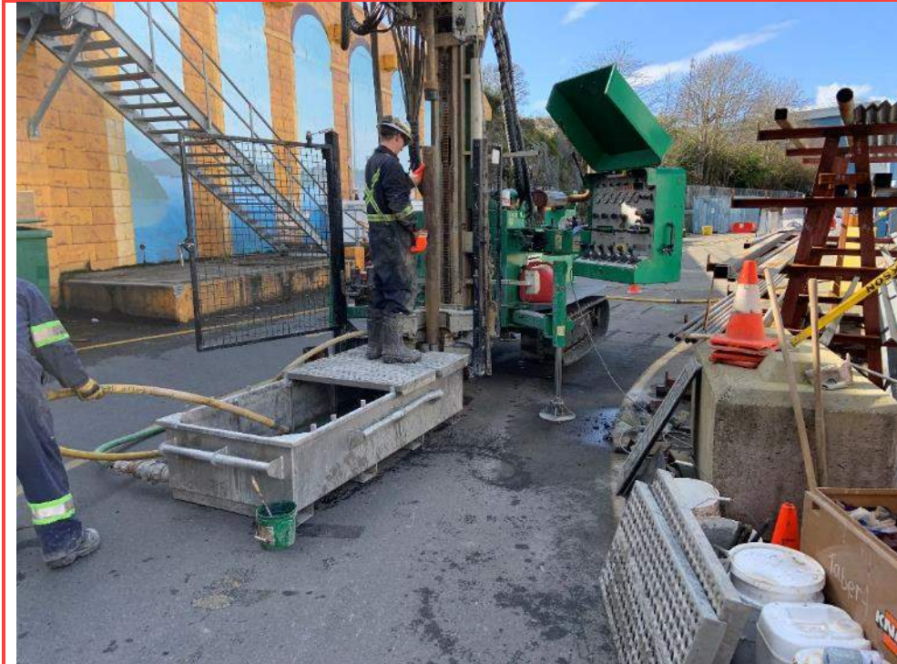
Photo 28: Overview of HQ3 drilling of BH20-07.
