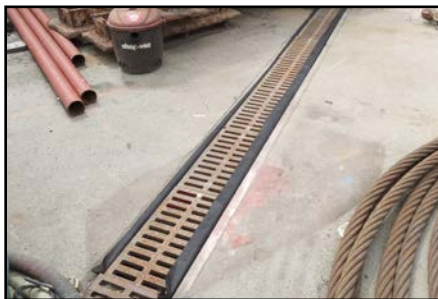
Prevent deleterious substances entering marine environment by placing filter cloth in the trench drains.
