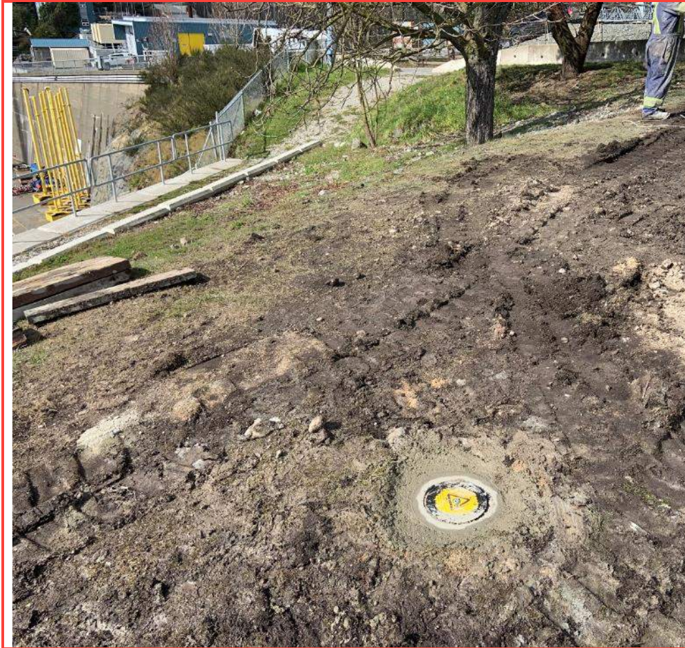
Photo 65: Monitoring well installed within BH20-02.
