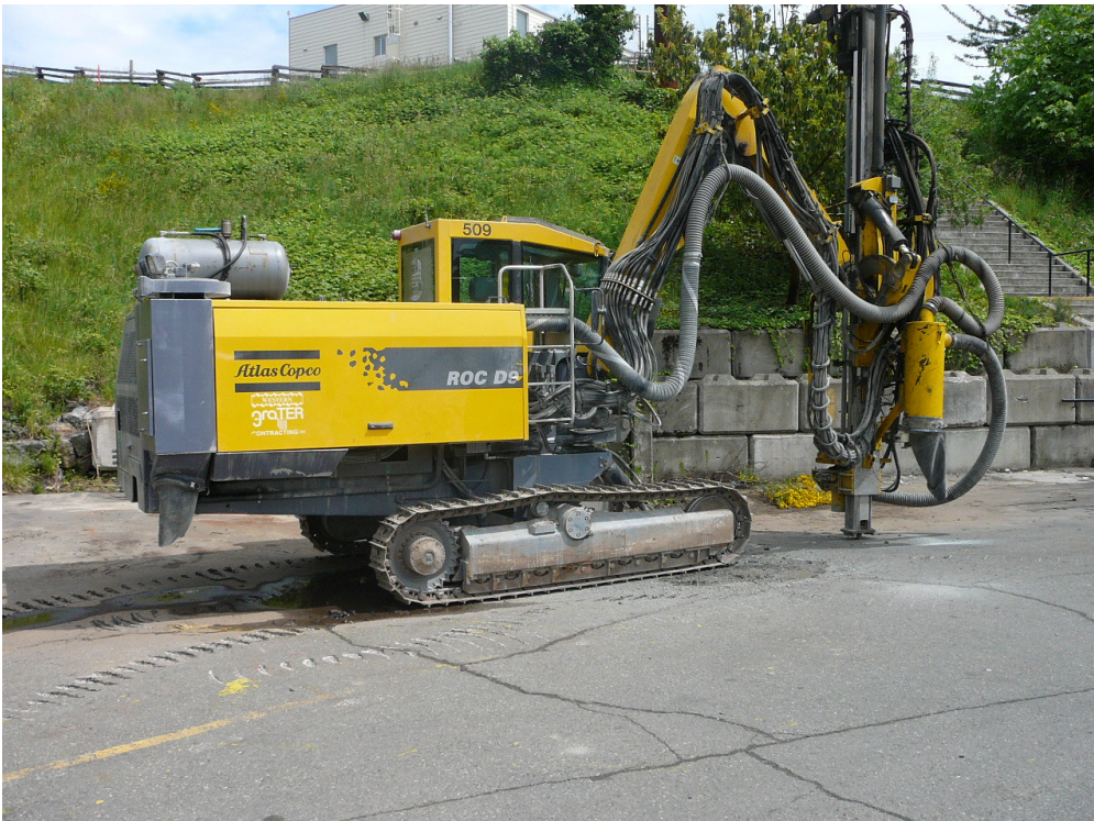
Photo 6: Atlas Copco ROC D9 hydraulic drill
