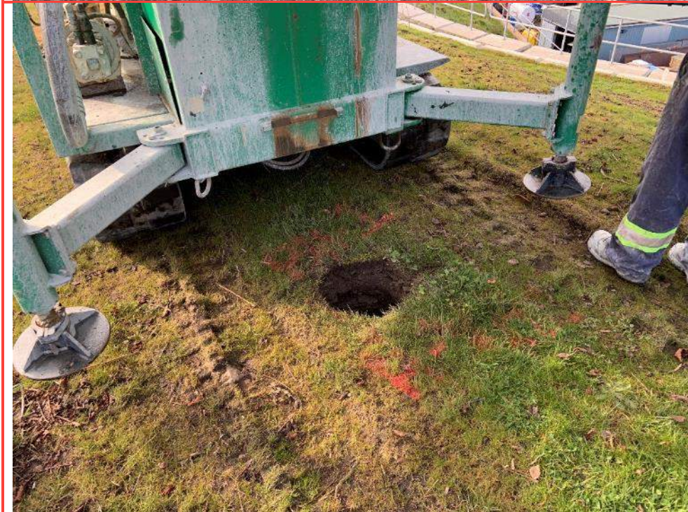
Photo 40: Drill rig set up over BH20-01 after hydro-vac excavation complete.
