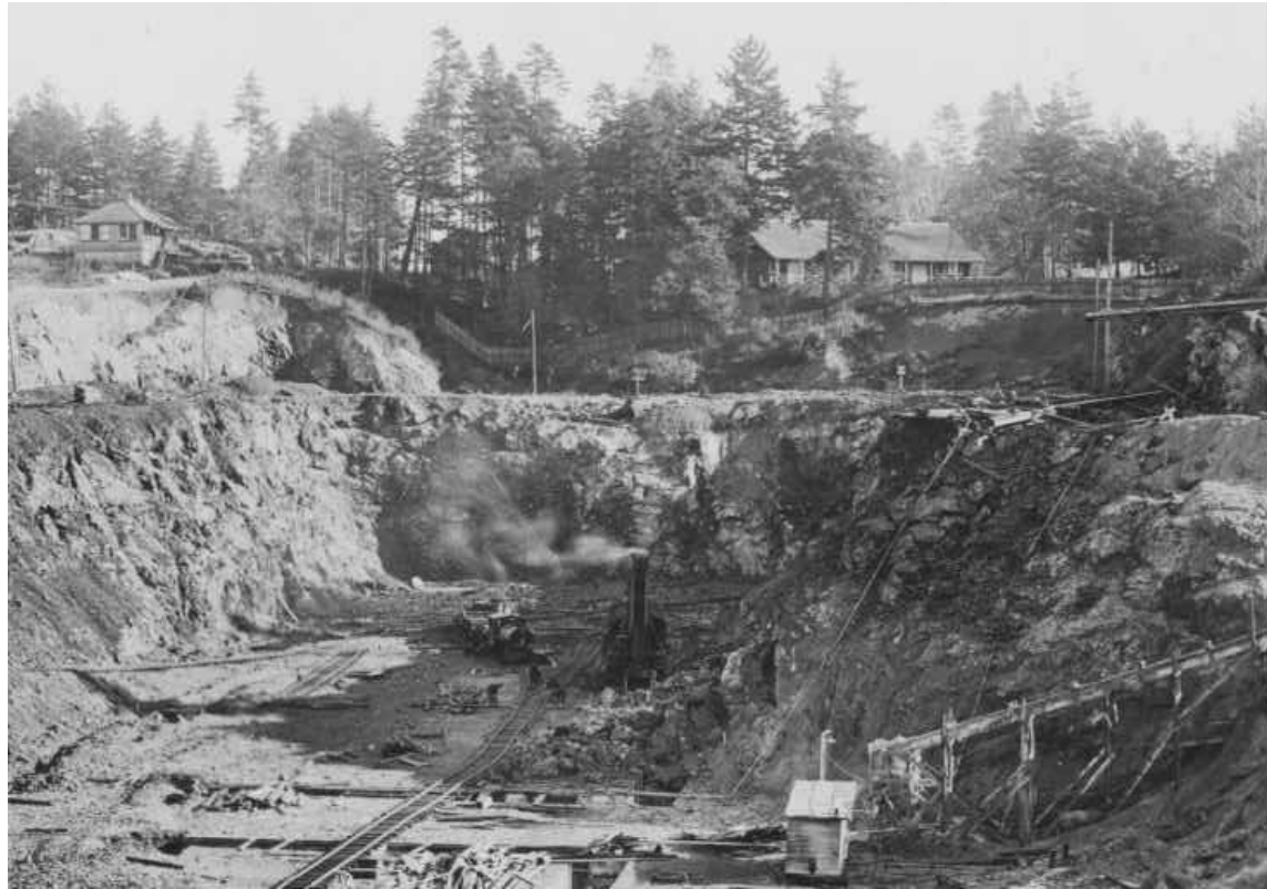
DOCK EXCAVATION AT EAST END WALL, LOOKING EAST (NOV 1922)
