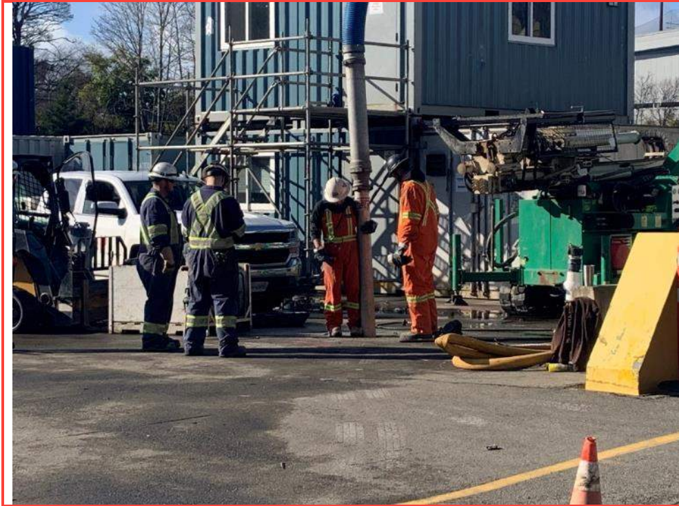
Photo 7: Hydro-vac excavation of BH20-04 in progress.
