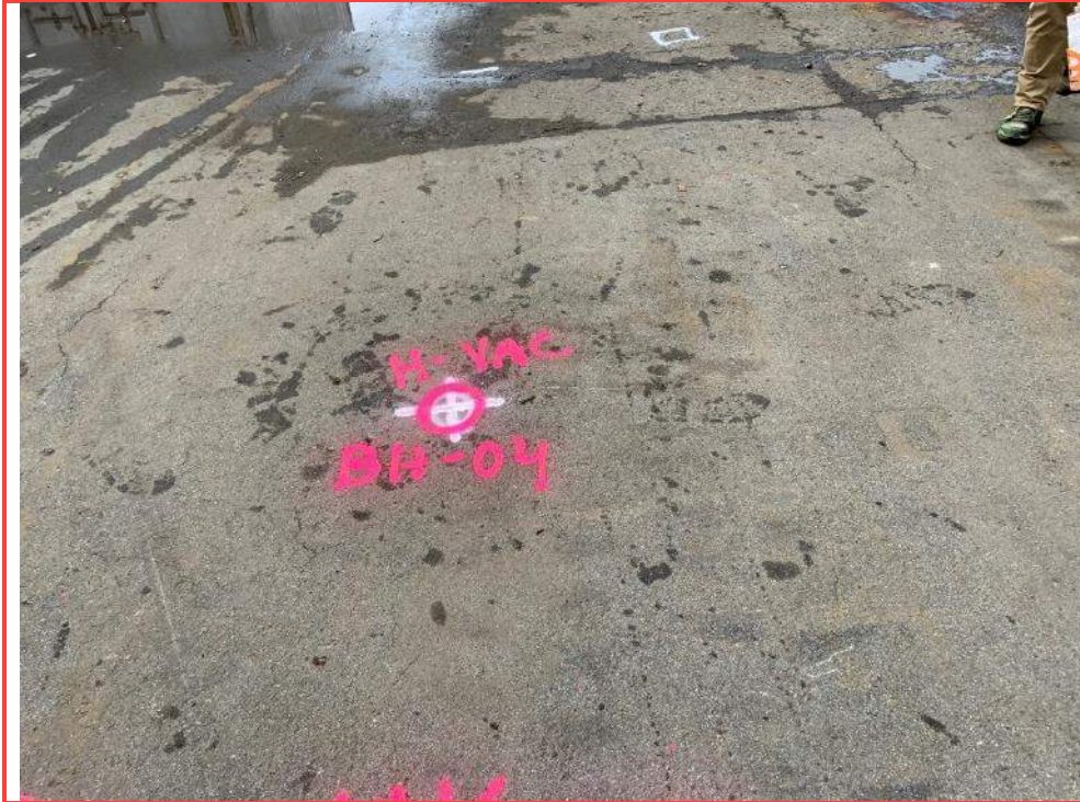
Photo 6: Overview of BH20-04 location prior to coring.
