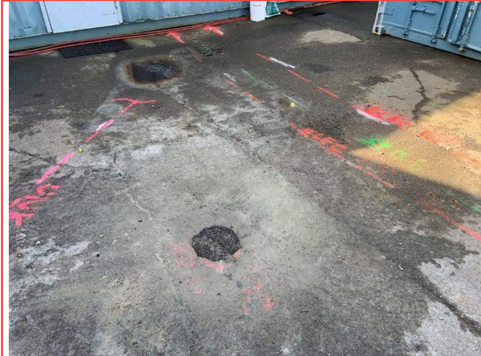
Photo 24: BH20-09 backfilled and asphalt pavement patched.
