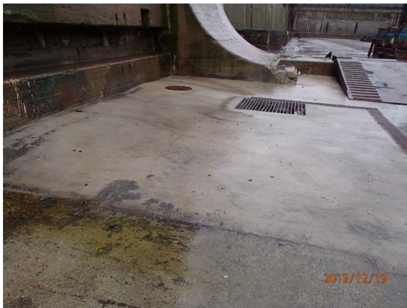
Photo 8: Trial patch sloping towards drains
