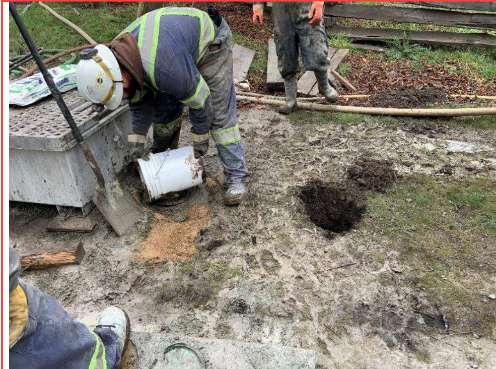
Photo 47: Monitoring well installed in BH20-01. Adjacent BH20-01A excavated approximately 1.2m by hand before drilling.
