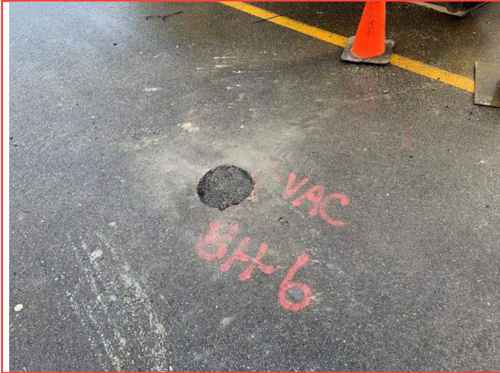
Photo 23: BH20-06 backfilled and asphalt pavement patched.
