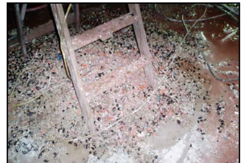
INADEQUATE containment: Biological growth mixed with paint waste on drydock floor.
