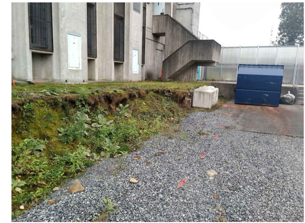
SITE PHOTO #3 ROCK WALL, STAIRS, DRIVEWAY LOOKING WEST
