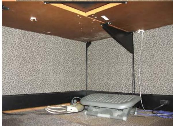
Configuration #3 - workstations that require some minor modifications to the work surfaces. Centre work surfaces need to have a metal plate added in order to fill in the keyboard cut-out that is currently there. Corner metal plates must be wider than the opening. All work surfaces need to be fused together to create a one-piece height adjustable work surface.
