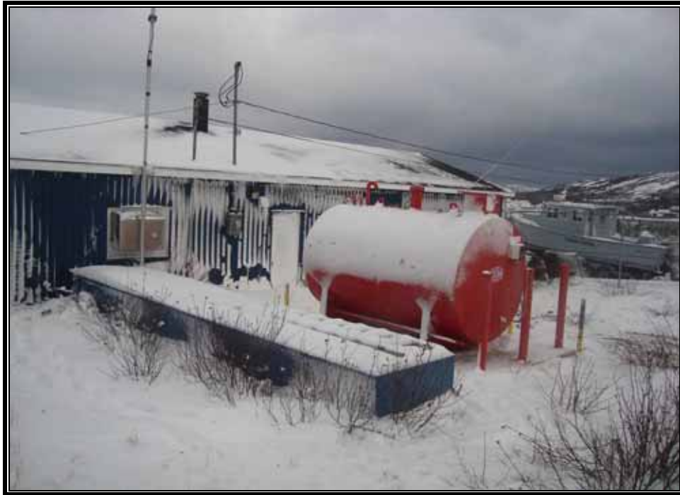
Photo 3: Southern view of the new self-dyked 9,092 L AST and of the artesian well located south of the building.
