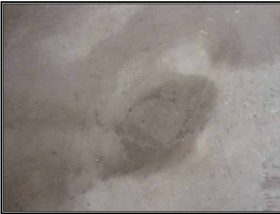
Photo 10: Concrete patch on LEWI-58590-09-TH01 performed after soil sampling.
