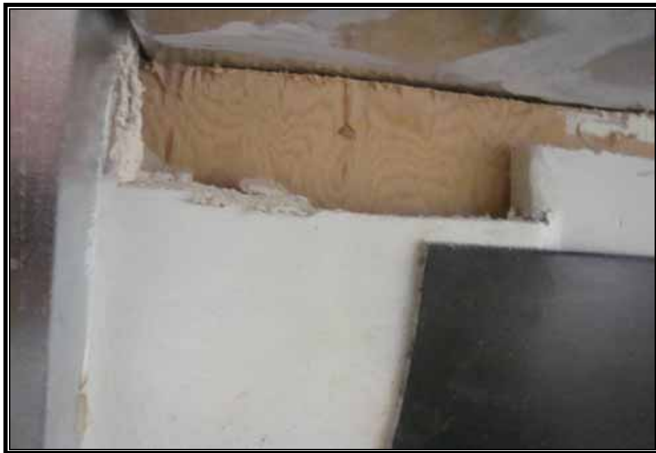
Photo 16: Mineral board sheeting sampled for asbestos content, inside the furnace room.
