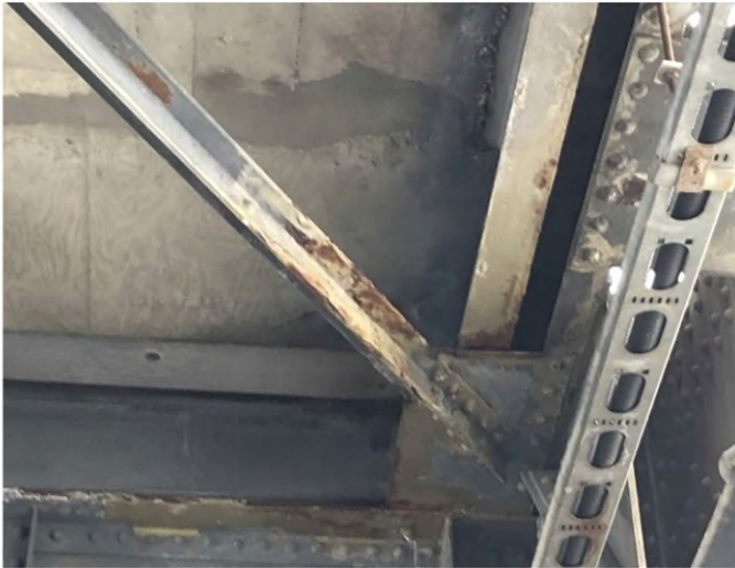
Example of Steel Member requiring repair
