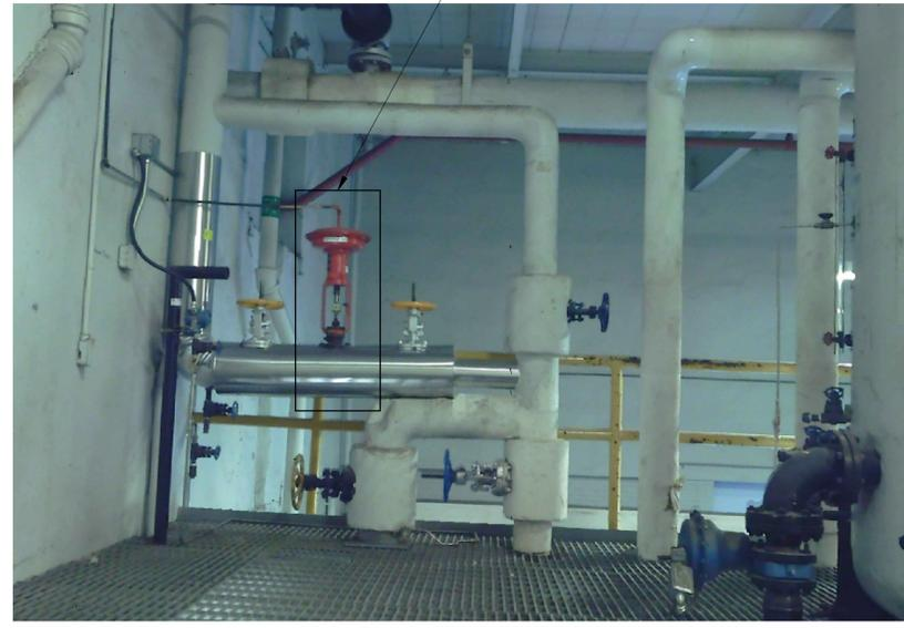
PHOTO 6: WATER LEVEL CONTROL VALVE (5889-M08)
