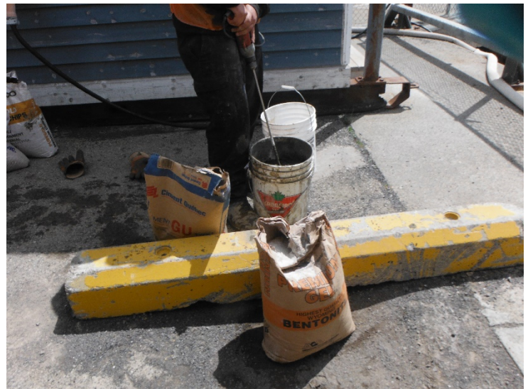
PHOTO 54 Creation of a bentonite cement plug
