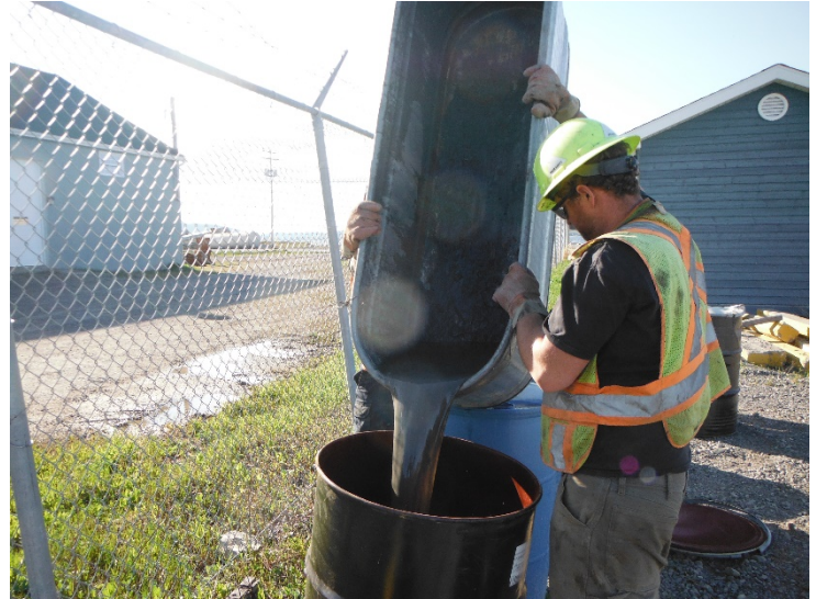
PHOTO 52 Recovery of auger wash water
