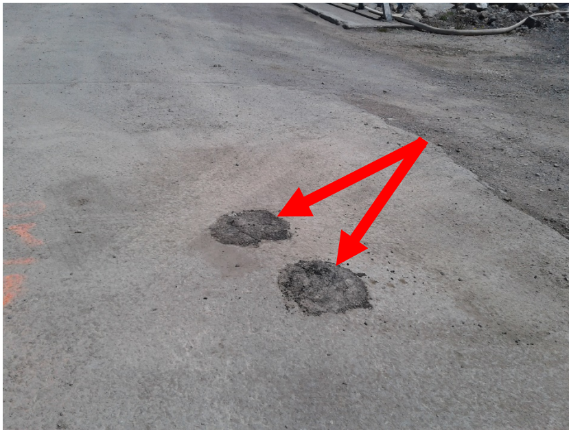
PHOTO 15 Rehabilitation of the surface of sampling well 2019-PE13 The borehole was moved because an object was detected by Mine/EOD
