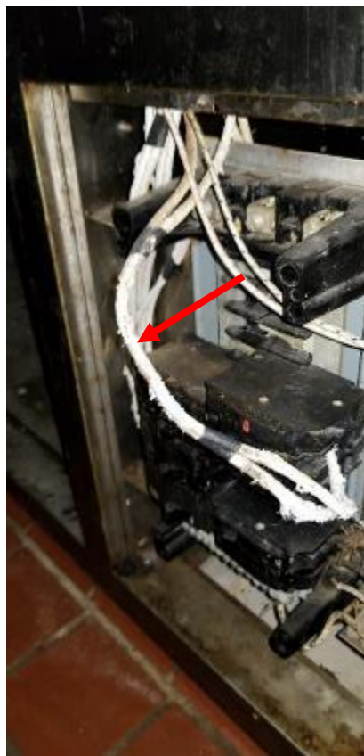
Photo 22: Friable, white fibrous electrical wire sheathing, observed in the first floor kitchen area contains 65% Chrysotile asbestos.
