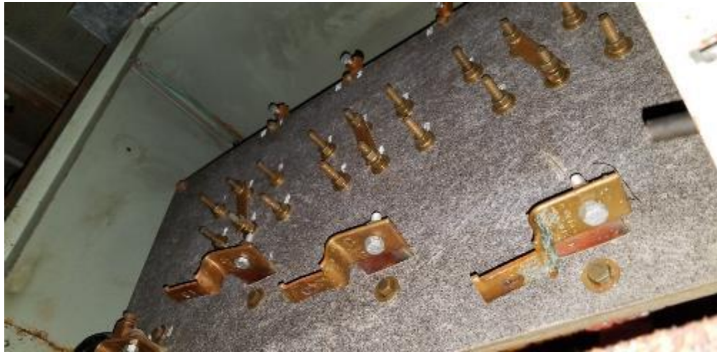
Photo 23: Suspect asbestos-containing transite panel observed in the basement west electrical room.
