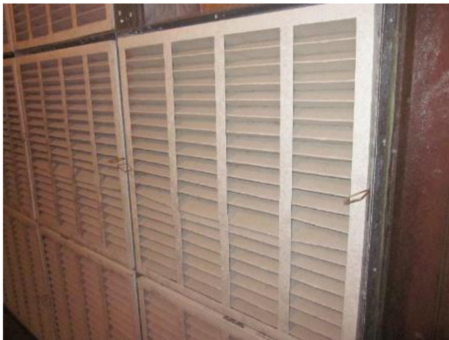
Photo 24: Suspected mould impacted air filters observed in sub-basement mechanical room.
