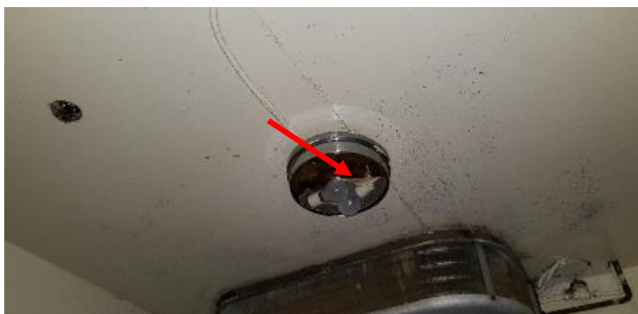
Photo 10: Light heat shield was observed in the south-west walk-in freezer on the first floor, kitchen area contains 75% Chrysotile asbestos.
