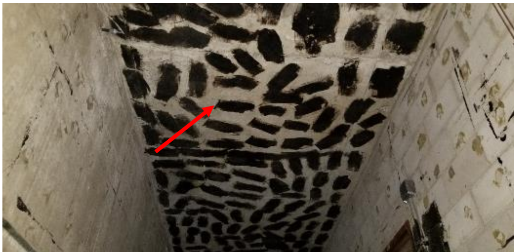
Photo 16: Black wall/ceiling mastic contains 11.67% Chrysotile asbestos
