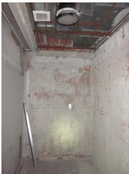
Photo 12: Remnant wall texture coat materials were confirmed to contain 1% Tremolite asbestos, in storage rooms adjacent to former first floor conference room. Based on visual observations, this areas appears to have already been selectively abated/chipped.
