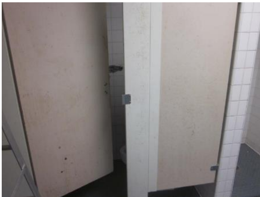
Photo 26: Suspected mould impacted washroom stalls in basement washroom areas (most surfaces visually impacted by mould growth).
