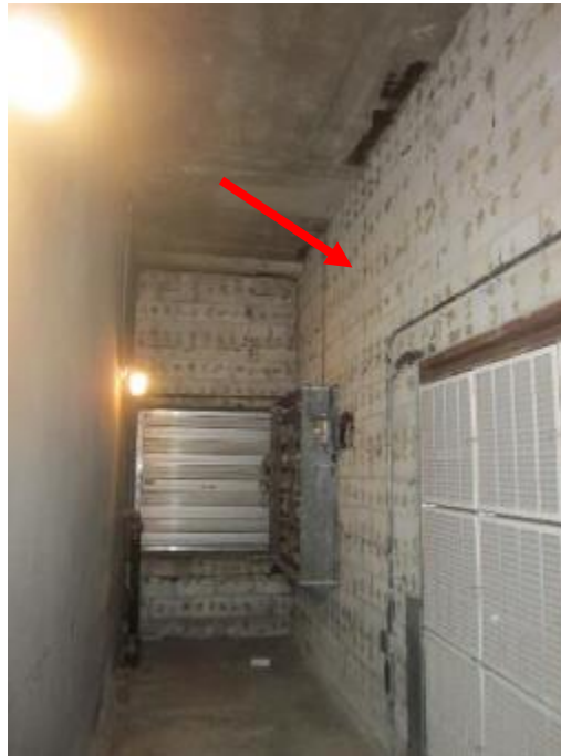
Photo 13: Adhesive pucks present throughout sub-basement and basement air plenums and rooms adjacent to plenums contains 0.5% Chrysotile asbestos.
