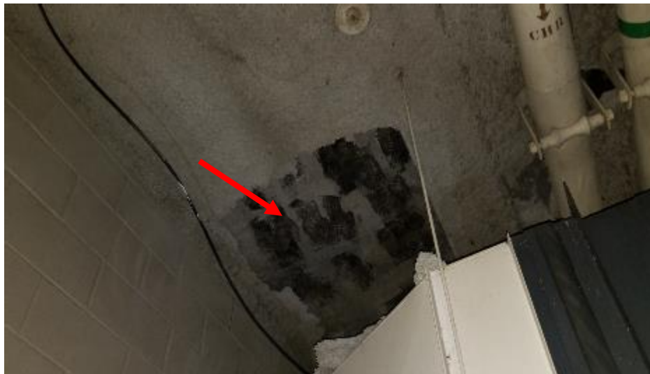
Photo 7: Tar layer beneath spray fireproofing in basement mechanical room contains 20.43-31.06% Amosite and 3.4-7.77% Chrysotile asbestos.
