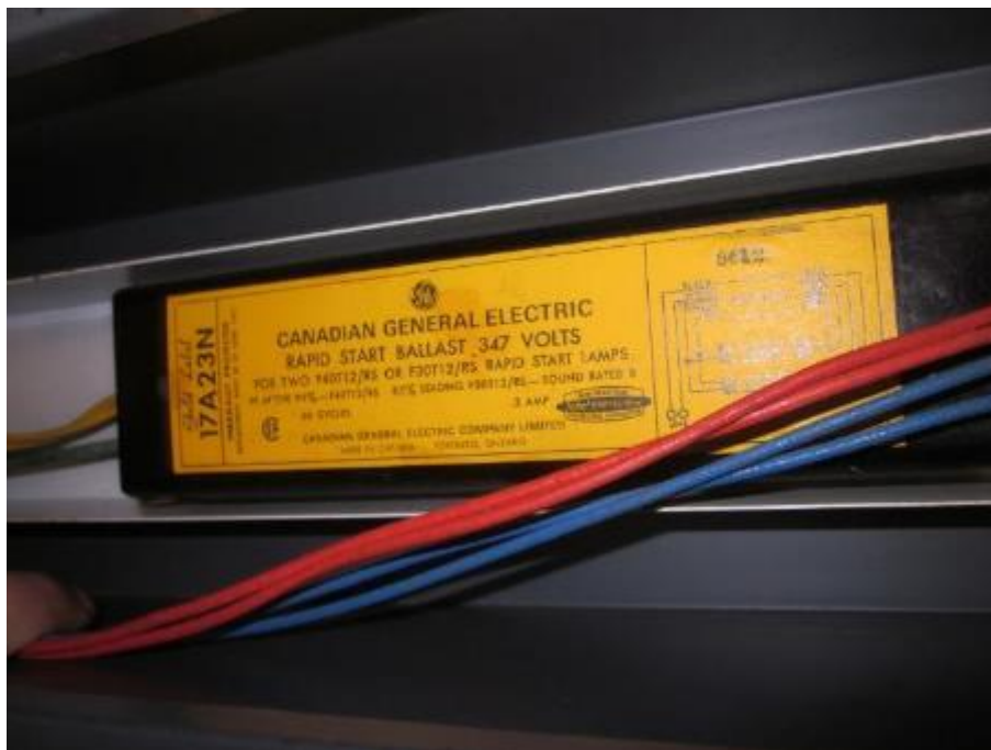
Photo 27: Based on limited visual observations, select exposed PCB-containing ballasts were identified in the building. All ballasts throughout the building should be assumed to contain PCBs, unless proven otherwise by additional investigation.
