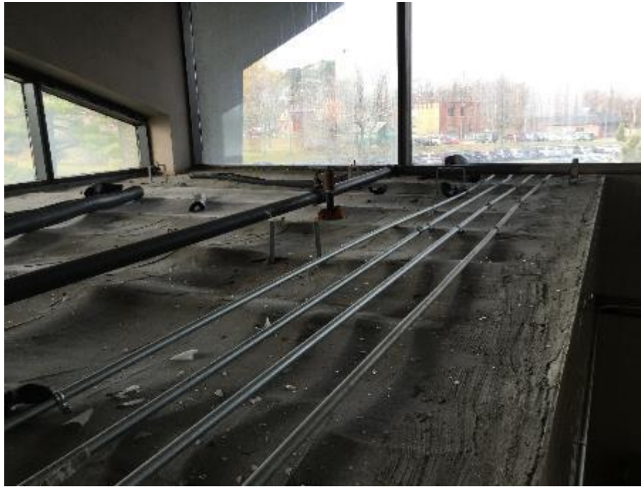
Photo 15: The cementitious layer on top of kitchen ceilings (such as walk-in fridges) has been confirmed to contain asbestos.
