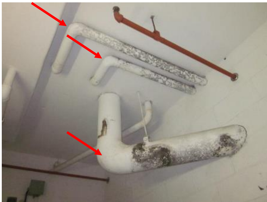
Photo 5: Grey cement compound pipe fitting insulation contains 25-50% Chrysotile asbestos and mould impacted pipe insulation canvas, sub-basement stairwell. Layered cardboard wrap pipe insulation was confirmed to not contain regulated concentrations of asbestos.
