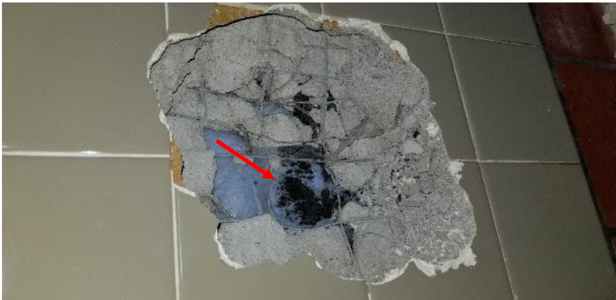
Photo 20: Black tar, applied to blue foam insulation contains 7% Chrysotile asbestos. The tar is concealed behind ceramic tiles and grey plaster on first floor kitchen walls.
