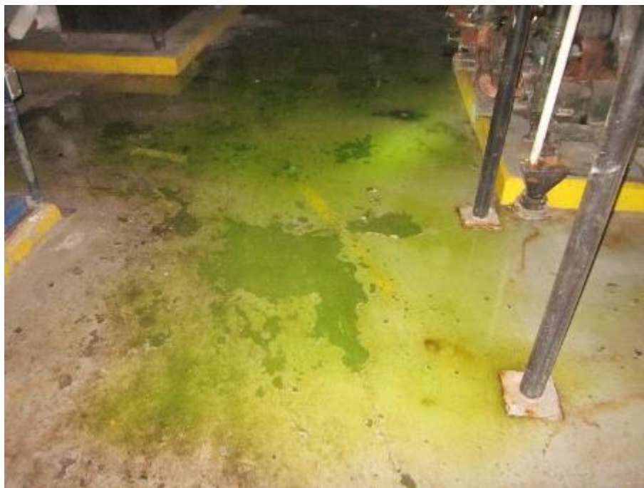
Photo 25: Suspected glycol and/or coolant leak was historically observed throughout the concrete floor of the sub-basement mechanical room (not accessible 2019 due to flooding).
