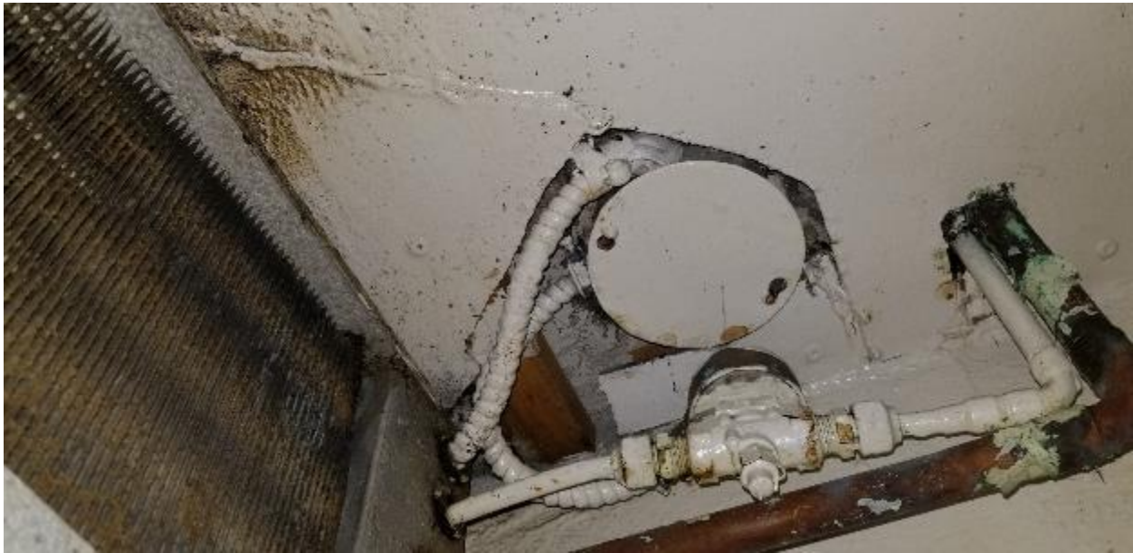
Photo 19: Transite ceiling panels in the south-west walk-in freezer on the first floor, kitchen area contains 9% Chrysotile asbestos.
