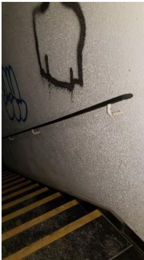
Photo 1: Textured wall coat and ceiling materials throughout select areas of the building, contains 1-2% Chrysotile asbestos (stairwell from first floor to basement pictured above)
