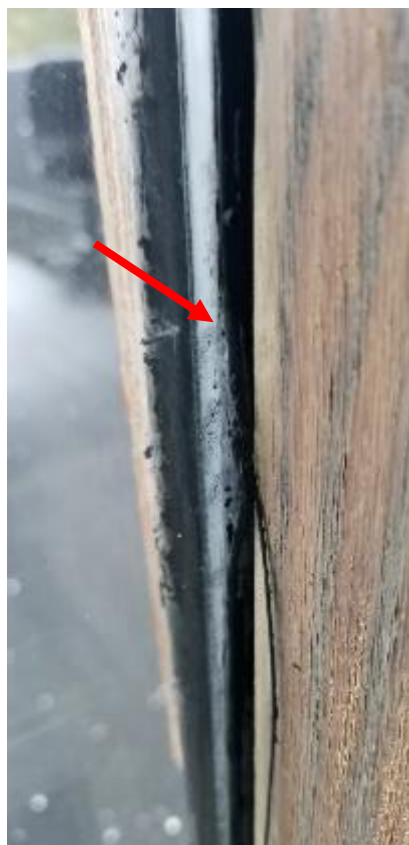
Photo 18: Black window caulking contains 4% Chrysotile asbestos and was observed on windows throughout the building.
