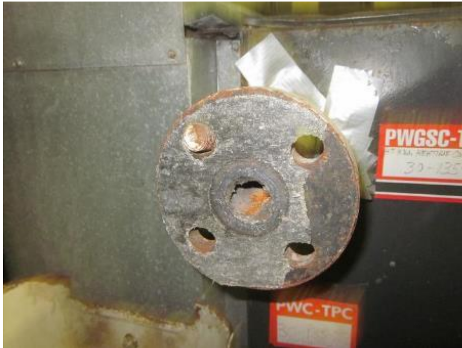
Photo 3: Pipe gaskets throughout the building contain 50% Chrysotile asbestos.
