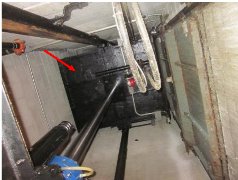
Photo 9: Black tar applied to bottom of elevator cab has been confirmed to contain 5.77% Chrysotile asbestos.
