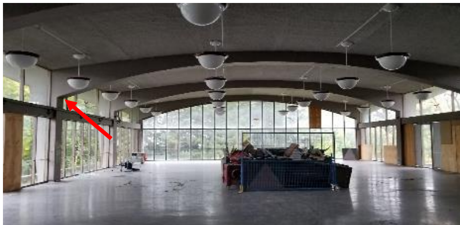
Photo 8: Plaster columns and ceiling bulkheads throughout the first floor kitchen and cafeteria area contain 1% Tremolite asbestos.
