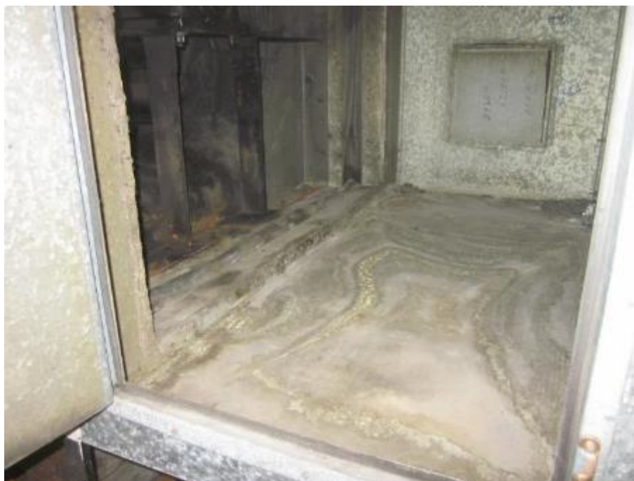
Photo 28: Interior of ventilation ductwork (basement mechanical room shown above) was observed to be impacted by suspected mould.
