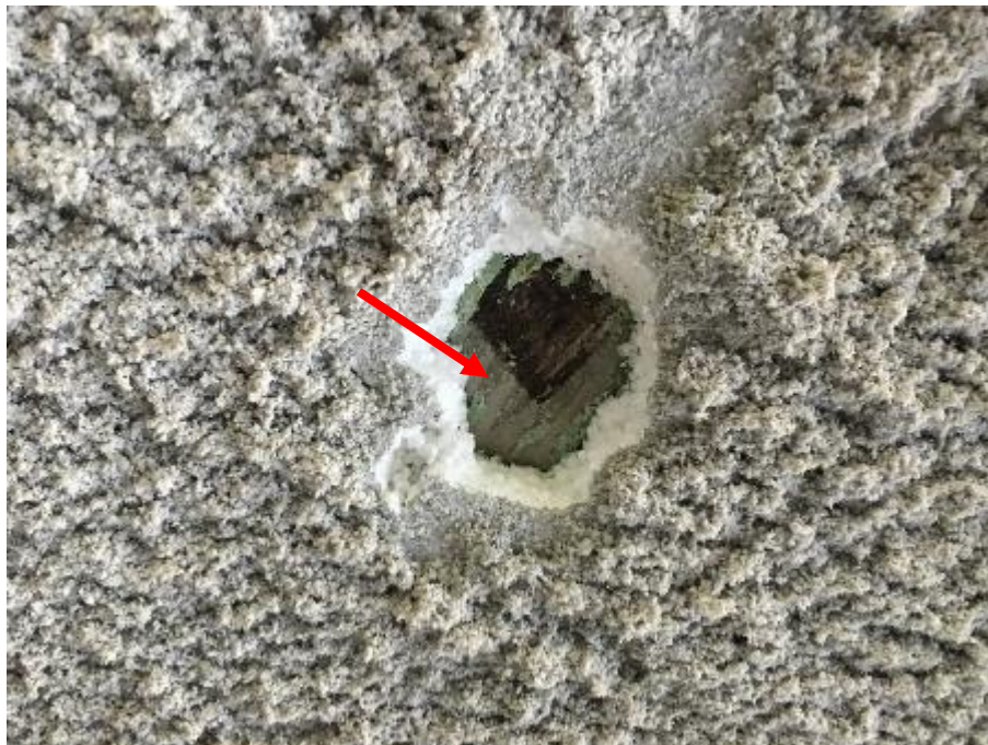
Photo 14: Green mastic and black tar beneath Styrofoam insulation, which is present beneath fireproofing materials, and drywall materials on the ceiling arches in the kitchen and cafeteria have both been confirmed to contain asbestos.
