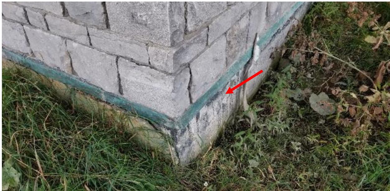
Photo 21: Non-friable exterior foundation tar contains 2% Chrysotile asbestos
