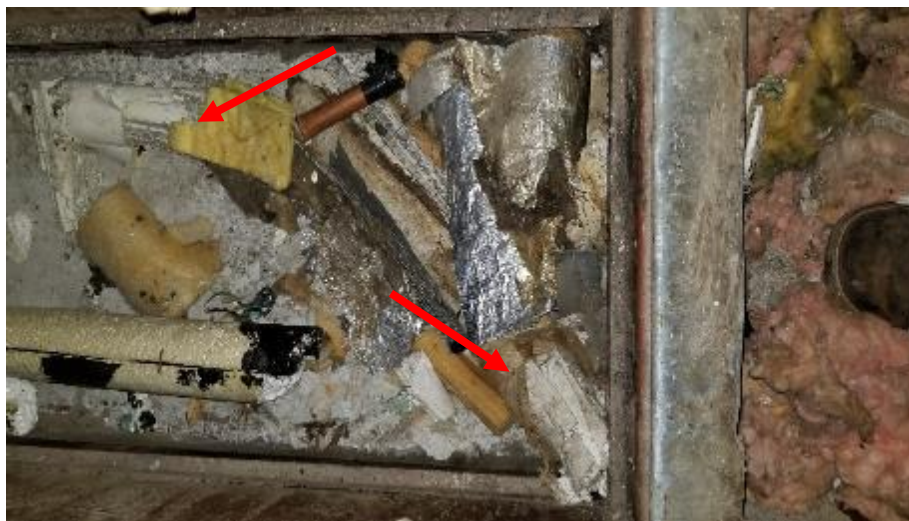
Photo 6: Aircell pipe insulation contains 5-25% Chrysotile asbestos. Aircell debris, pictured in the first floor kitchen pipe shaft.
