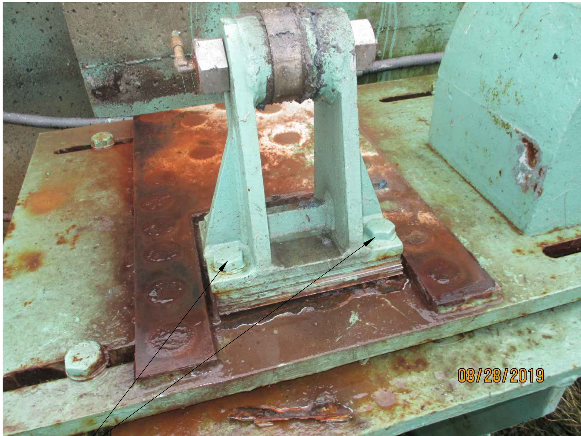
DAMAGED SPAN LOCK RECEIVER MOUNTING BOLTS
